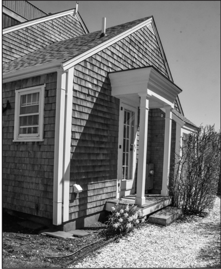
Photo 5: West elevation - overall view.
