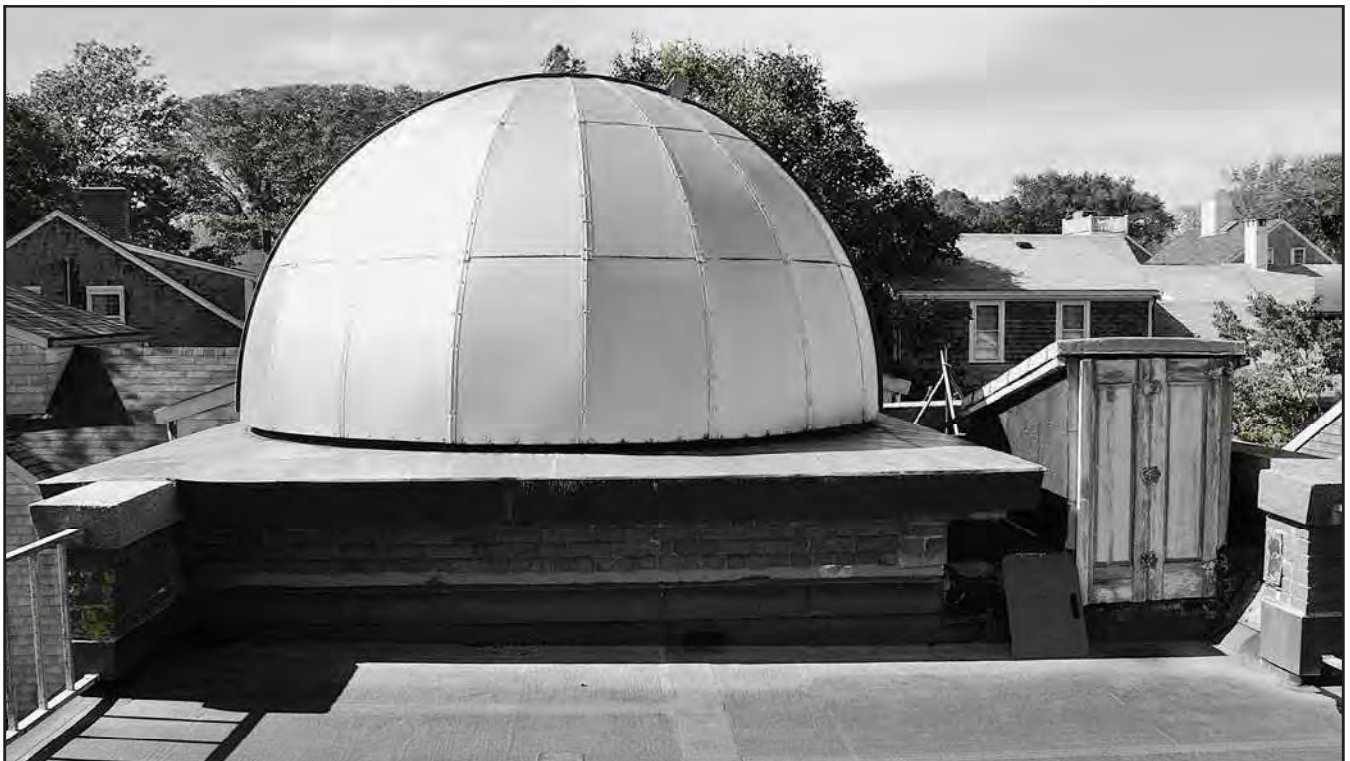
Photo 7: East elevation of Observatory dome, headhouse for staircase, & roof as seen from roof of Astronomical Study
