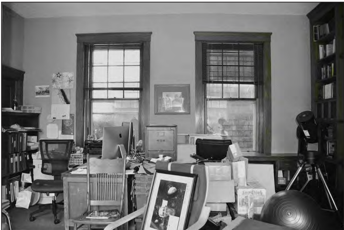
Photo 26: Astronomical Study – 1st story north wall showing original windows, plaster wall, and woodwork trim
