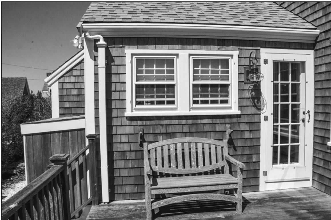
Photo 6: South elevation - kitchen wing - detail of south kitchen entry and storage sheds (photo left).
