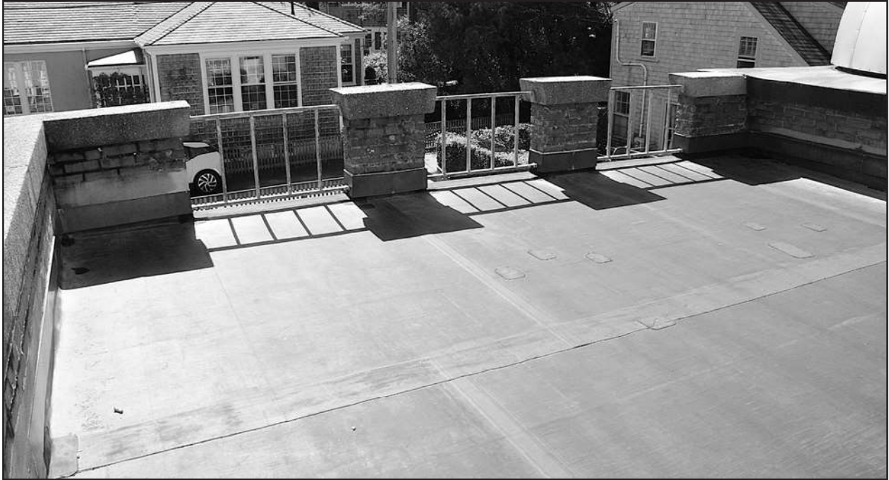
Photo 10: Astronomical Study – south side of roof, showing membrane roofing, railings, & brick piers with cast-stone caps
