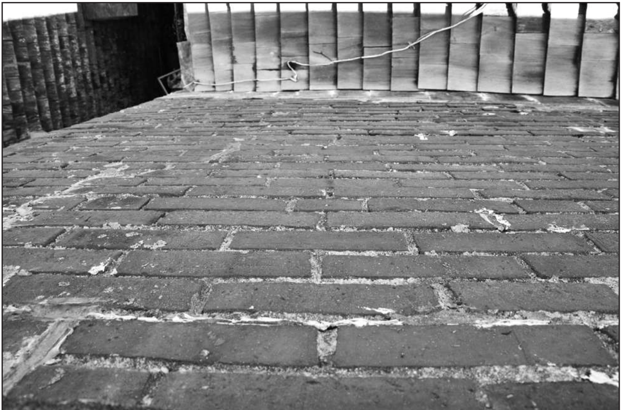
Photo 9: East elevation of Astronomical Study showing typical brickwork above 1st story wood-shingle roof of attached Maria Mitchell House
