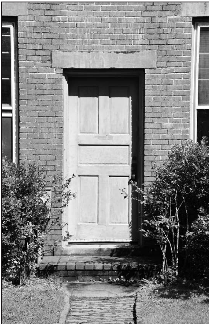
Photo 5: Façade (south elevation) of Astronomical Study – detail of entry & masonry
