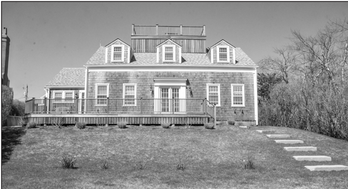
Photo 11: South elevation - overall view, including stone steps leading to rear (south) lawn.
