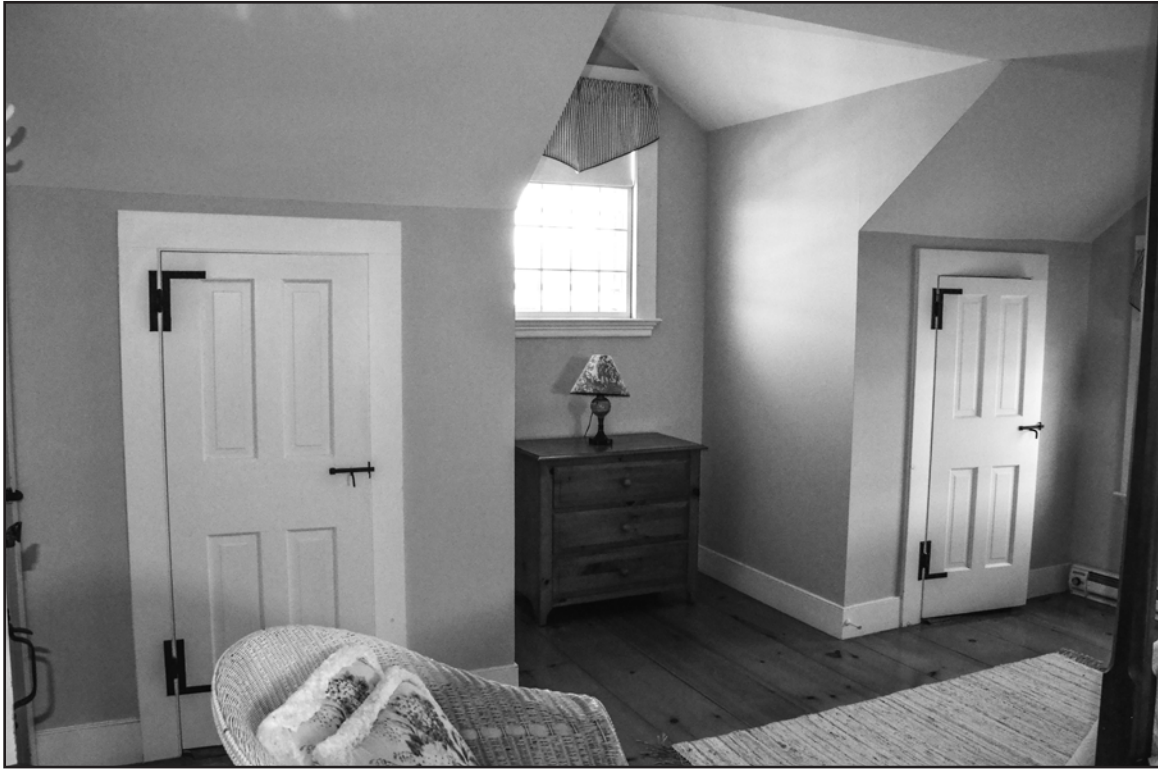
Photo 34: Interior - 2nd floor - Bedroom #2 - north end. This layout of corner closets flanking the dormer is mirrored at the south end of this room and at both ends of Bedroom #3.
