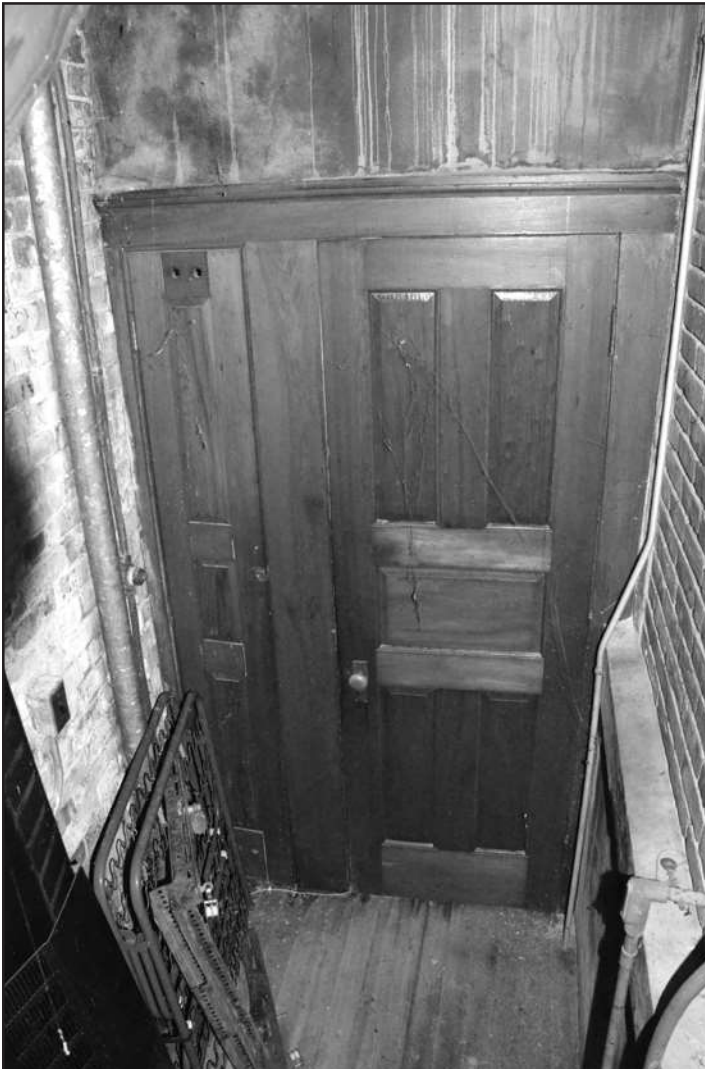
Photo 18: Observatory interior – basement level of east end of staircase
