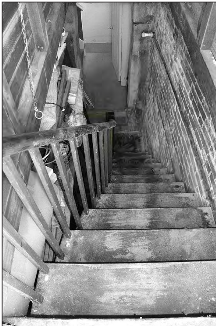
Photo 21: Observatory interior – 2nd story stair seen from roof headhouse looking west to 1st story
