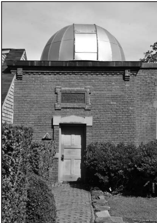
Photo 2: Façade (south elevation) of Observatory
