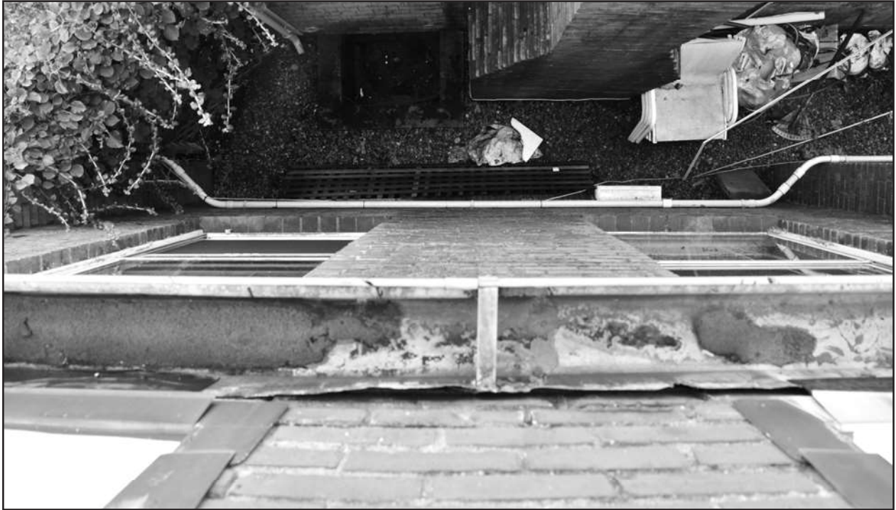
Photo 8: North elevation (east end) of Observatory from roof – built at property line and inaccessible except for oblique views
