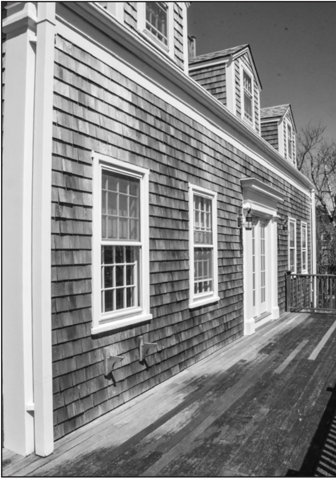
Photo 9: South elevation - entry & deck - showing typical eave.
