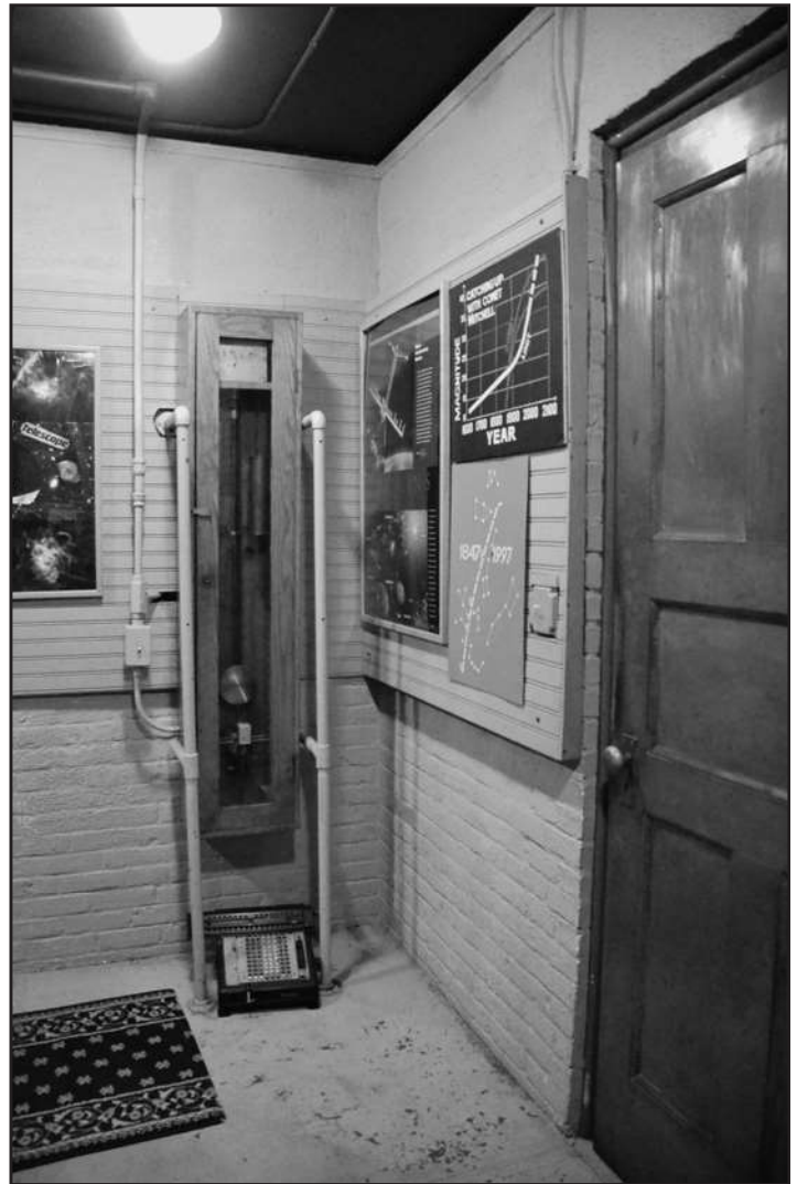
Photo 15: Observatory interior - 1st story showing north wall with oak case containing weights and east wall with partial view of copper-clad door frame & door leading to Astronomical Study
