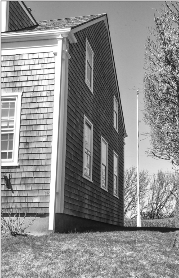
Photo 13: East elevation - overall view looking northwest.
