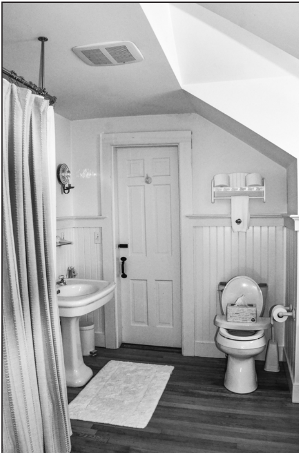
Photo 38: Interior - 2nd floor - Bathroom - west wall of room showing original sink and door.
