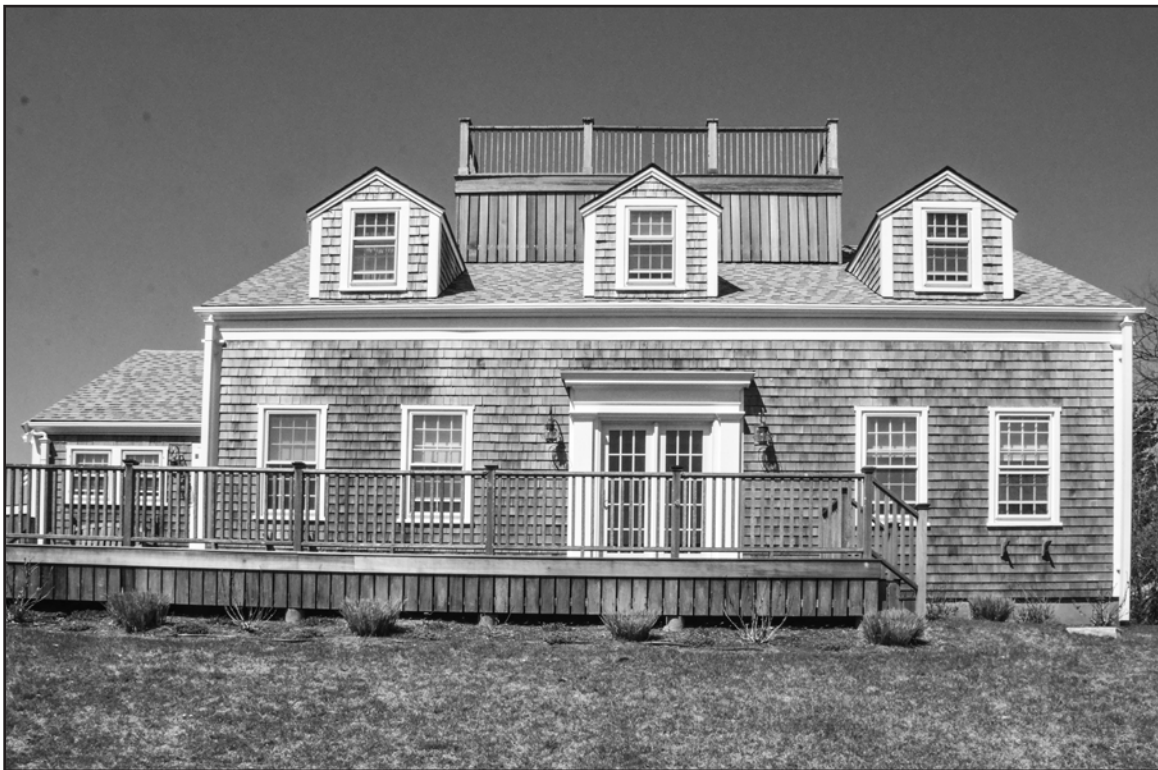
Photo 8: South elevation - overall view.
