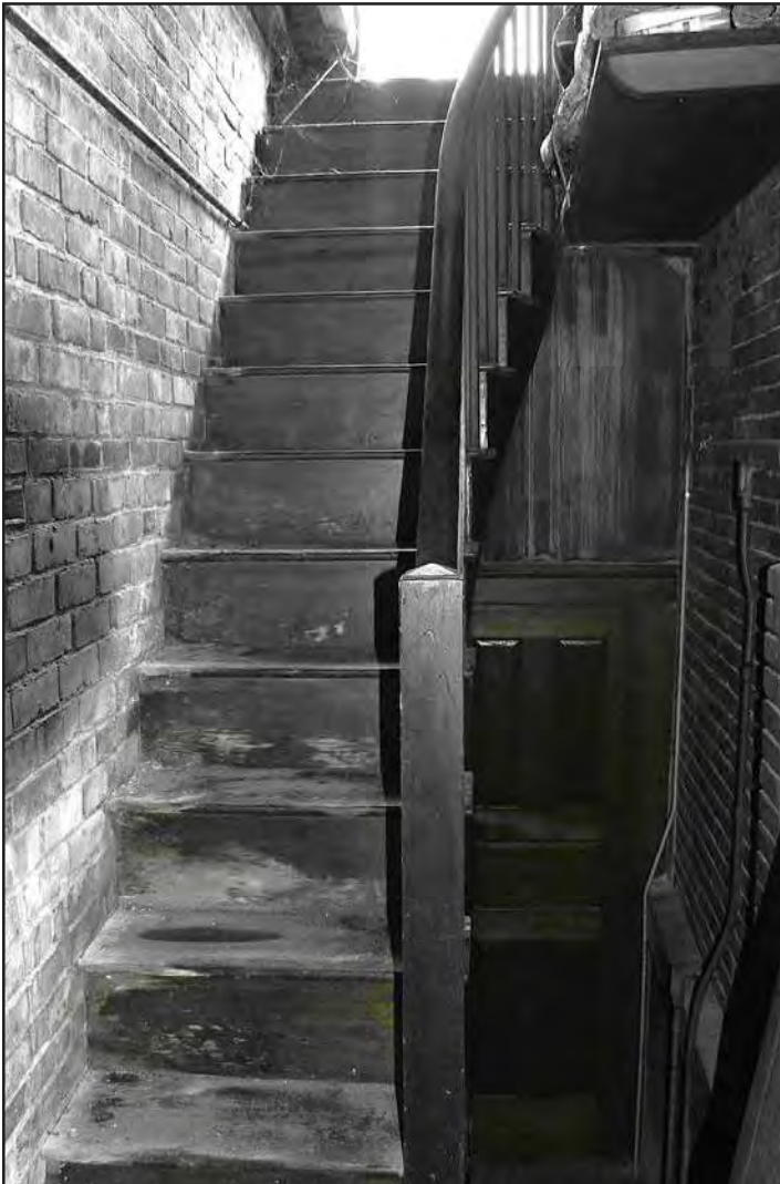
Photo 20: Observatory interior – 2nd story stair at west end of stairhall leading to headhouse at roof
