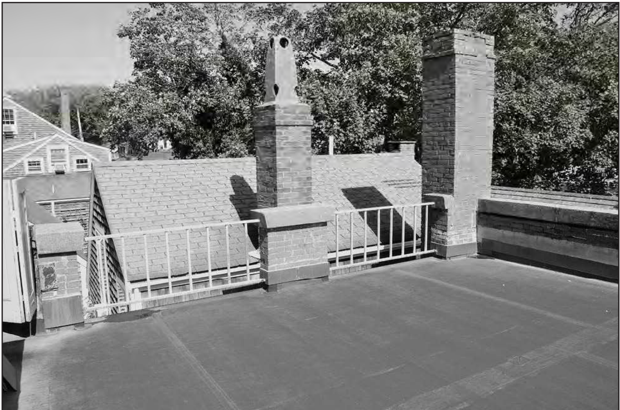
Photo 11: Astronomical Study – north side of roof, showing membrane roofing, railings, brick piers with cast-stone caps, & brick piers with cast-stone caps
