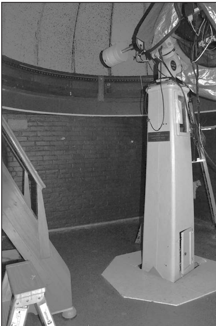
Photo 22: Observatory interior – 2nd story showing brick drum with dome, telescope & telescope pier, & moveable stepladder
