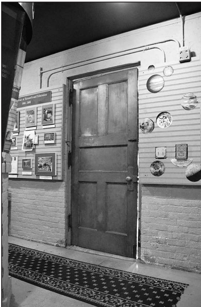
Photo 16: Observatory interior – 1st story showing south wall with copper-clad casing and door
