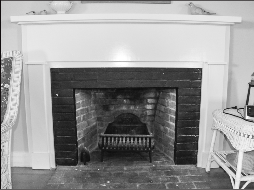
Photo 36: Interior - 2nd floor - Bedroom #2 - detail of west wall fireplace.
