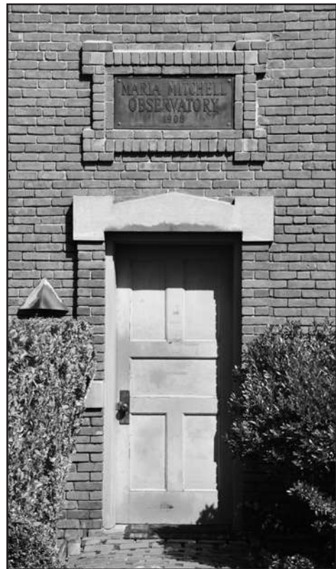
Photo 3: Façade (south elevation) of Observatory showing details of main entry & dedication plaque
