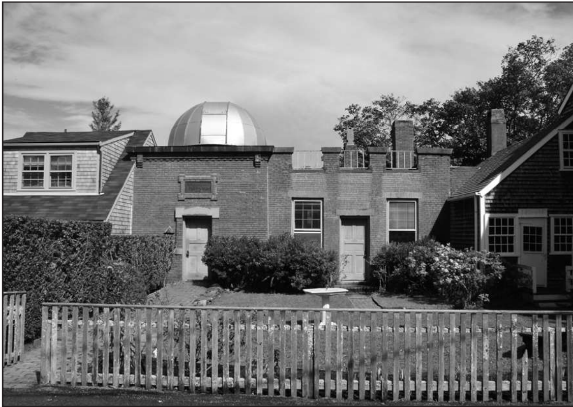
Photo 1: Façade (south elevation) of Observatory (photo left) & Astronomical Study (photo right)
