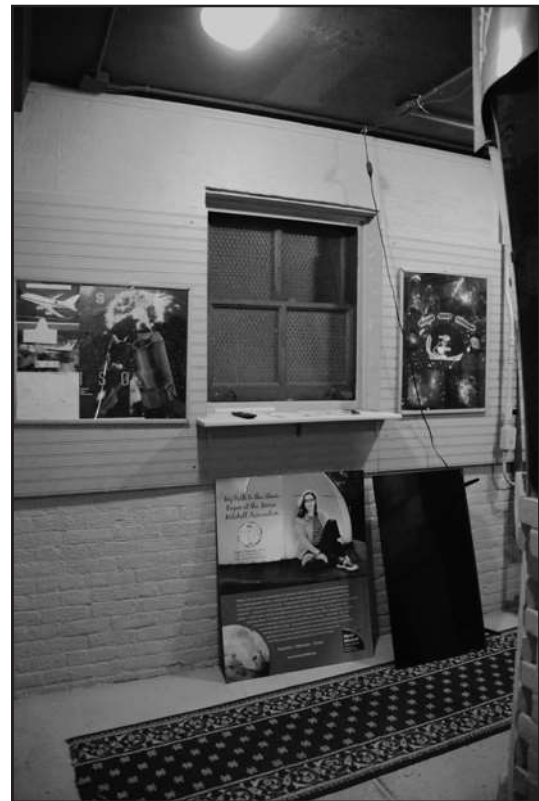
Photo 14: Observatory interior – 1st story showing north wall with copper-clad window & casing, wire glass
