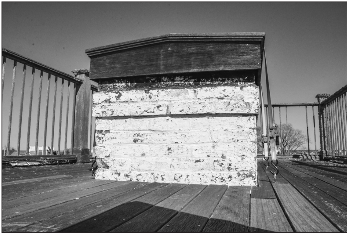
Photo 4: View from widows' walk to capped chimney and typical railing.
