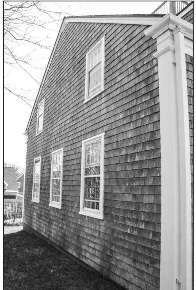
Photo 14: East elevation - overall view looking southwest.
