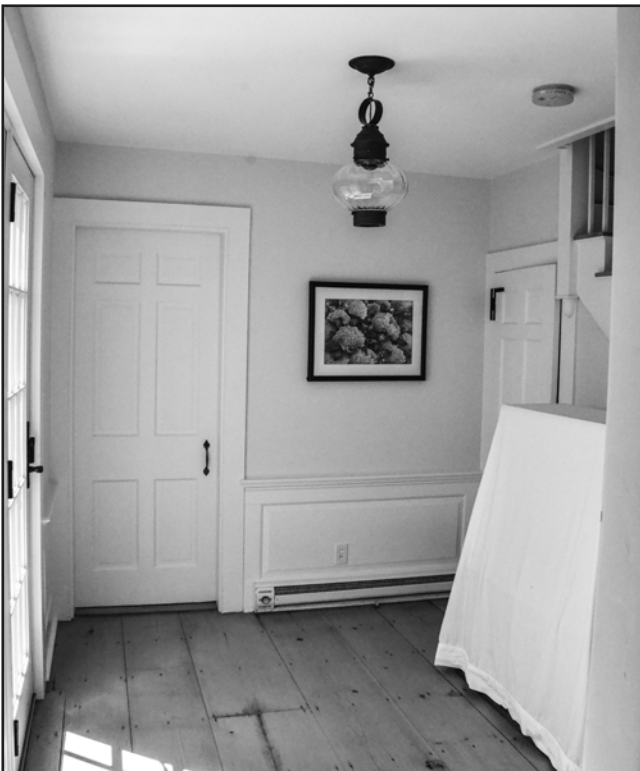
Photo 17: Interior - 1st floor - Entry Foyer - west wall with door to dining room, showing closet door beneath stair on north wall.
