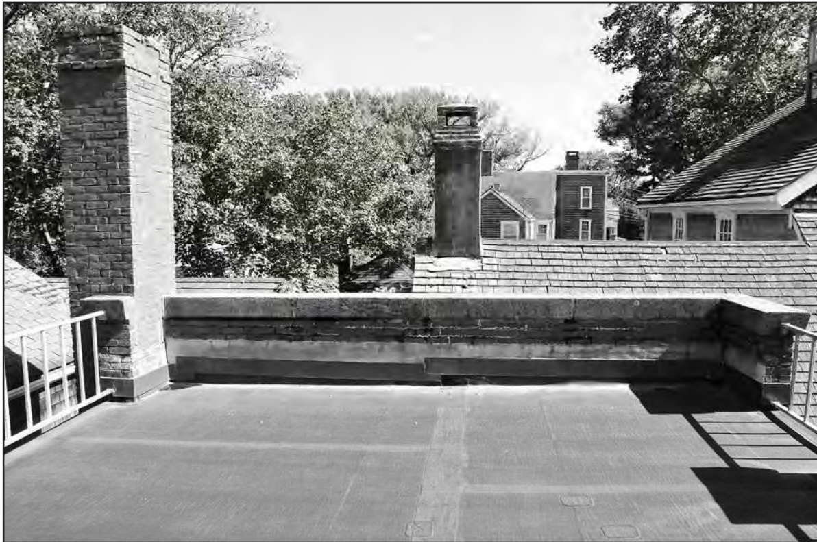
Photo 12: Astronomical Study – east side of roof, showing membrane roofing, chimney (northeast corner), & solid masonry parapet
