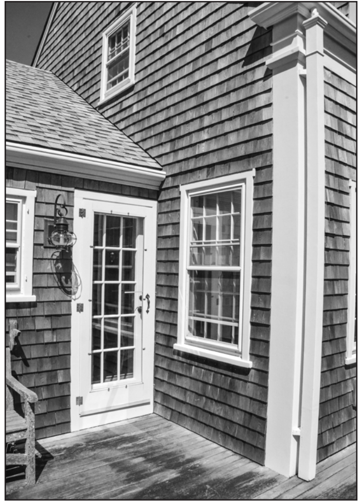
Photo 10: South elevation - kitchen wing - detail of corner pilaster, entablature & typical window surround.
