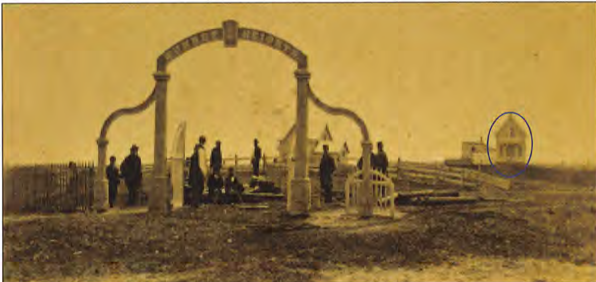
GPNsg14282 Entry gate to Sunset Heights development.
