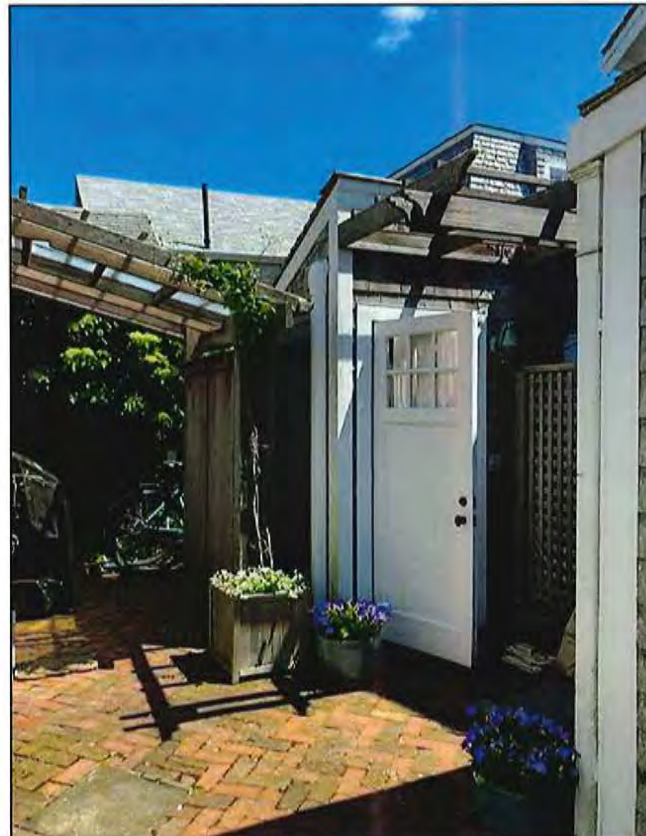
Shower Entrance at West Elevation
