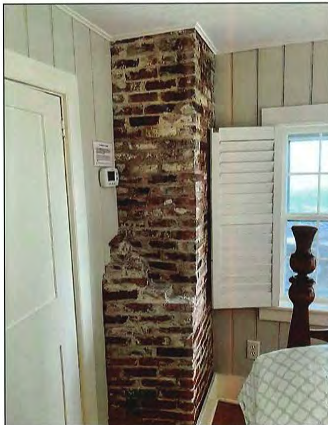
Brick Chimney, South Bedroom First Floor
