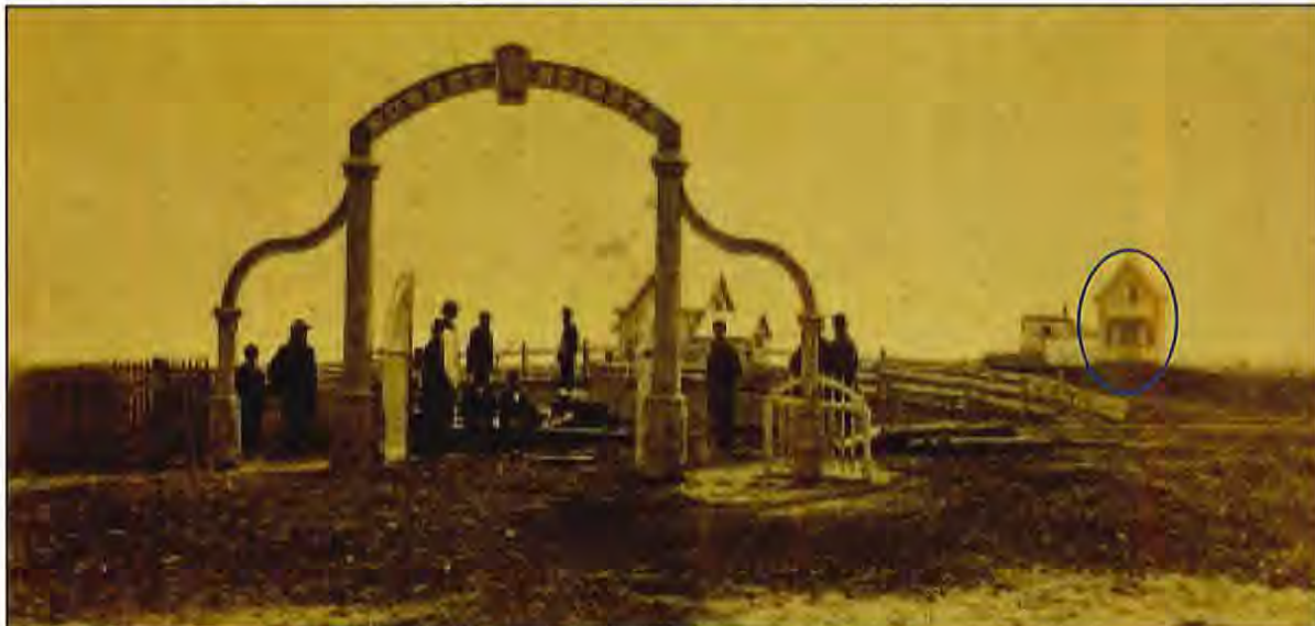
GPNsg14282 Entry gate to Sunset Heights development.
