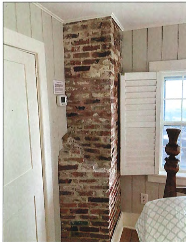
Brick Chimney, South Bedroom First Floor
