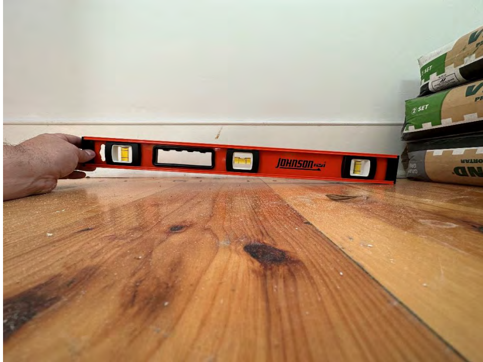
Photo 18 - Main floor level (Interior)
