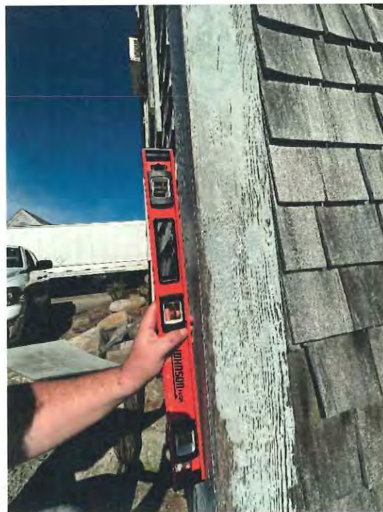
Photo 6- Waterside exterior corner
