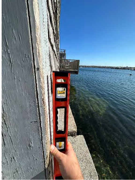
Photo 7 - Waterside exterior corner
