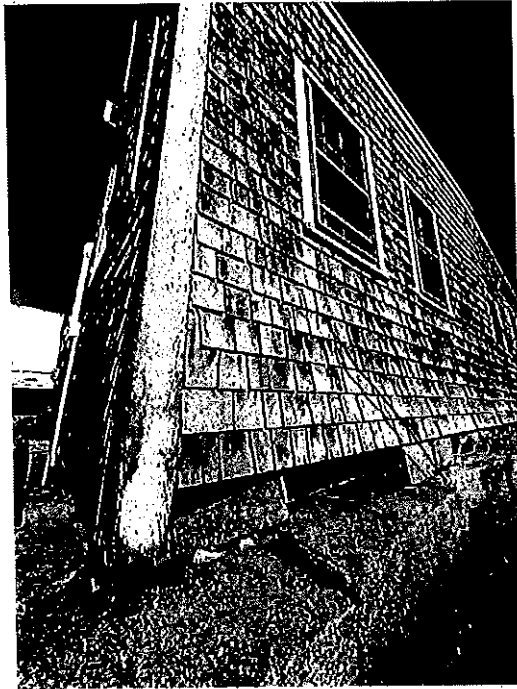
Photo 5- Waterside exterior corner
