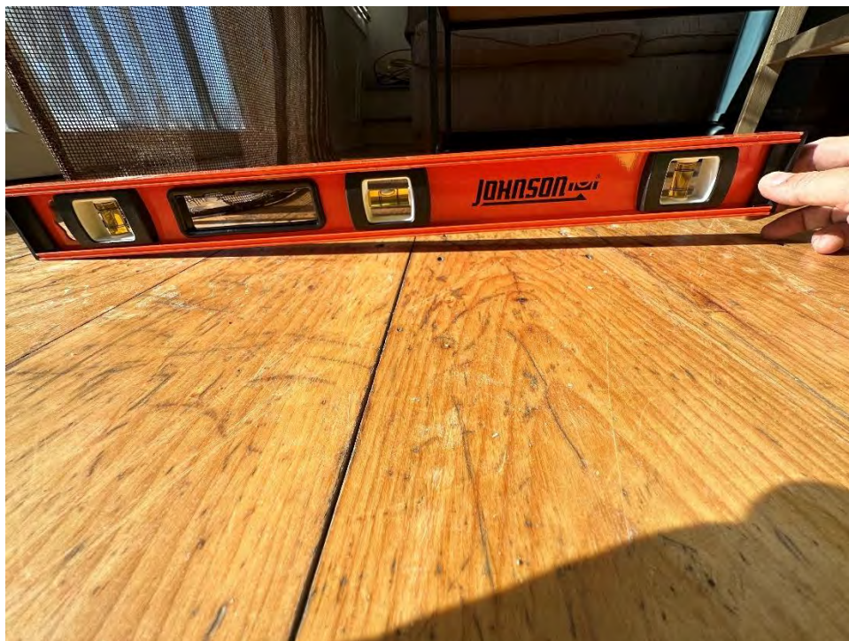
Photo 19 - Main floor level (Interior)
