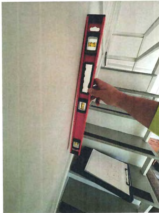
Photo 21 - Second level gable end wall (Interior)
