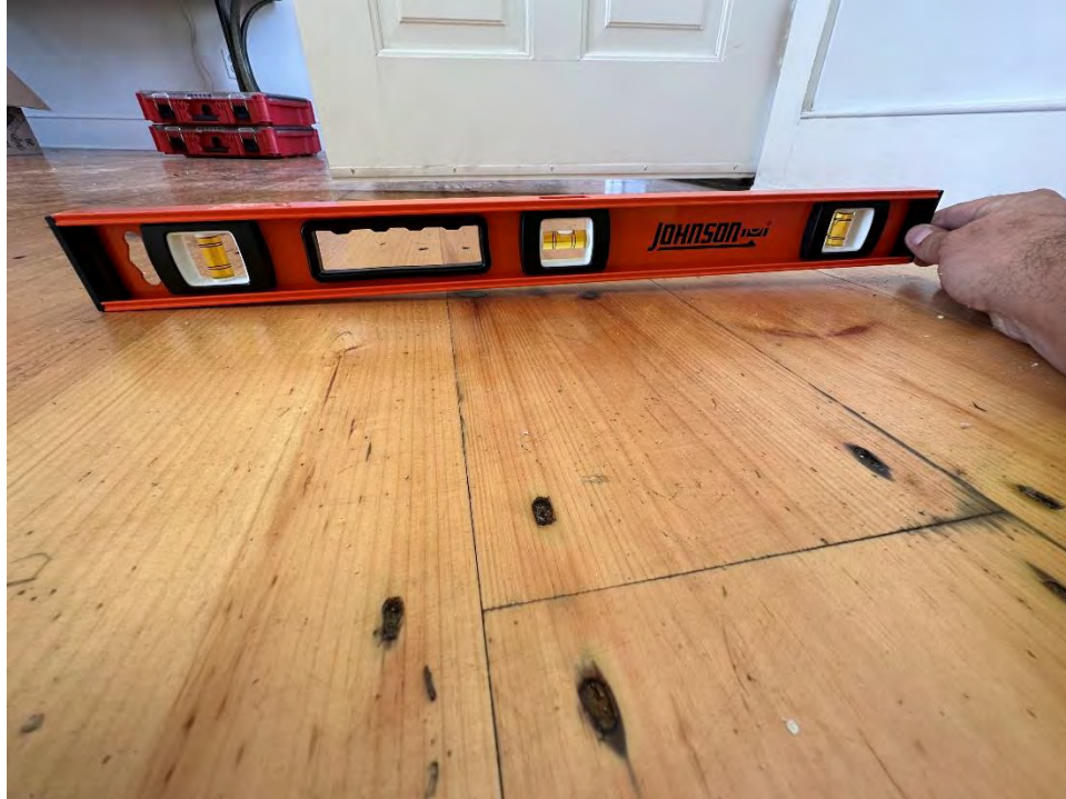
Photo 20 - Main floor level (Interior)
