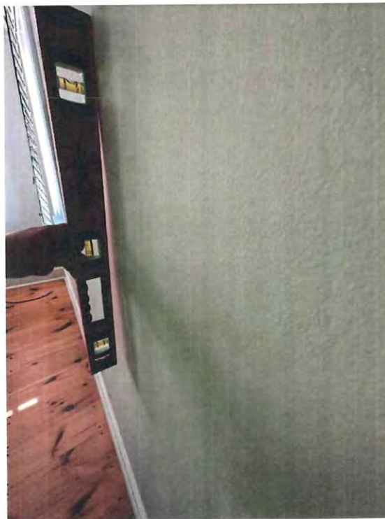
Photo 12 - Bearing wall waterside bow
