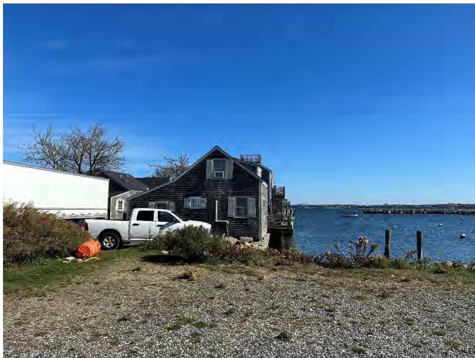
Photo 2-Exterior view from Petral Landing
