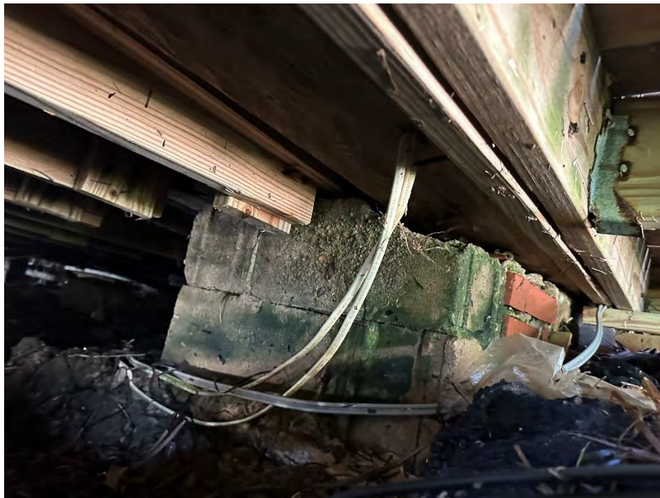
Photo 31 - Framing built on chimney (Crawl Space)
