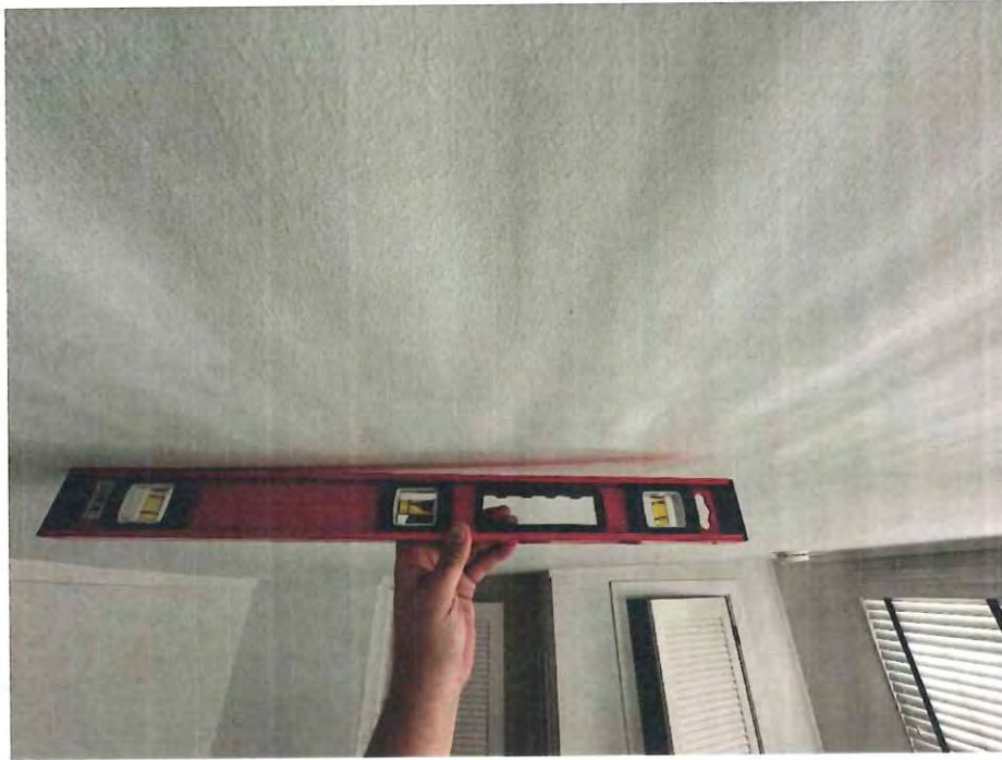
Photo 13 - Ceiling/Second floor slope (Interior)
