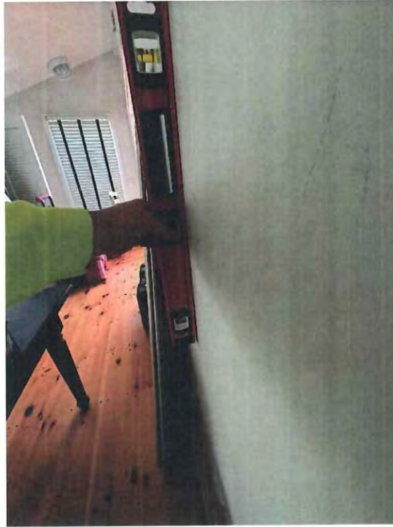
Photo 16 - Kitchen wall/bearing wall (Interior)
