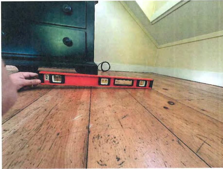
Photo 22 - Second floor level (Interior)
