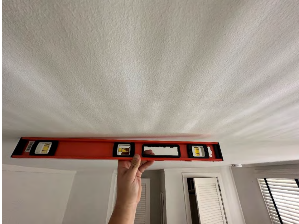
Photo 13 - Ceiling/Second floor slope (Interior)
