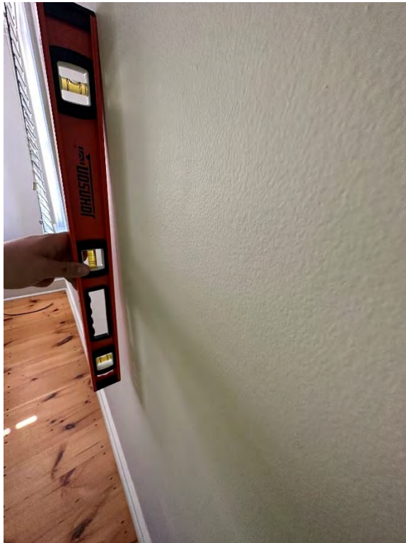
Photo 12 - Bearing wall waterside bow
