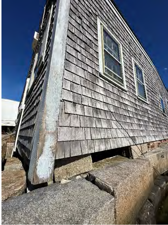
Photo 5- Waterside exterior corner
