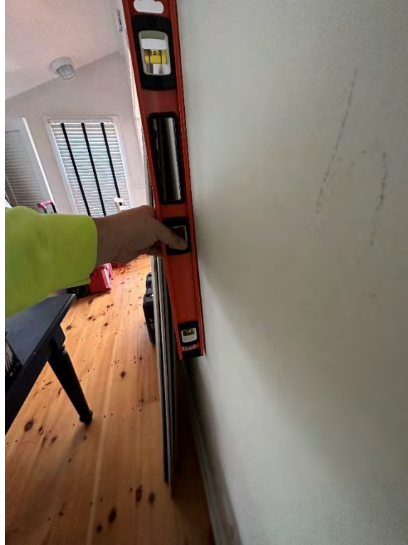
Photo 16 - Kitchen wall/bearing wall (Interior)
