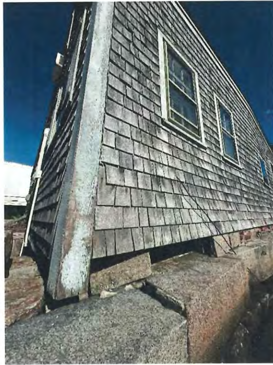
Photo 5- Waterside exterior corner
