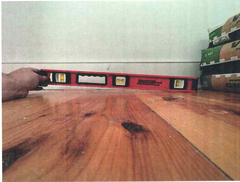
Photo 18 - Main floor level (Interior)
