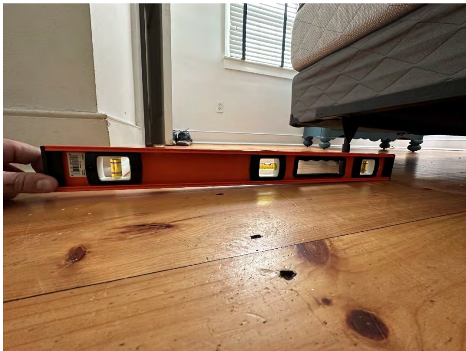
Photo 14 - First floor waterside slope (Interior)
