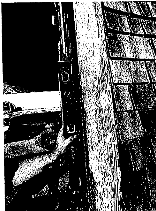
Photo 6- Waterside exterior corner
