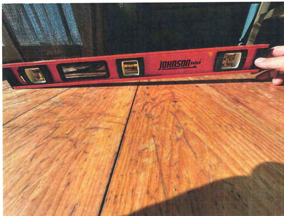
Photo 19 - Main floor level (Interior)
