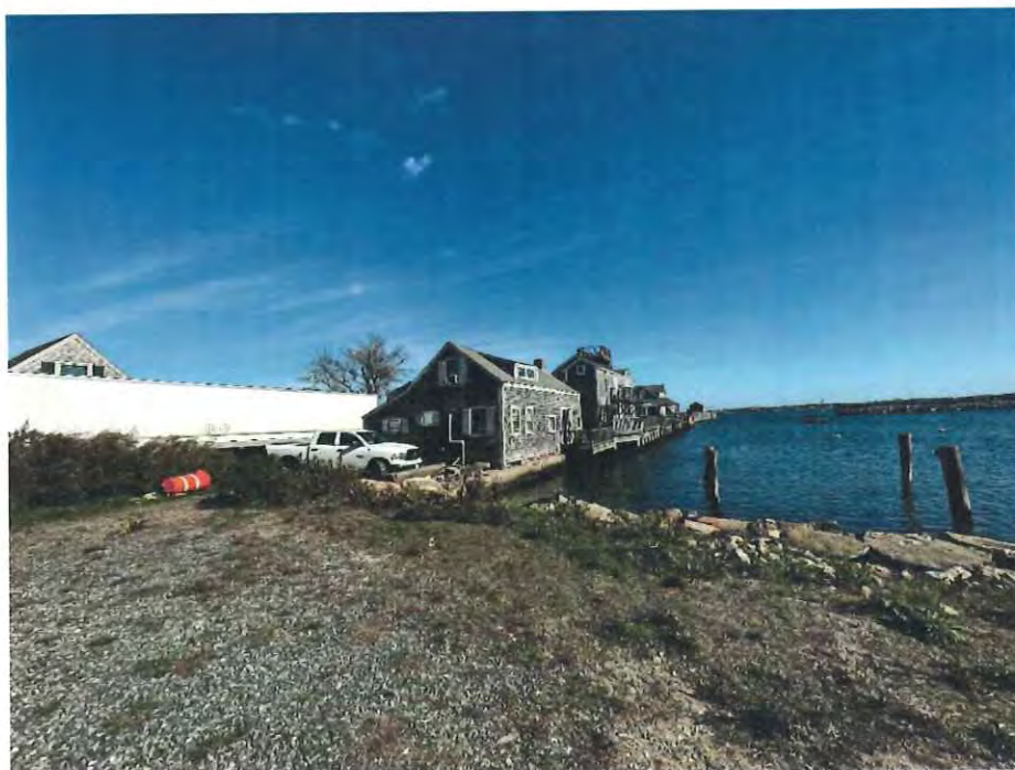
Photo 1 -Exterior view from Petral Landing
