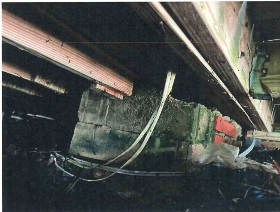
Photo 31 - Framing built on chimney (Crawl Space)
