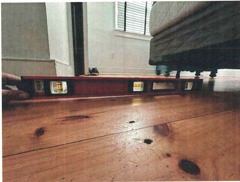
Photo 14 - First floor waterside slope (Interior)
