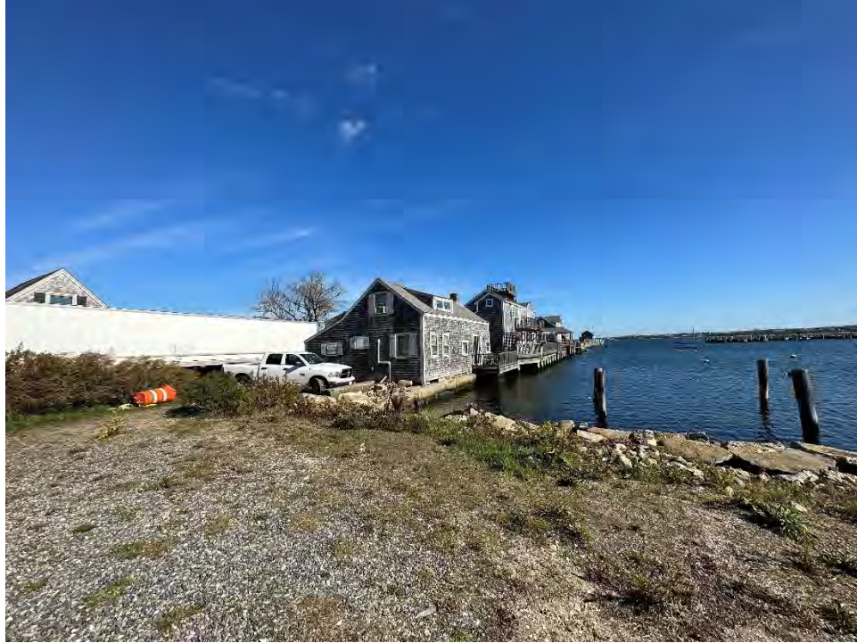
Photo 1 -Exterior view from Petral Landing
