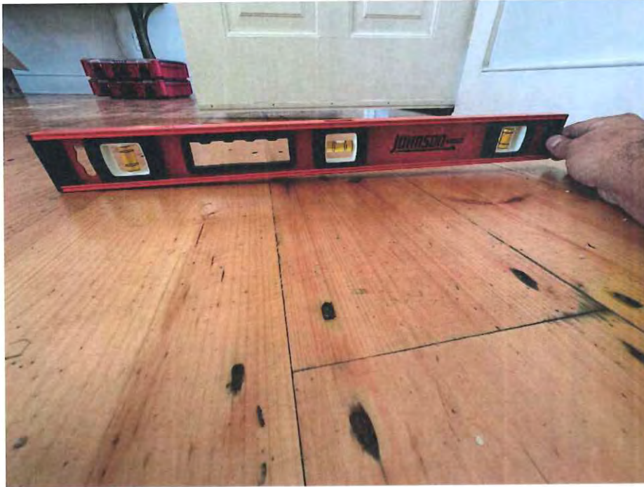
Photo 20 - Main floor level (Interior)
