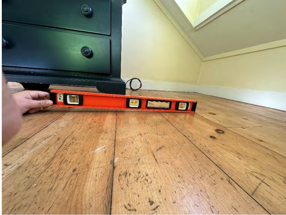
Photo 22 - Second floor level (Interior)
