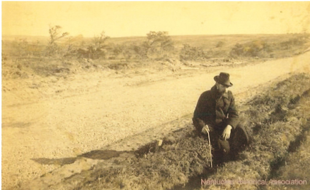
Milestone road construction underway with a man measuring the depth of an old rutted road beside it. 1894. Courtesy Nantucket Historical Association.
