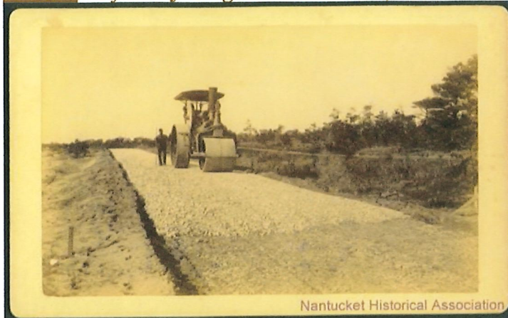
Road roller at work on Milestone Road, Siasconset, Nantucket. 1899. Courtesy Nantucket Historical Association.
