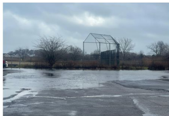
Flooding in the Beachmont VFW parking lot looking towards Frederick's Park (December 2022)
