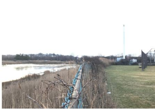
Fredericks Park (right) and wetlands (left) separate by a chain link fence (looking west)
