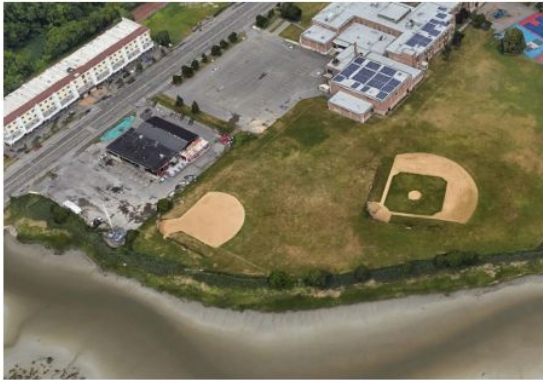
Aerial image of Fredericks Park in Revere
