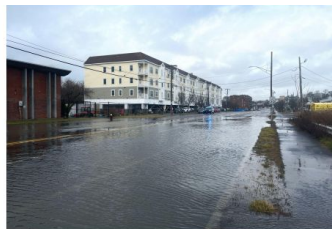
Flooding overtopping Bennington Street looking northbound (December 2022)
