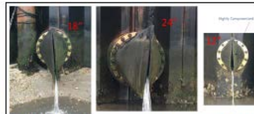
Figure 14: Visual Inspection of the ProFlex Check Valves at the Easy Street Bulkhead (2/13/2020)
