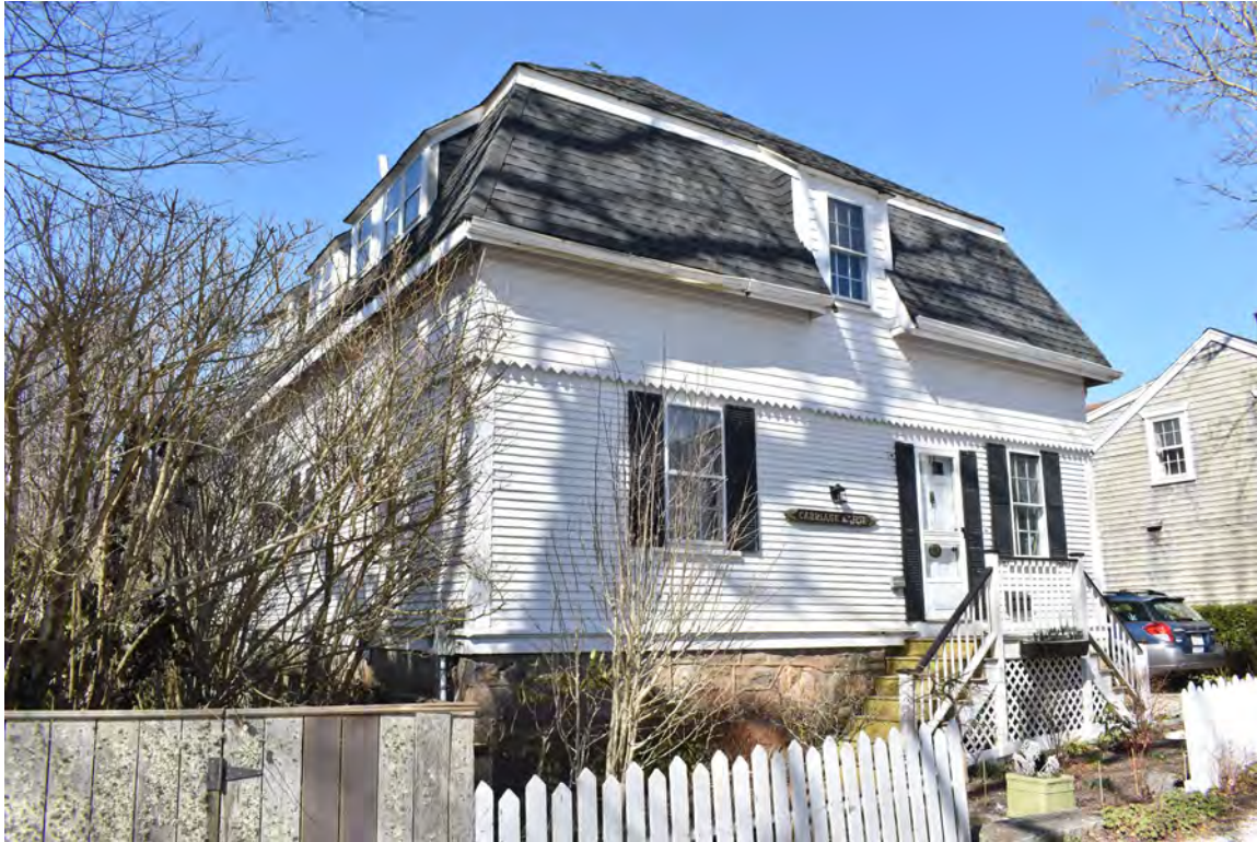
Photo 2. 5 Rays Court, looking northeast.
