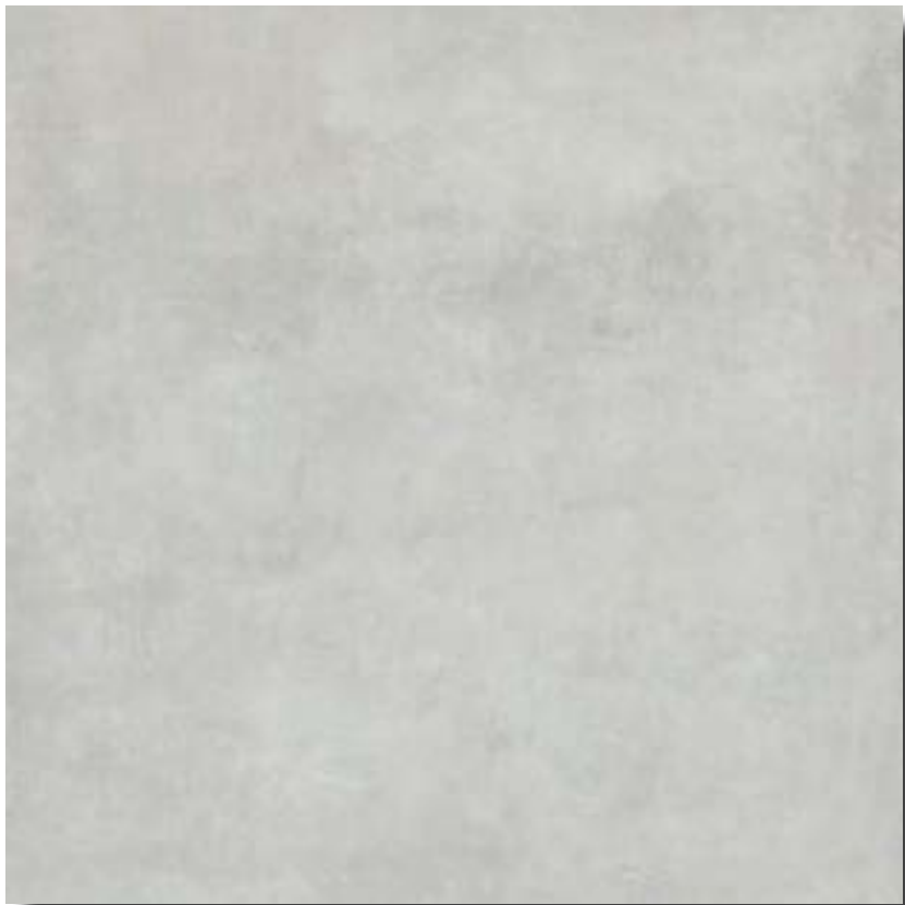
RETAINING WALLS - PARGED CONCRETE
