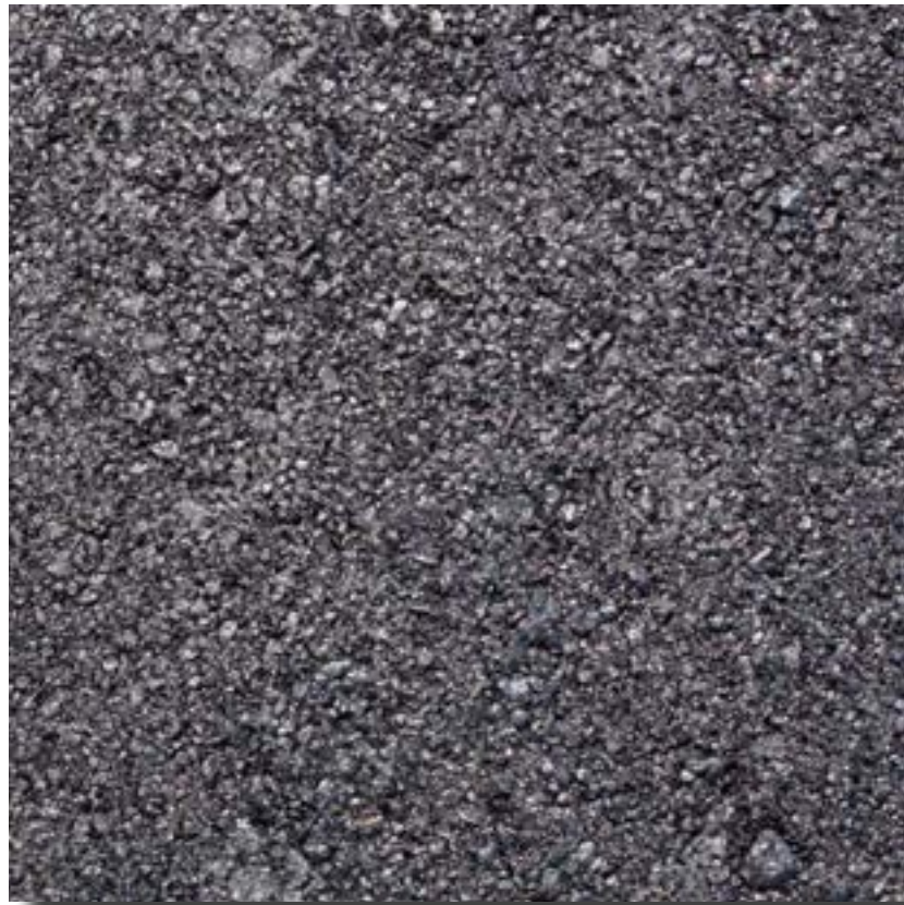
ROADWAY - BLACK TOP ASPHALT
