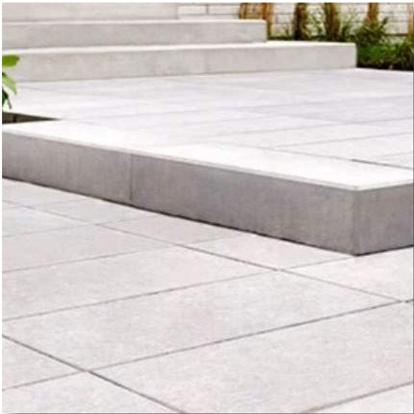
RISERS - CONCRETE BLOCKS
