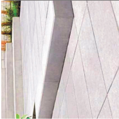
RISERS - CONCRETE BLOCKS
