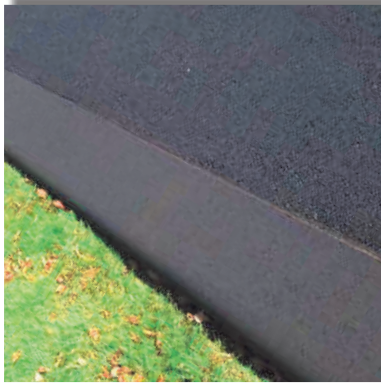
CAPE COD BERM - BLACK TOP ASPHALT
