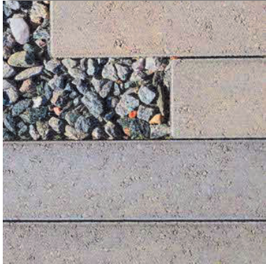
PATIOS - CONCRETE PAVERS
