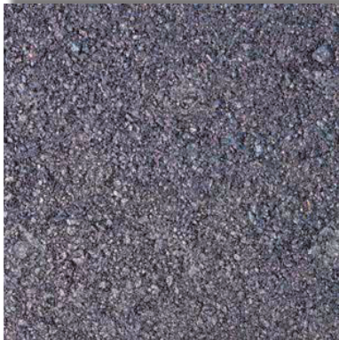
ROADWAY - BLACK TOP ASPHALT
