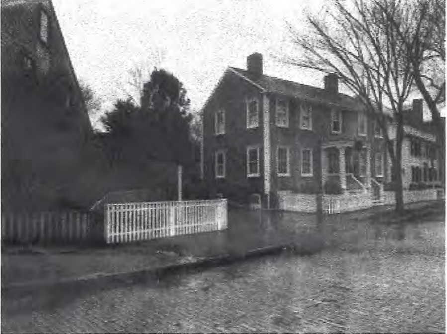
4 VIEW 2 MAIN ST
