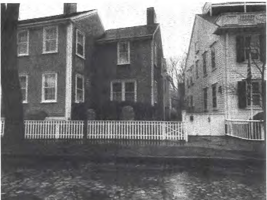
6 VIEW 4 MAIN ST
