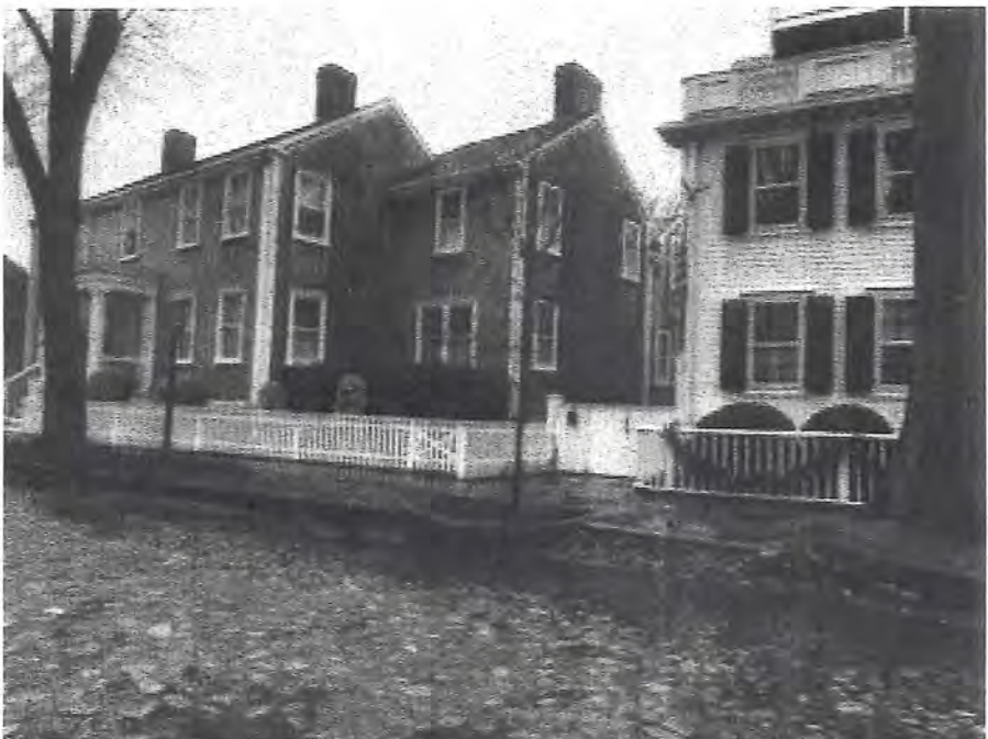
8 VIEW 6 MAIN ST
