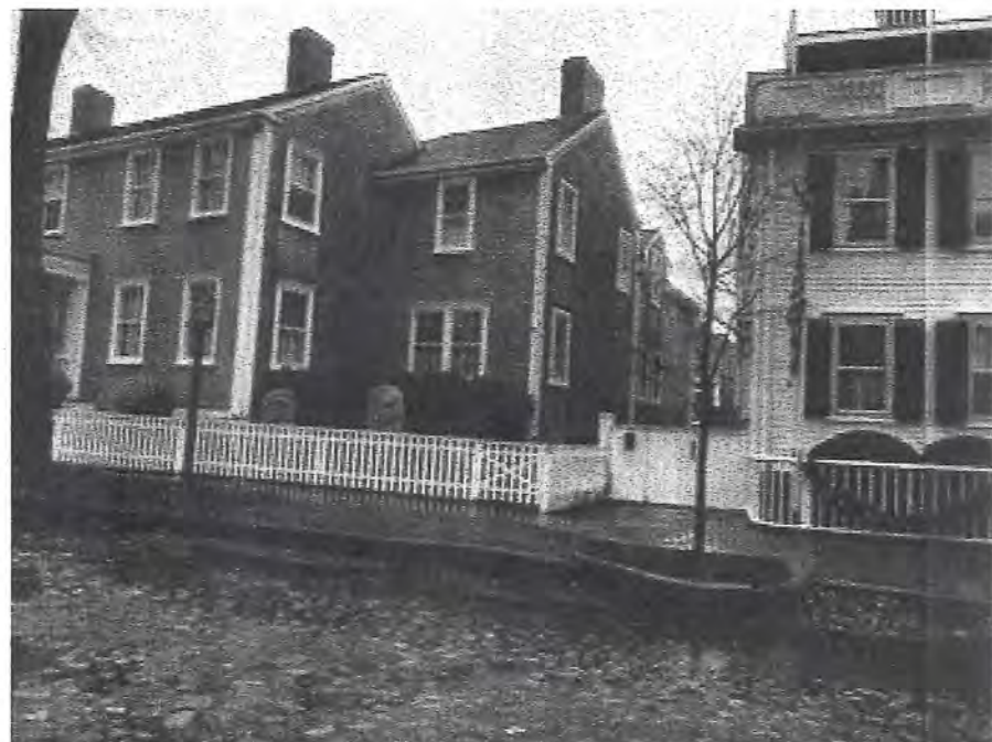
7 VIEW 5 MAIN ST
