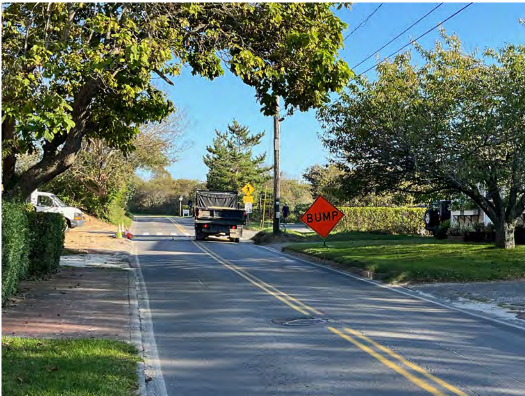
Temporary 'Bump' at utility connection at Pedestrian Bike Crossing.
