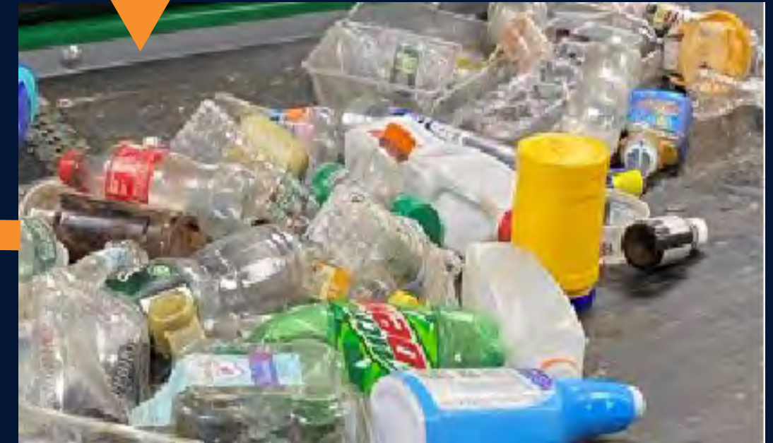
Picking conveyor (pickers not shown)
