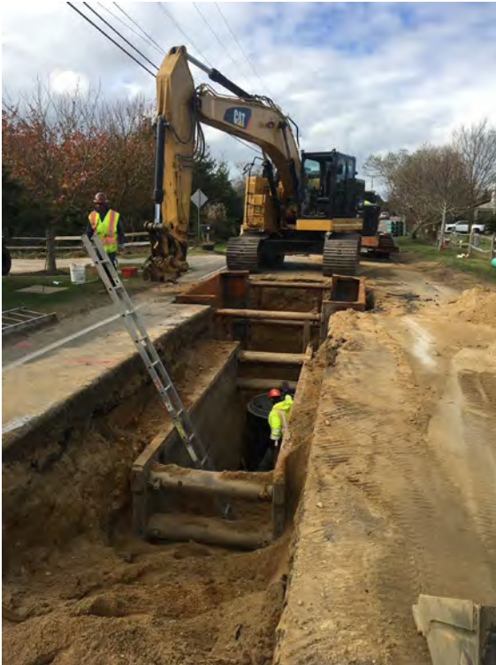
Wastewater (Sewer and Septic)
