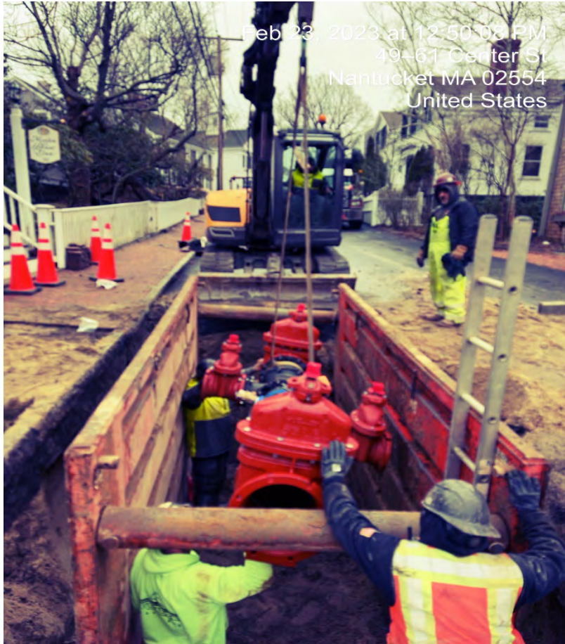
Water Gate Valve Installation
