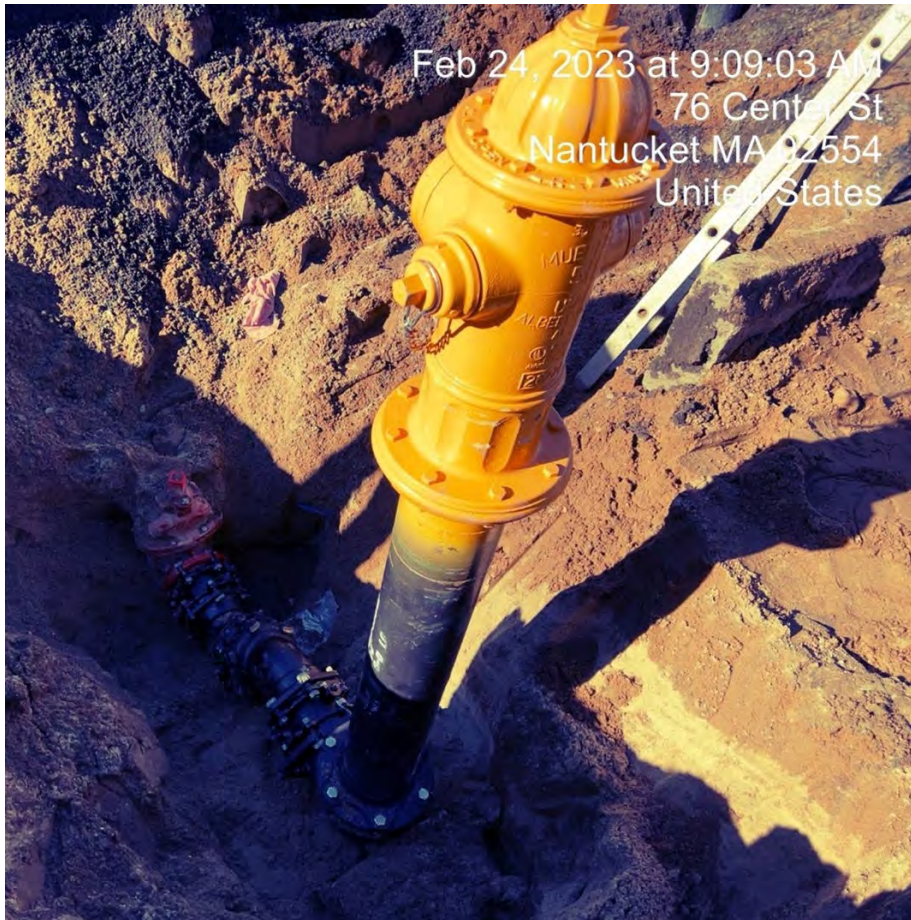
Fire Hydrant Installation
