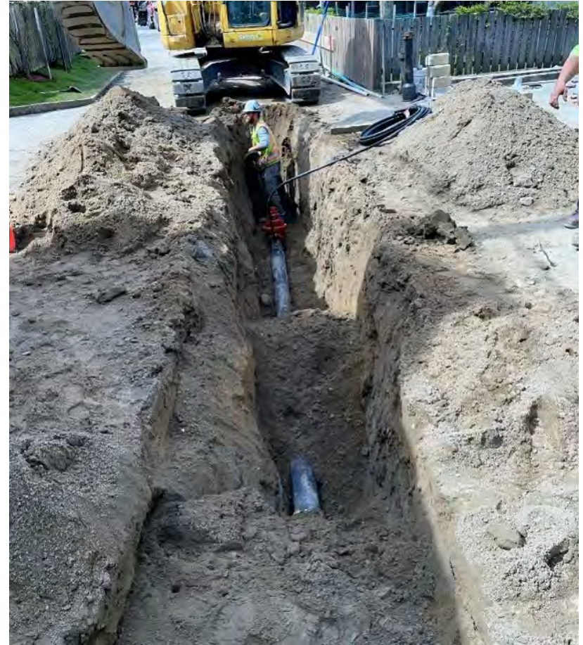
Water Main Installation
