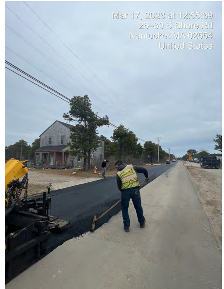
Temporary Trench Paving
