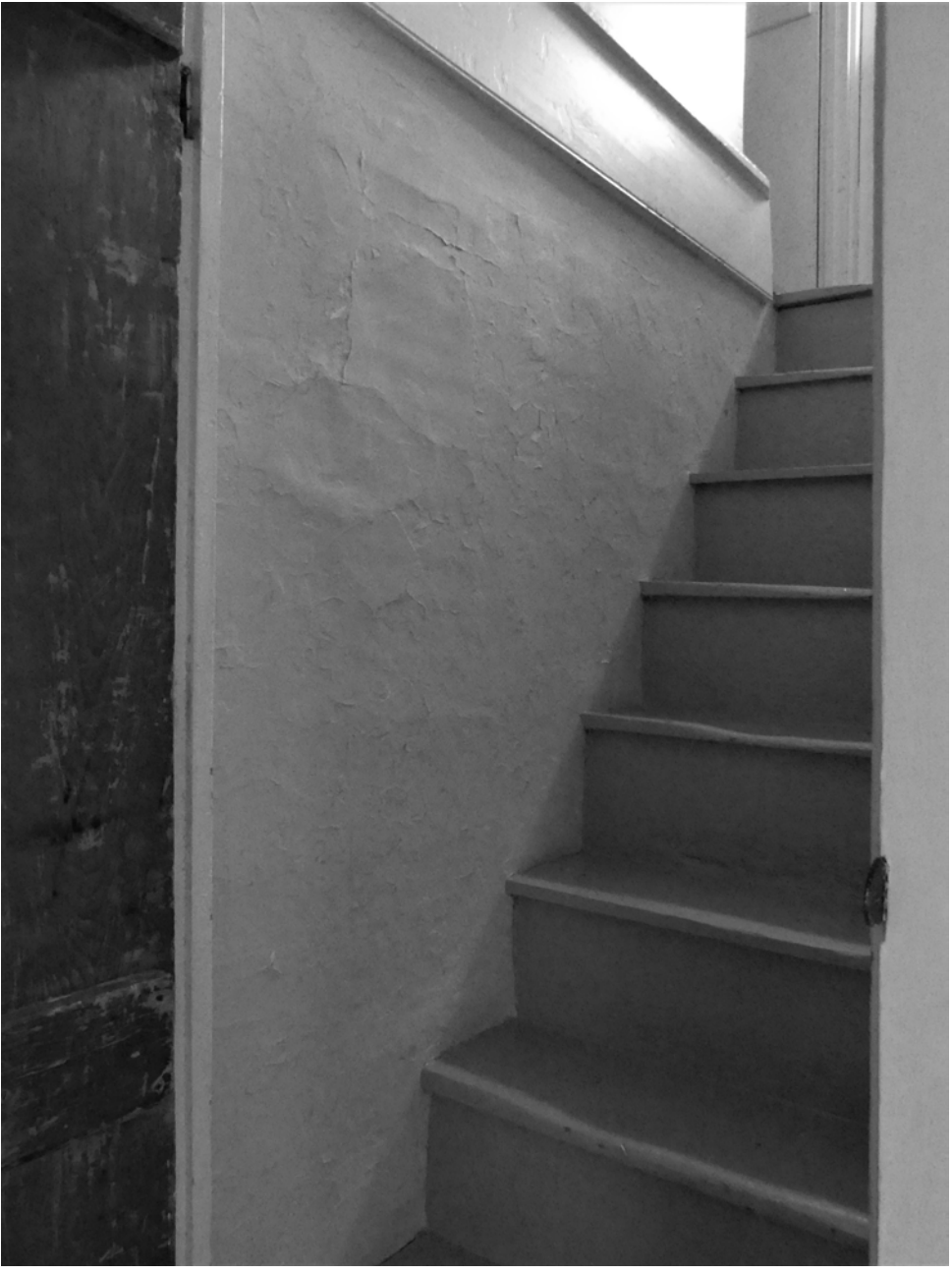
Photo #20 – interior 1 st floor at rear ell showing rear staircase with lime plaster wall & original stair treads & risers
