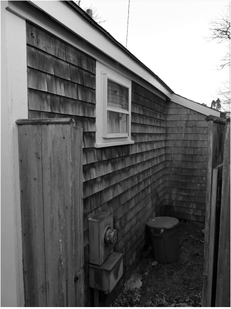
Photo #36 – Cottage – west elevation
