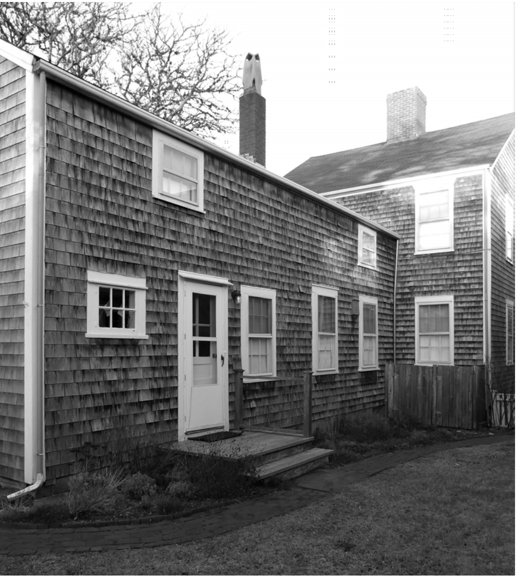
Photo #7 – south elevation of rear ell & partial west elevation of main block of house
