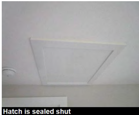
Hatch is sealed shut
