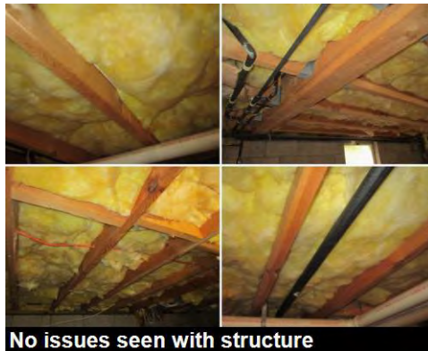
No issues seen with structure
