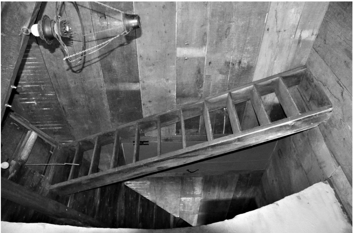
Photo #29 – interior attic – ladder stair to roof hatch
