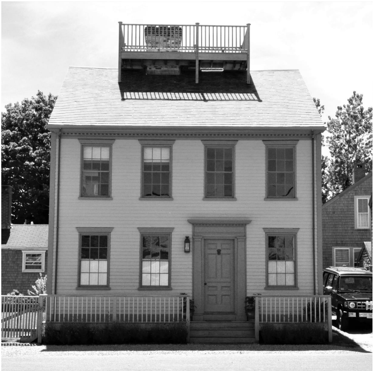
Photo #1 – façade (east elevation)
