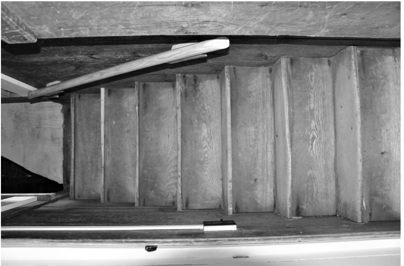
Photo #27 – interior 2 nd storey staircase to attic
