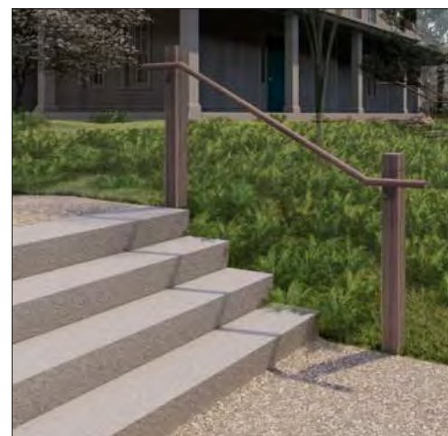
⑰ GRANITE STAIRS WITH WOOD HANDRAIL
