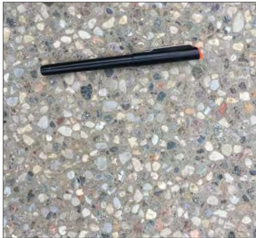
① EXPOSED AGGREGATE CONCRETE TERRACE small driftwood aggregate mix
