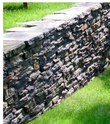
⑯ GOSHEN STONE RETAINING WALL
