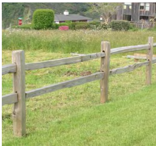
⑦ SPLIT RAIL FENCE
