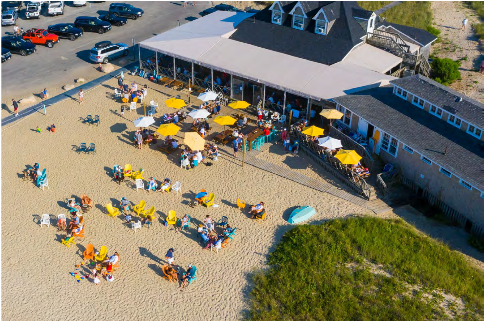
EXISTING BUILDING PHOTOS
