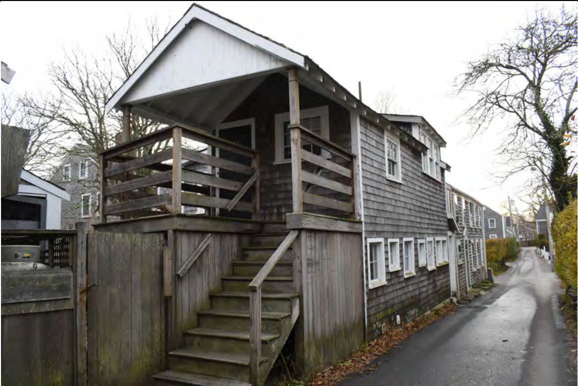
Photo 3. Cottage, looking southwest along Hillers Lane.
