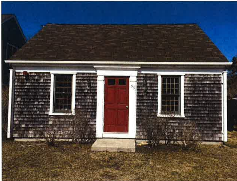
Figure 1: Photo of the South Valley PS building, constructed in 1988.
