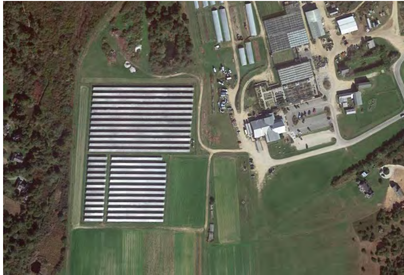
2MWdc solar array at Bartlett's Farm
