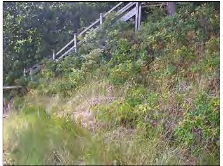
A variety of salt-tolerant vegetation was planted on the face of this bank to stabilize fill added to address bank erosion. (Photo: CZM)
