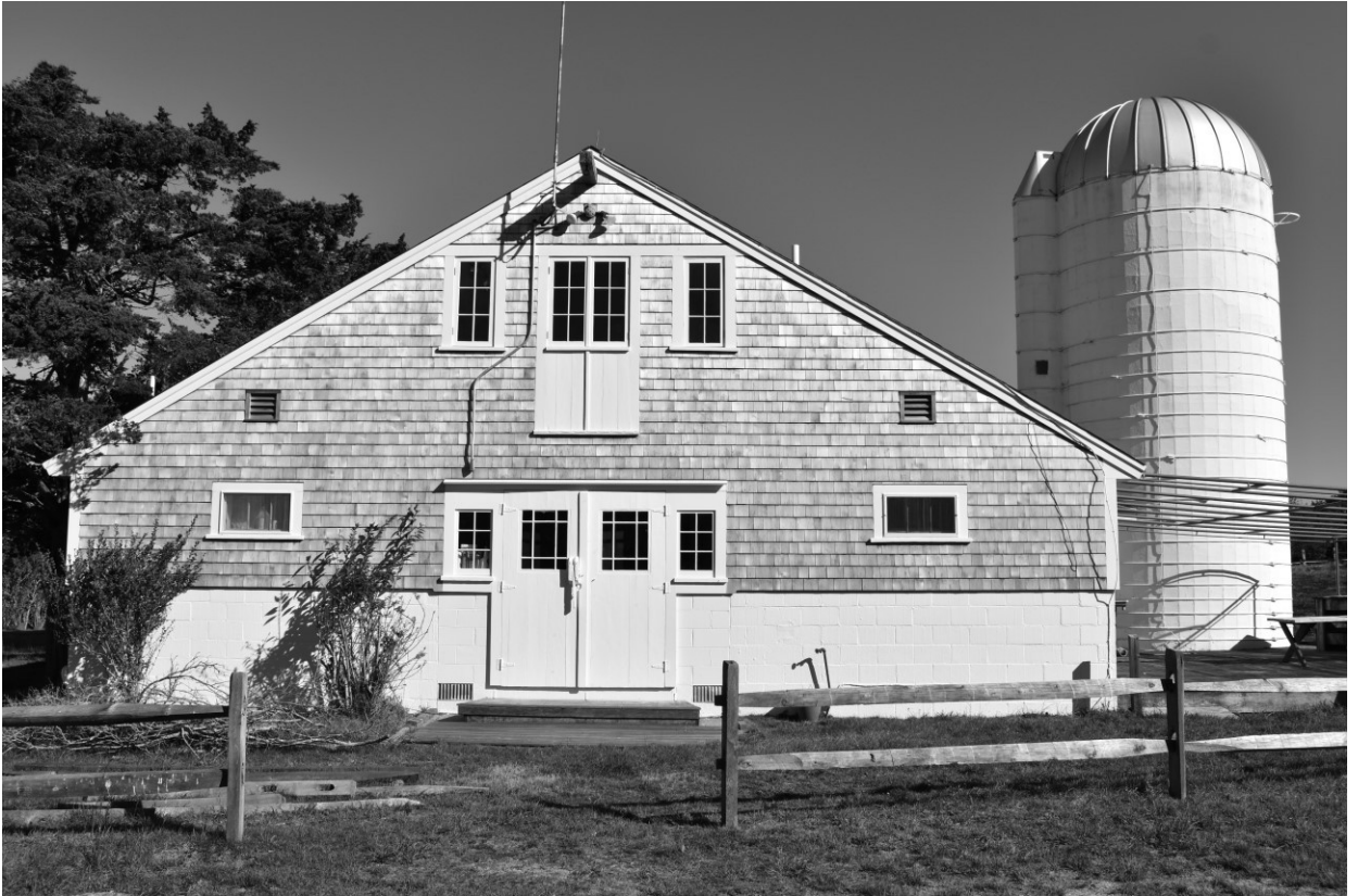
Photo #1 – south elevation of the Barn
