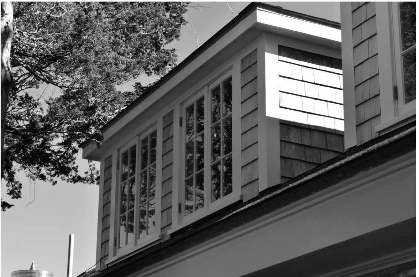
Photo #17 – Barn – west elevation – north dormer
