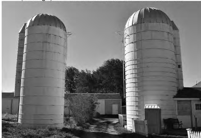
(left to right) East and West Silos – north elevations
