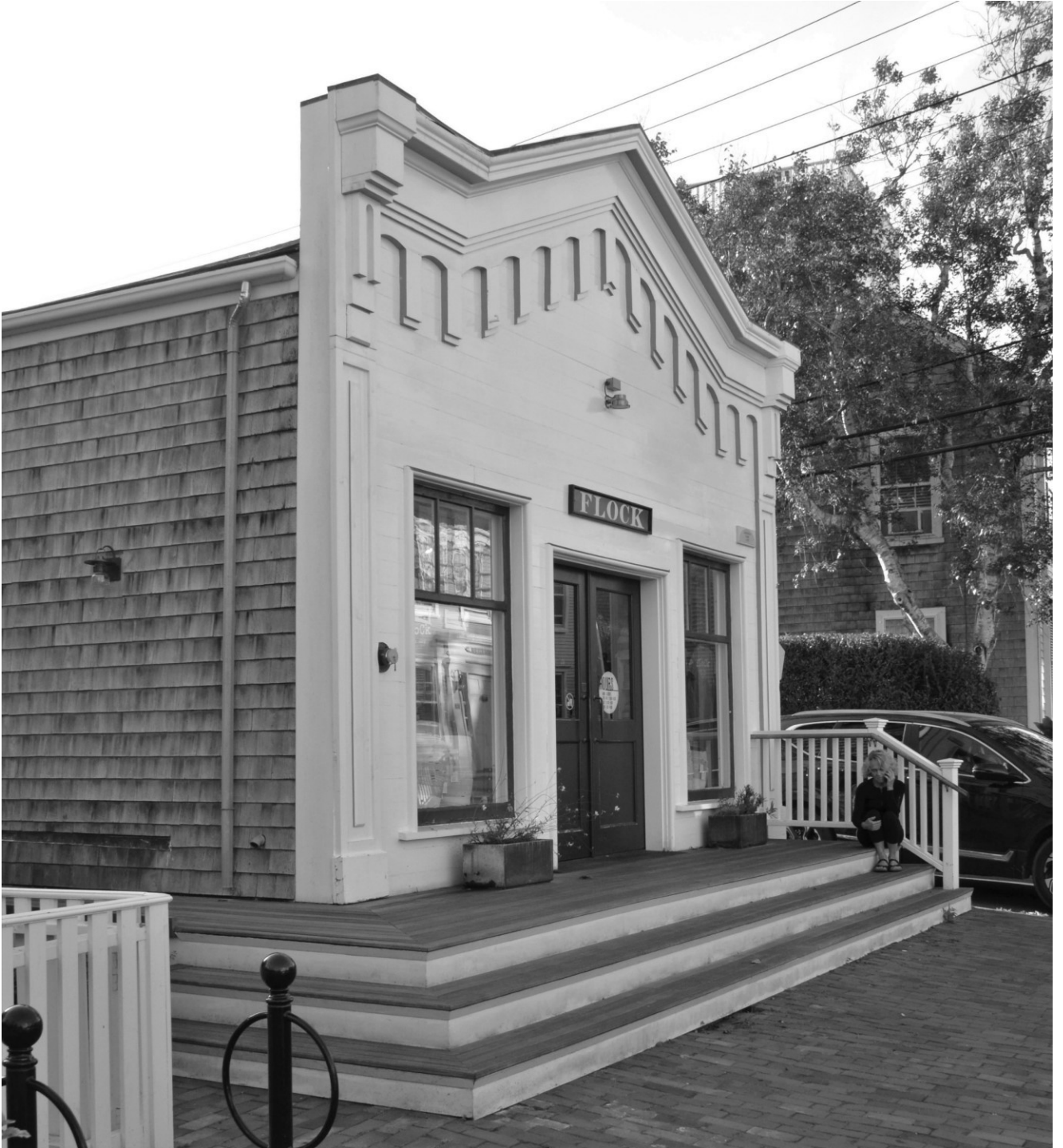
Photo #1 – façade (east elevation)
