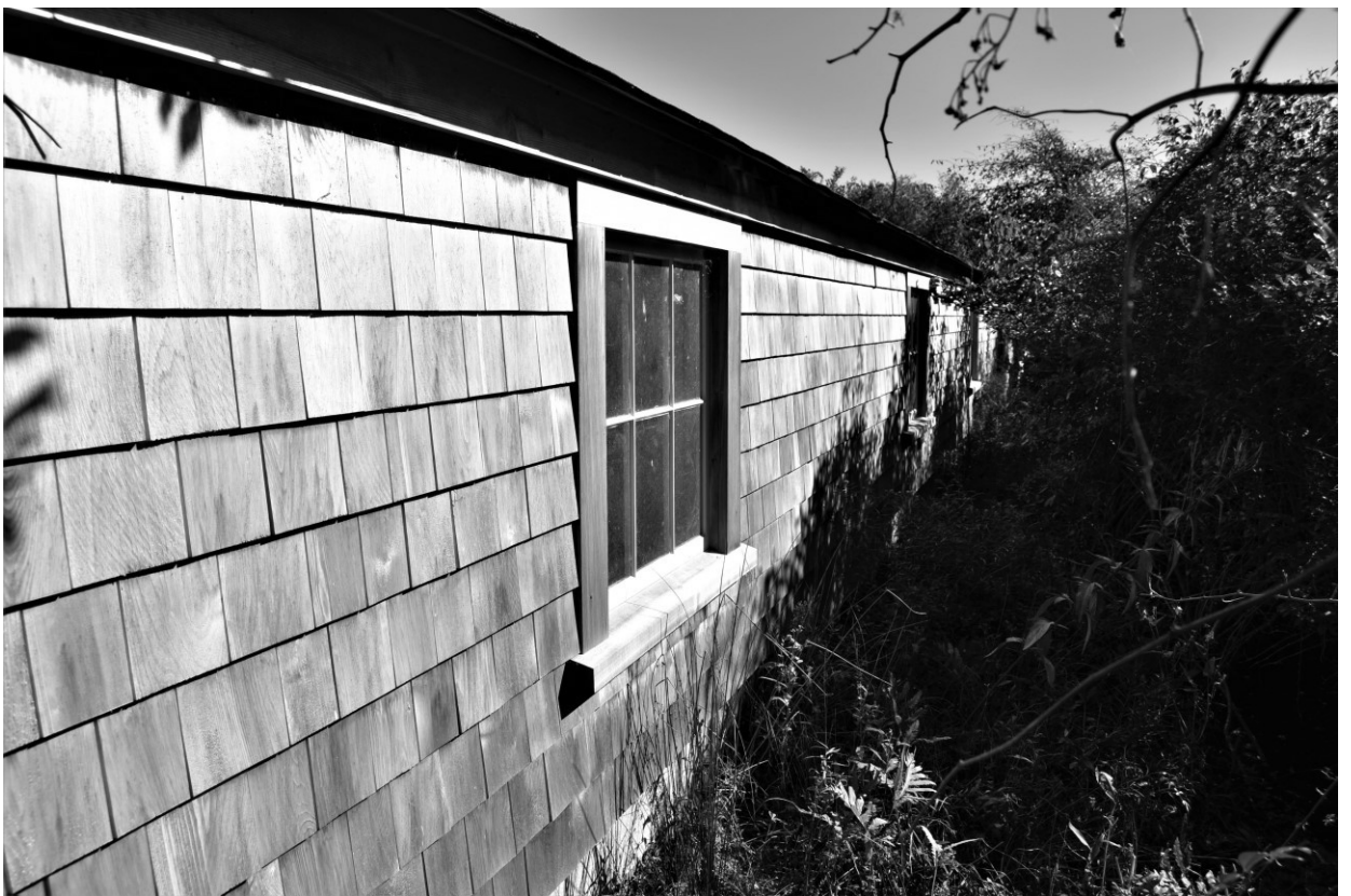
Photo #25 – Long Shed – south elevation viewed from west end looking eastward
