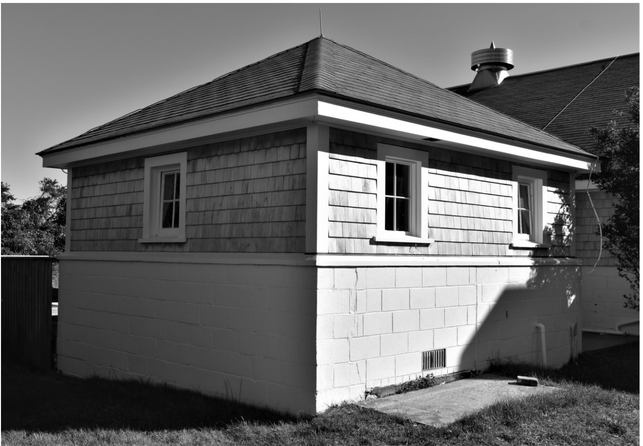
Photo #12 – Barn - west & south elevations of the Milk House
