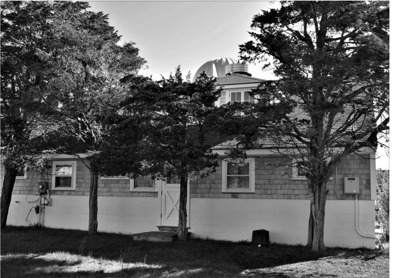
Photo #16 – Barn – west elevation (south end) with dome of West Silo photo background)
