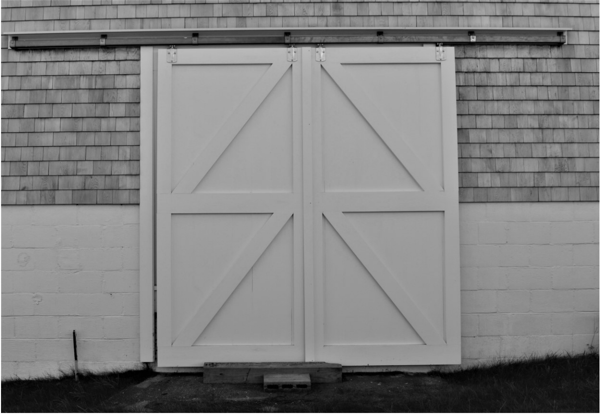
Photo #8 – north elevation – barn door – center doorway
