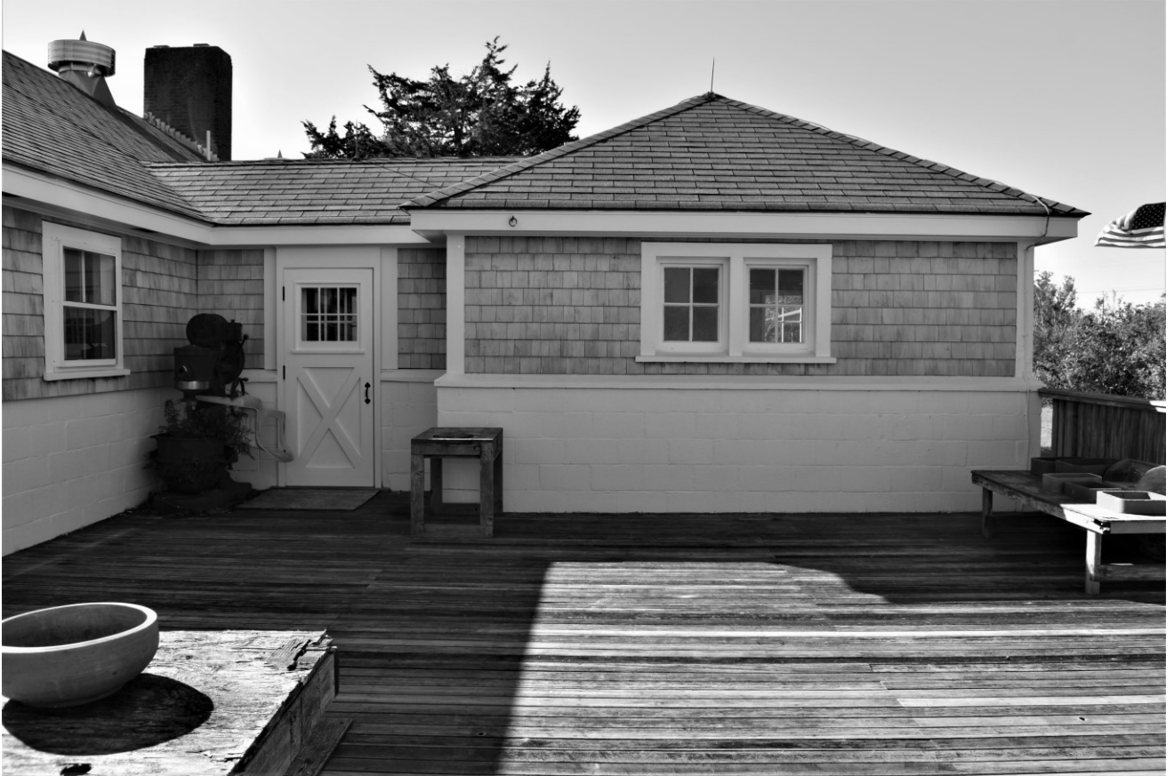
Photo #11 – Barn - north façade of connector & Milk House
