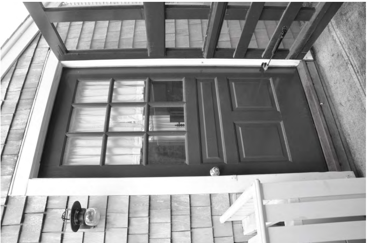
Photo #8 – west elevation - entry
