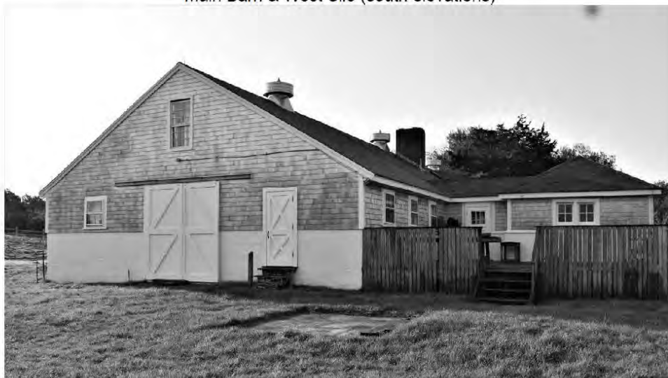
Main Barn & Milk Room (north & west elevations)
