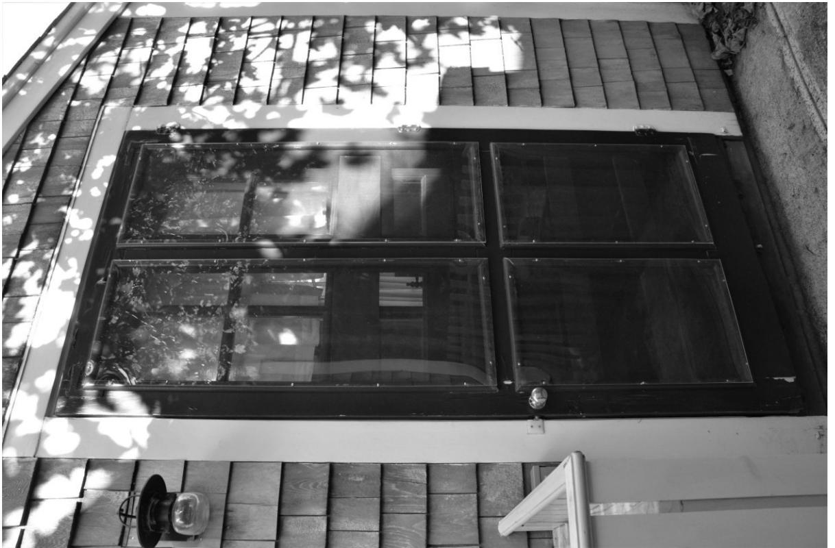
Photo #7– west elevation – entry with screen door closed
