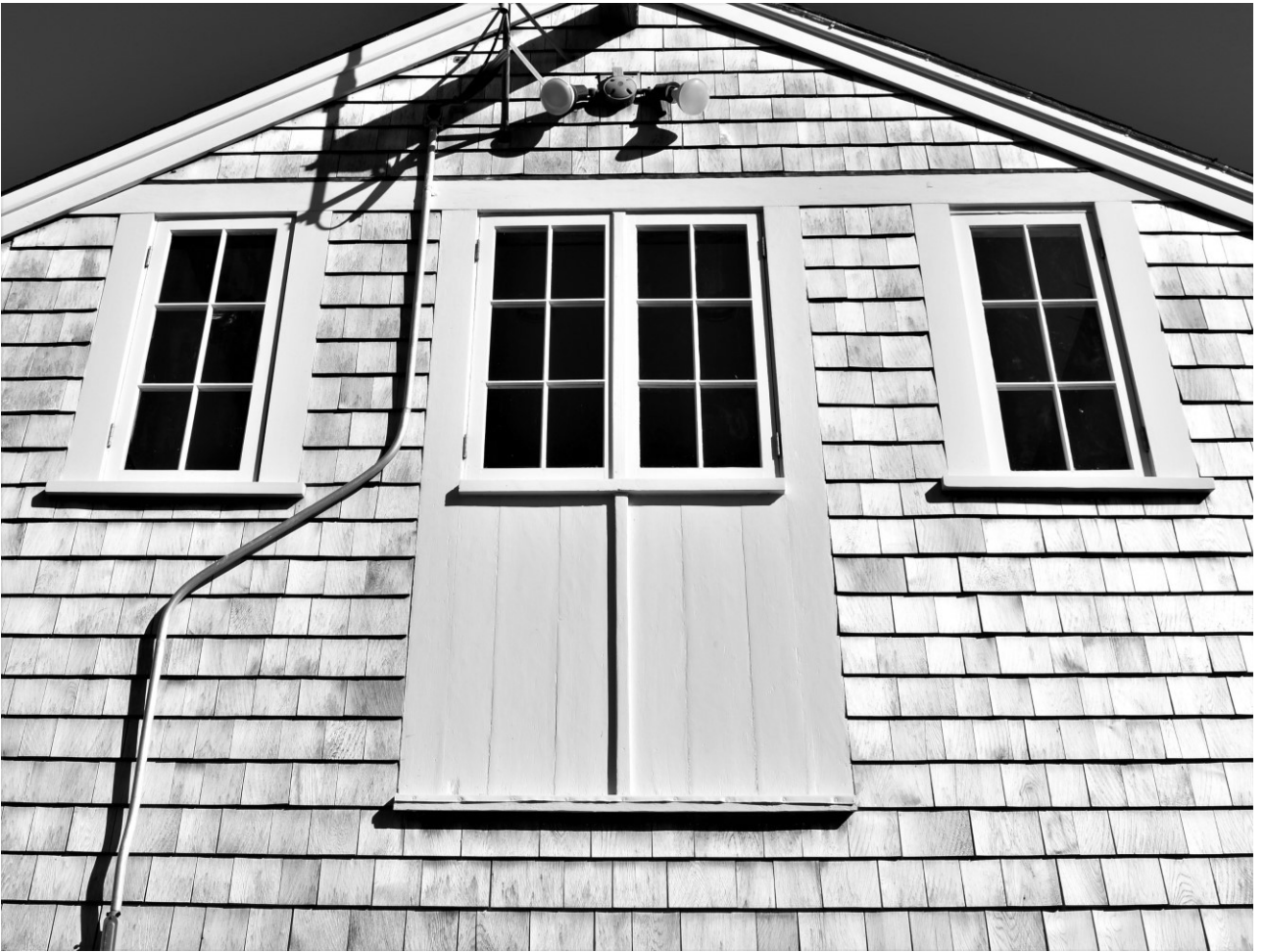
Photo #3 – south elevation of Barn – detail of gable windows & door
