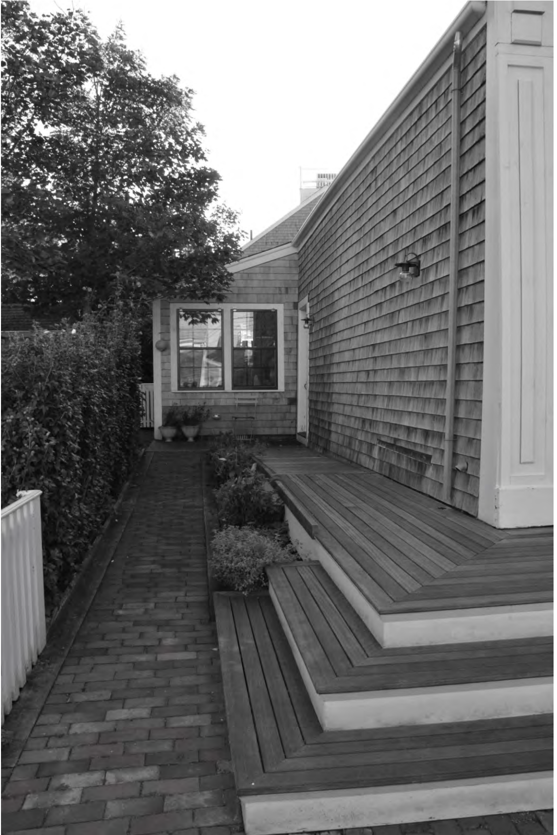
Photo #11 – south elevation and partial east elevation (photo left)
