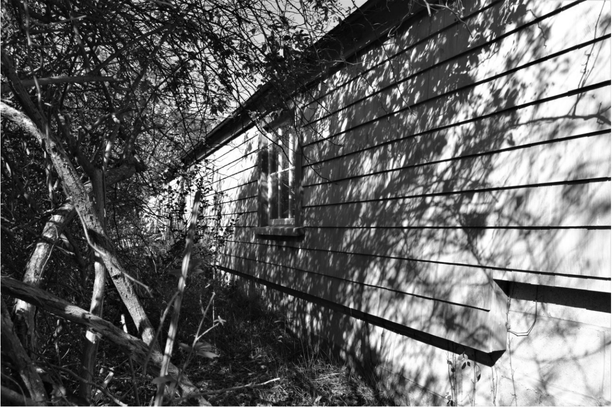
Photo #24 – Long Shed – south elevation – viewed from east end looking westward
