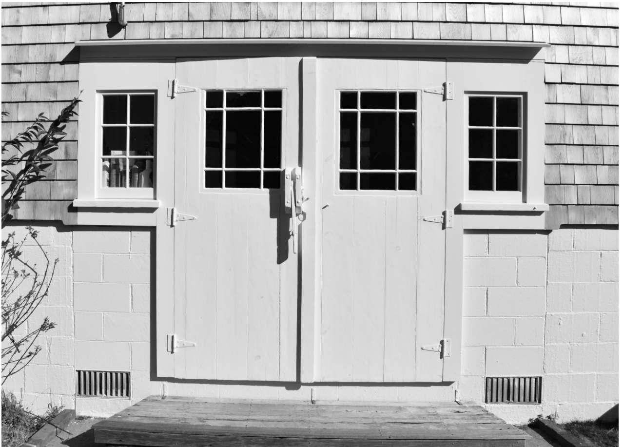
Photo #2 – south elevation of the Barn – detail of entry
