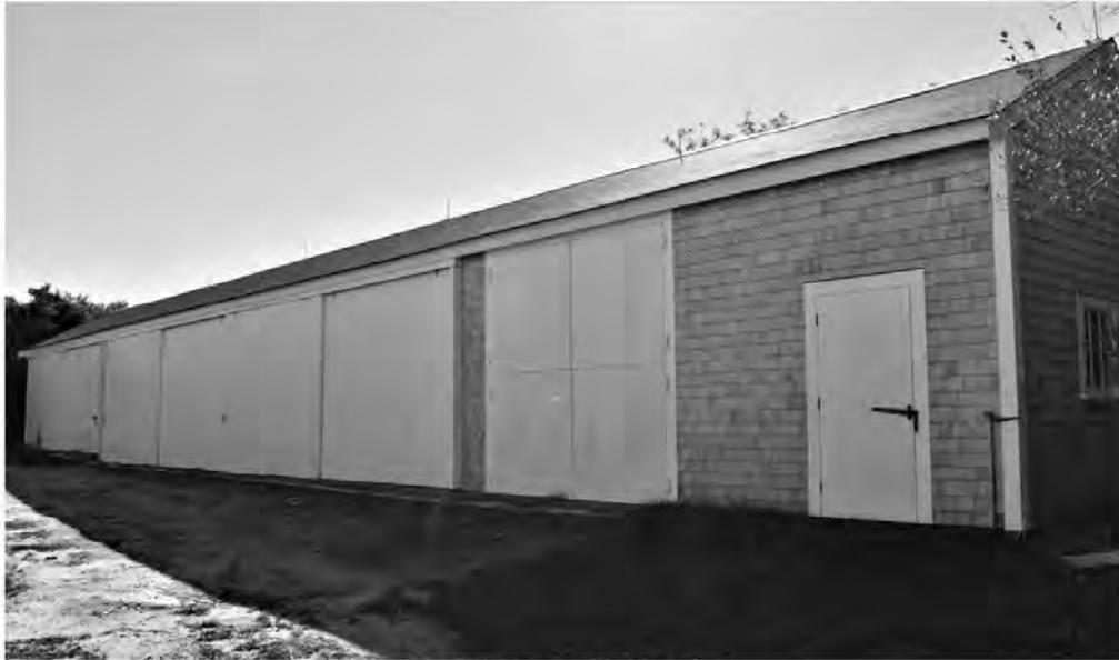
Long Shed – north elevation
