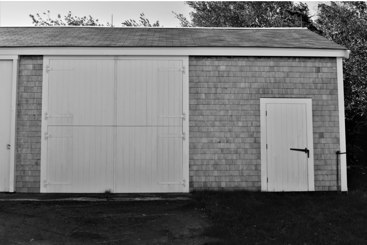
Photo #20 – Long Shed – north elevation showing typical finishes at western bays
