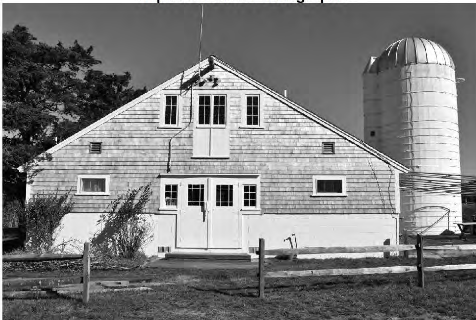
Main Barn & West Silo (south elevations)
