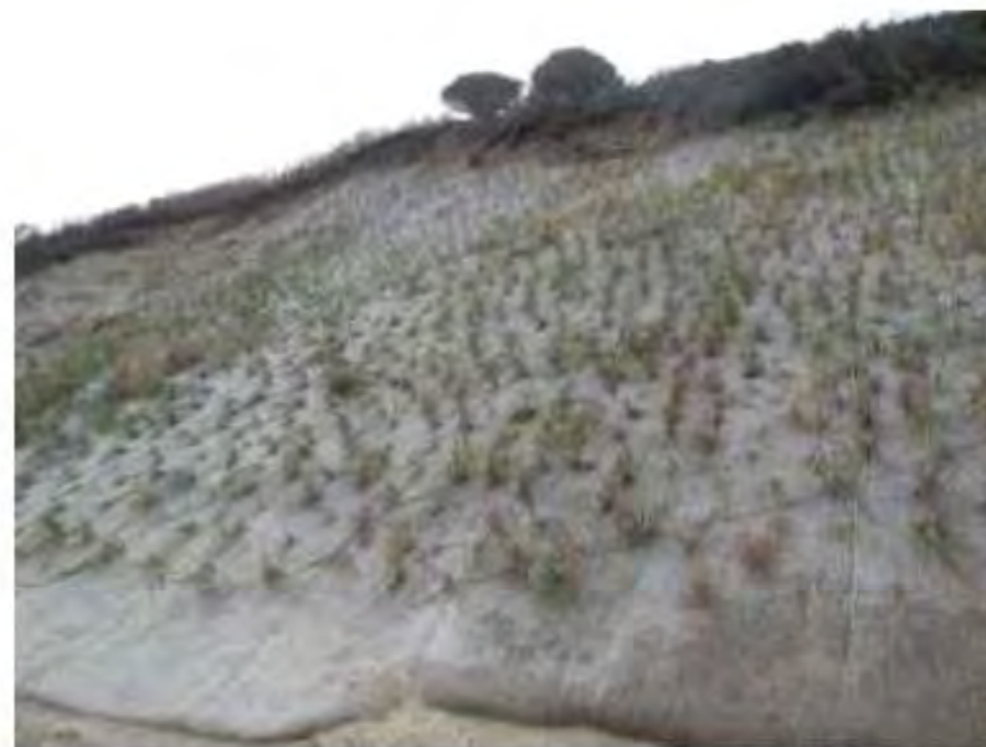
Beach Grass with Jute Mesh, Sicaonset Bluff, Nantucket (WPI, 2014)
