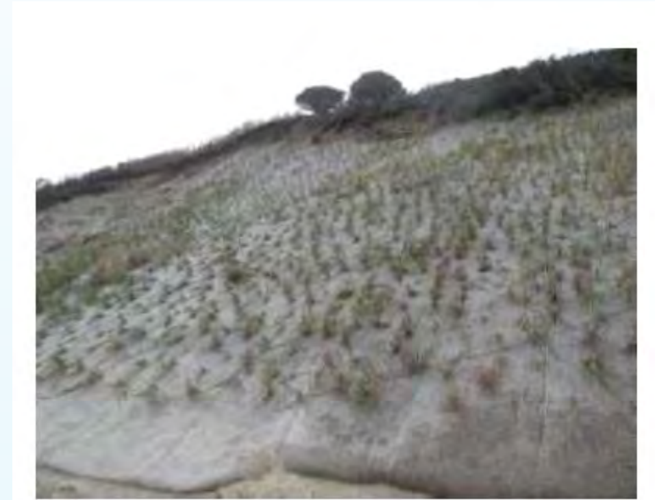
Beach Grass with Jute Mesh, Sicaonset Bluff, Nantucket (WPI, 2014)
