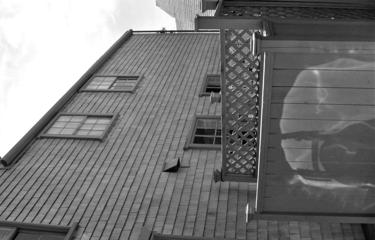
Photo #6 – north elevation of Rear Ell
