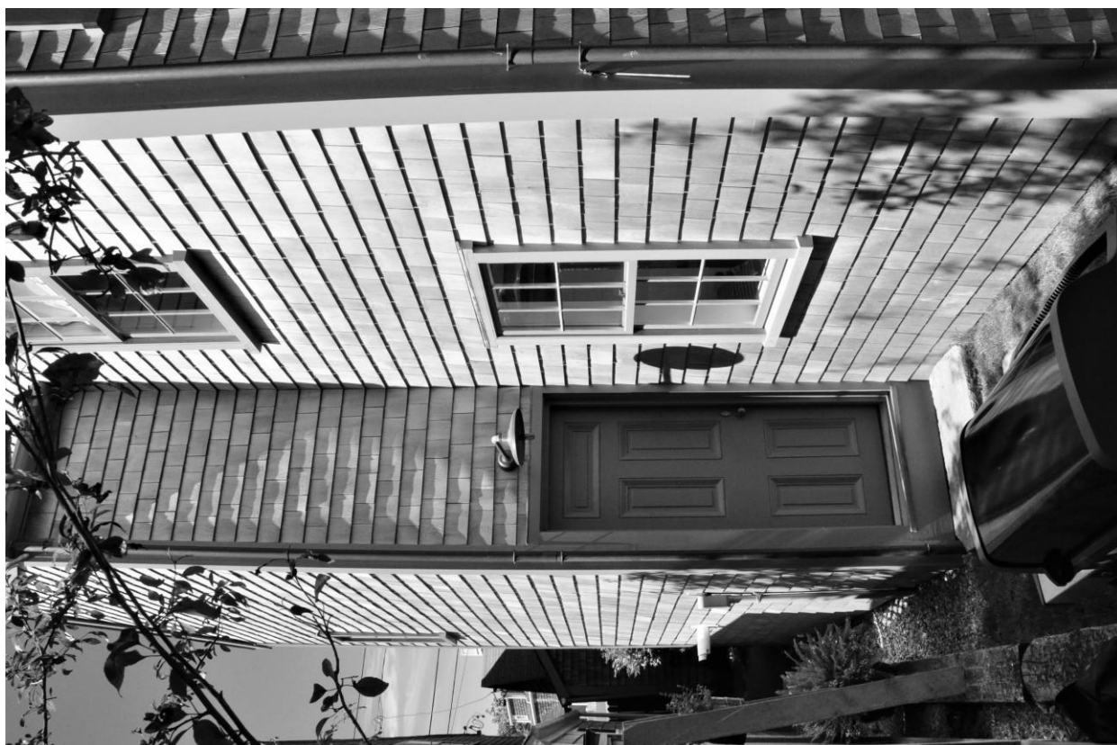
Photo #5 – west elevation of Rear Ell
