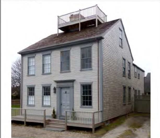
façade (east elevation)
