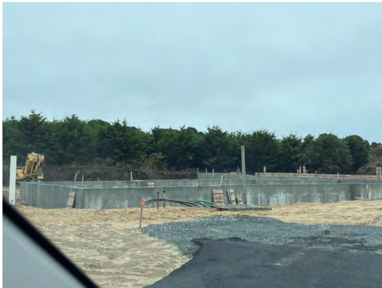
Photo of new foundation in front of new building at Richmond at the current terminus of Harvey Road.
