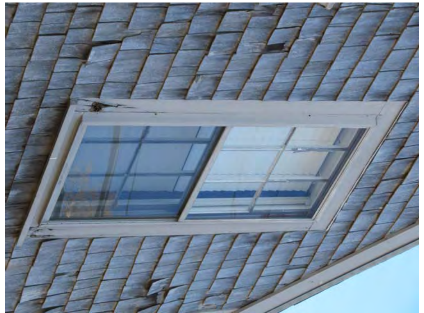
2. Main House, east elevation, second floor, typical six-over-six wood window
