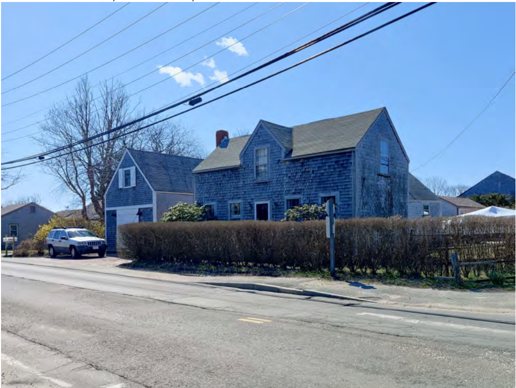
2. 5 Surfside Road, Main House (right) and Cottage (left), view southwest
