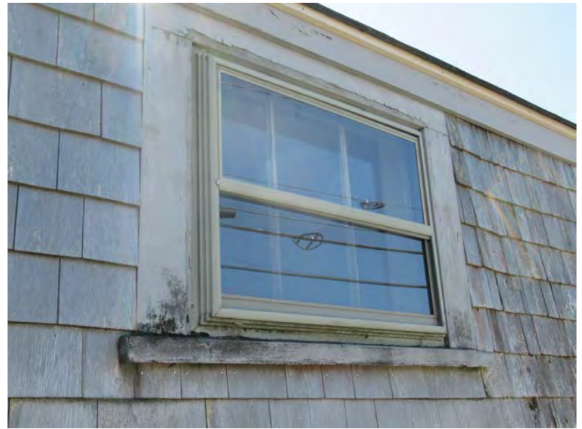
22. North elevation of first ell, window detail, view southwest
