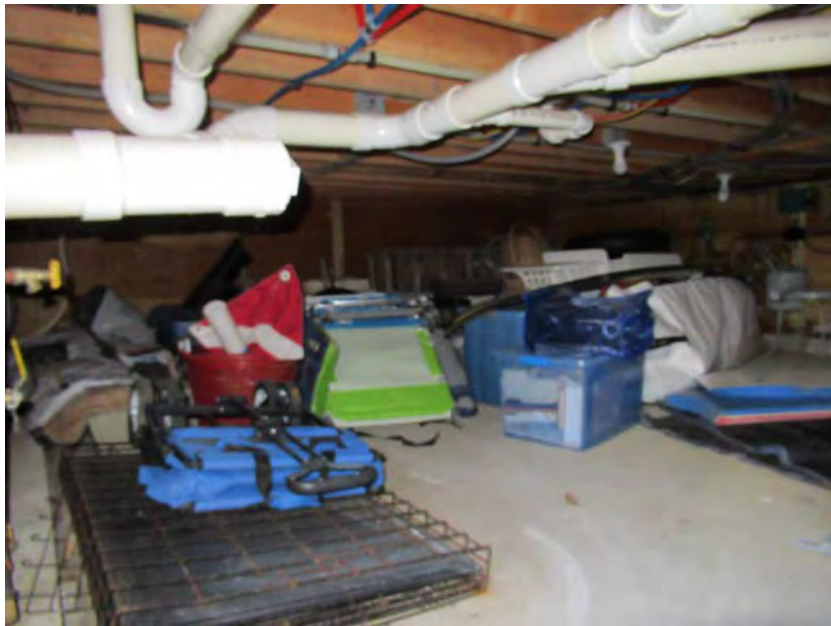
11. Cottage, crawl space, view southeast
