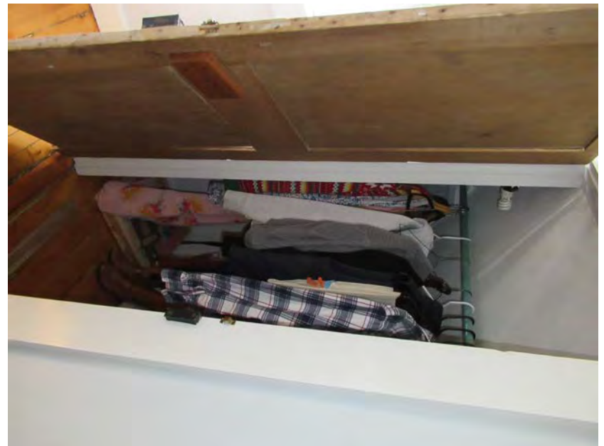
62. Second floor, bedroom closet, view southwest
