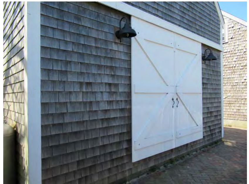
2. Cottage, east elevation detail, view northwest
