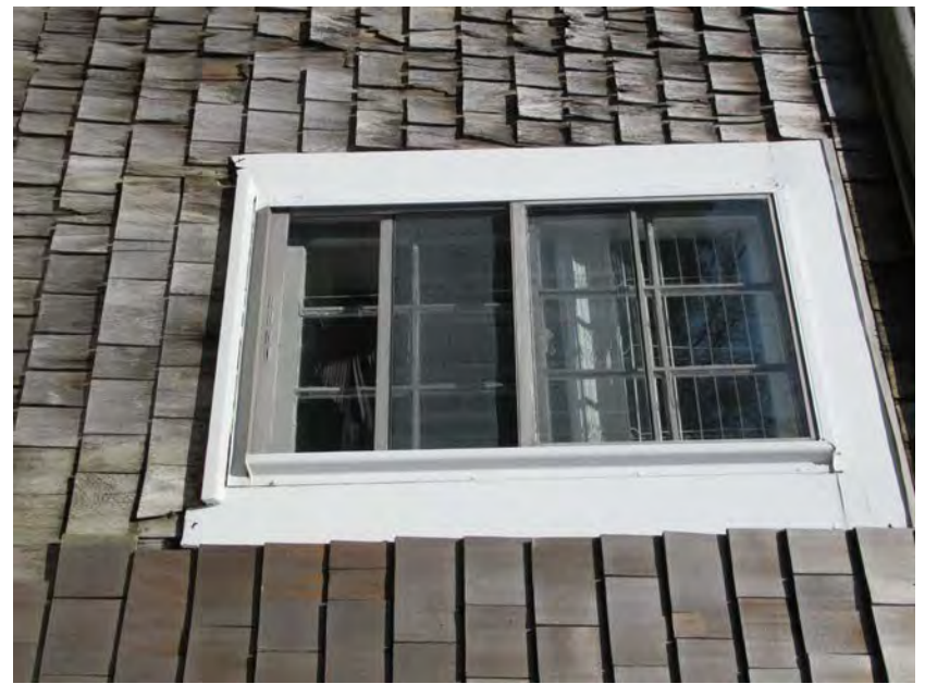
6. Main House, ell, south elevation, typical six-over-six wood window
