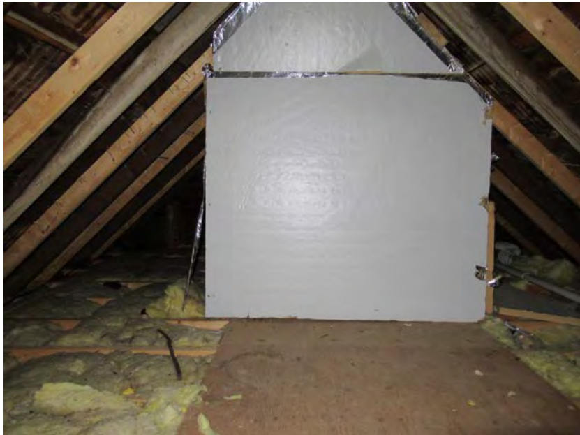
67. Second floor, utility room, view east
