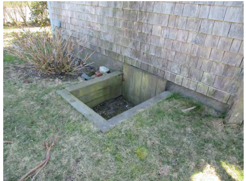
26. North elevation, crawlspace access, view southeast
