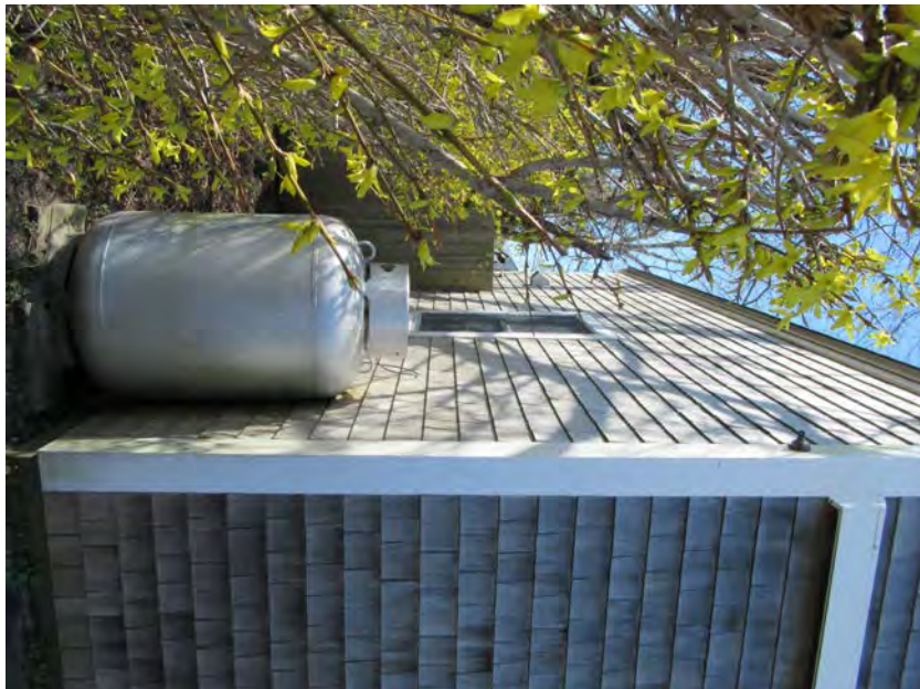
3. Cottage, south elevation, view northwest
