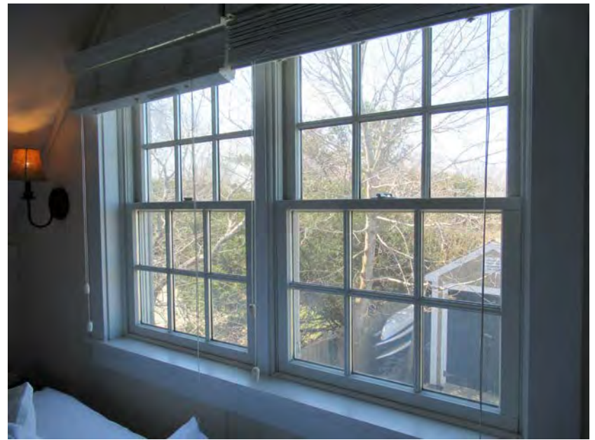
26. Cottage, second floor, window detail, view southwest
