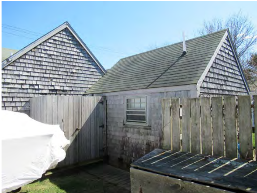
19. West elevation of first ell (far left), north (left) and west (right) elevations of second ell, view southeast
