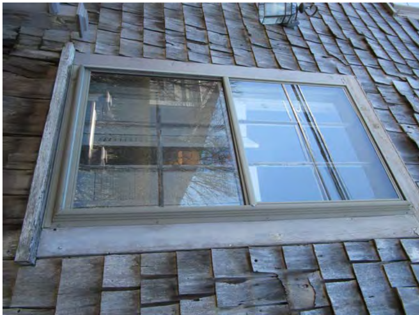
1. Main House, east elevation, first floor, typical six-over-six wood window
