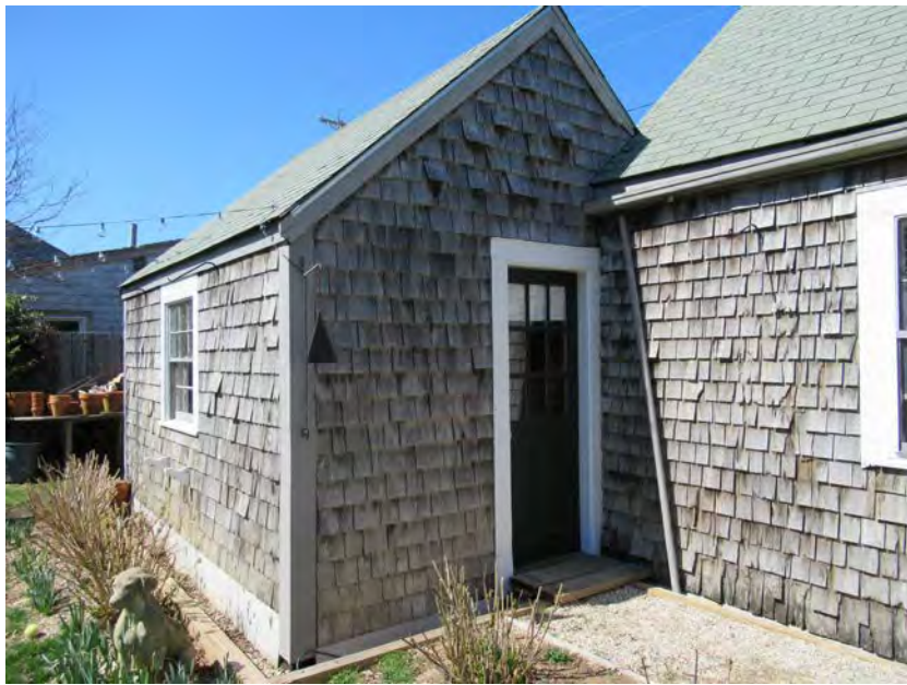
13. South elevation (left) and east elevation (right) of second ell, view northwest
