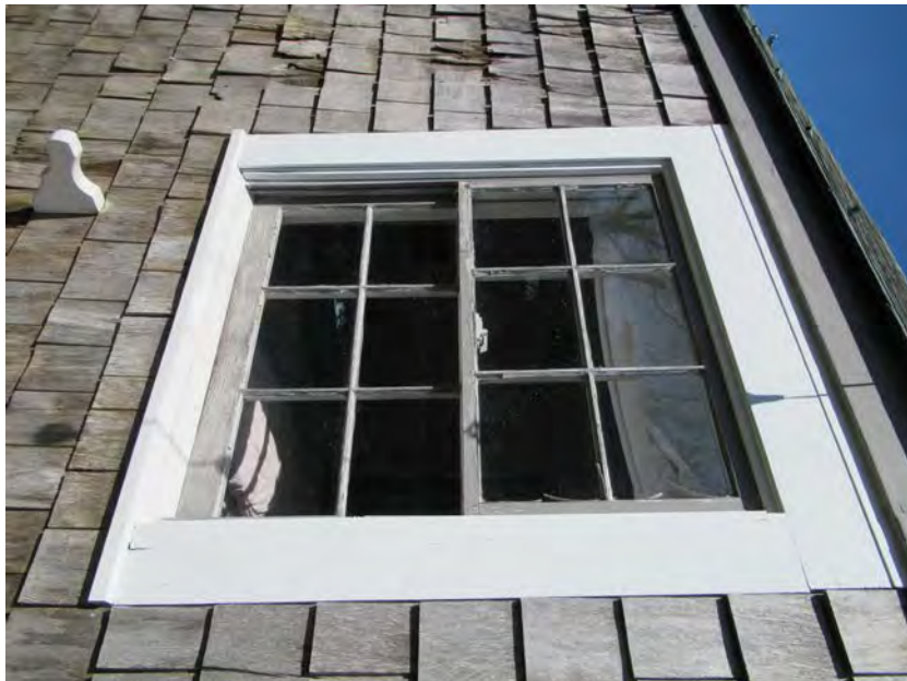
15. South elevation, second ell, window detail, view northwest
