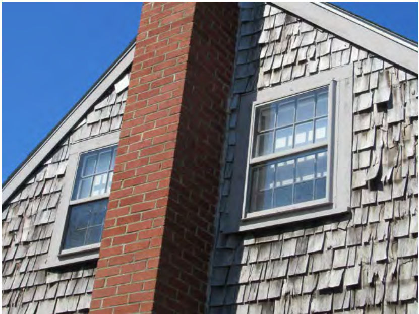
7. Main House, south elevation, second floor, eight-over-eight wood window
