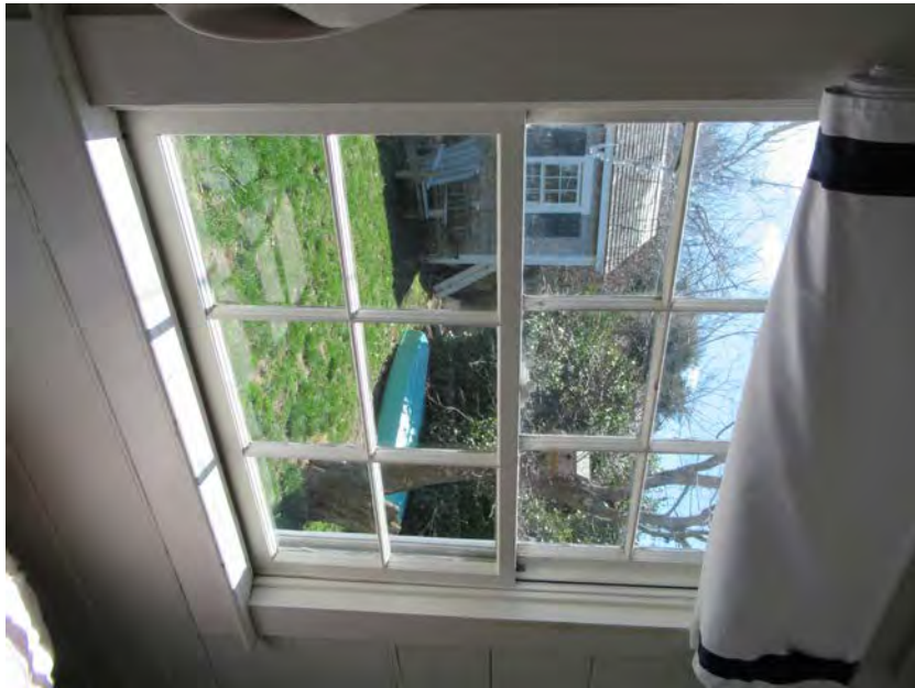
47. First floor, bedroom, window detail, view southwest
