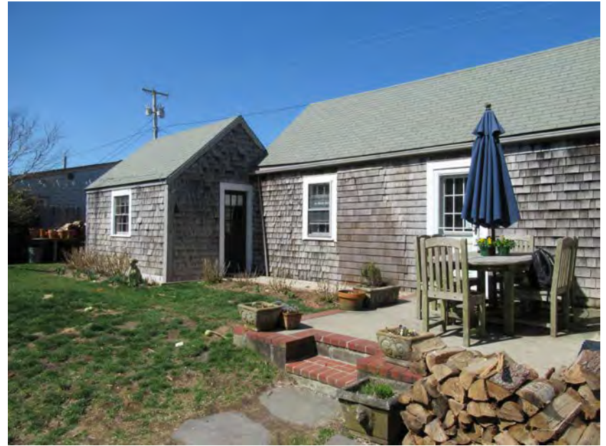
10. South elevation, view northwest
