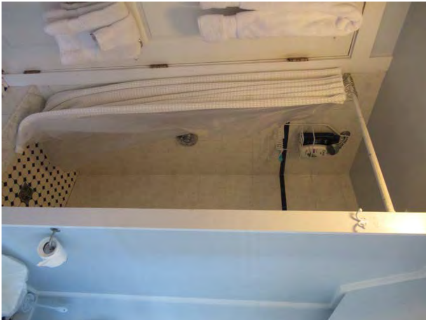
59. Second floor, bathroom, view northwest
