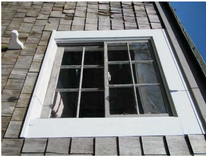
5. Main House, ell, south elevation, typical six-over-six wood window
