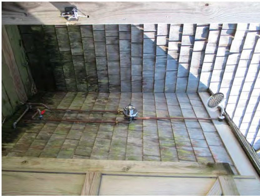
21. West elevation of first ell, outdoor shower detail, view southeast
