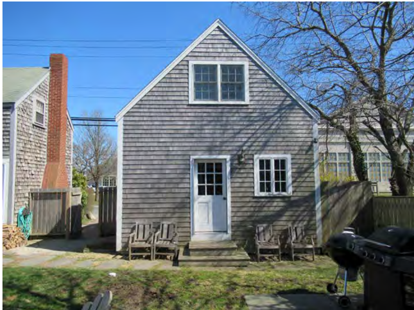
7. Cottage, west elevation, view east
