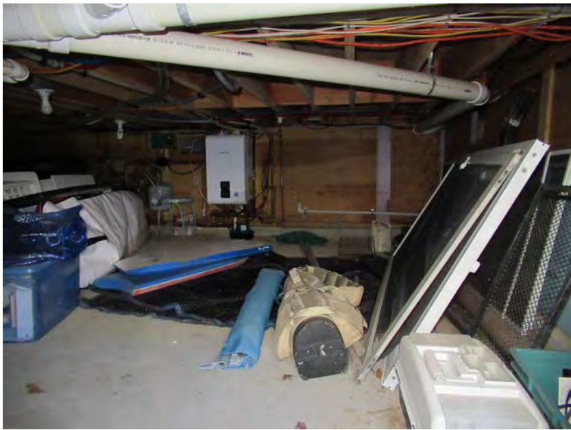
10. Cottage, crawl space, view south
