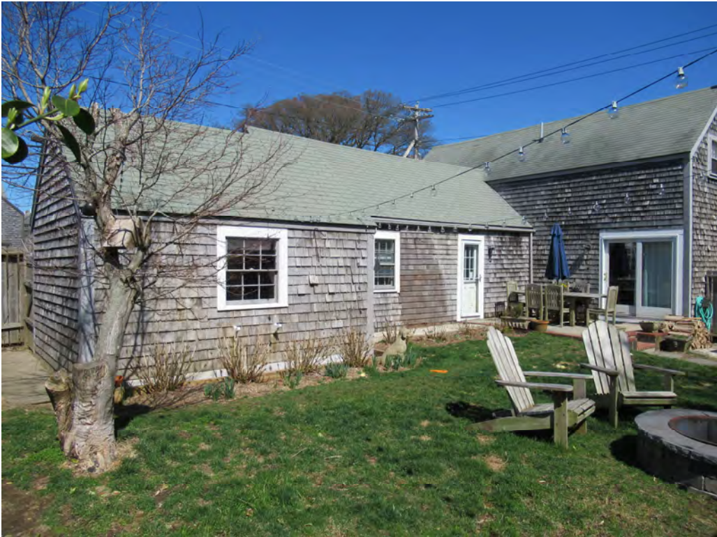
4. 5 Surfside Road, Main House, view northeast
