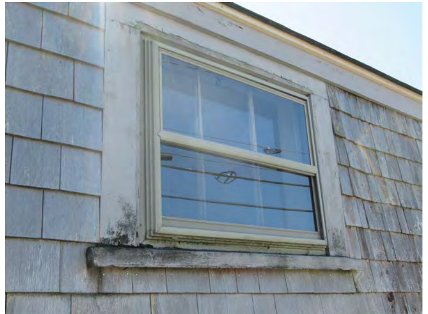
4. Main House, ell, north elevation, typical three-over-three wood window
