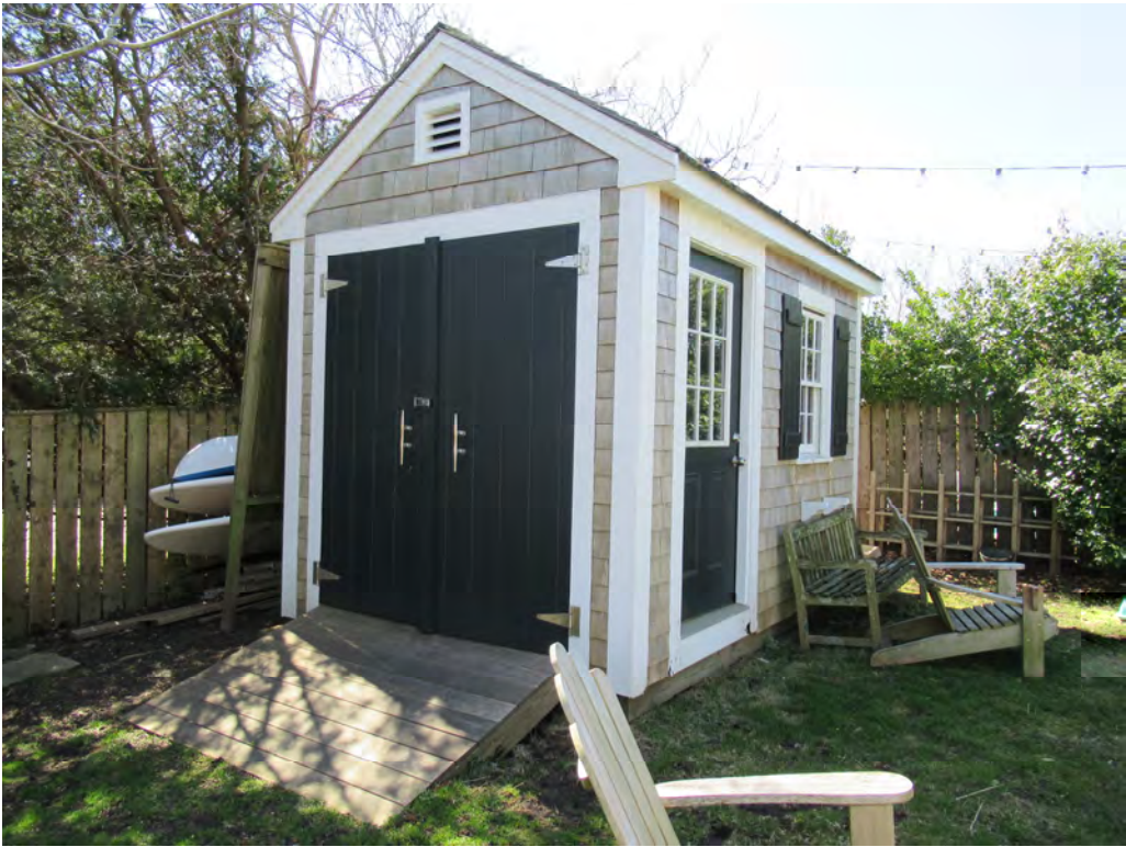
9. 5 Surfside Road, Shed, view southwest
