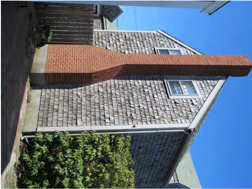
8. South elevation, view northwest
