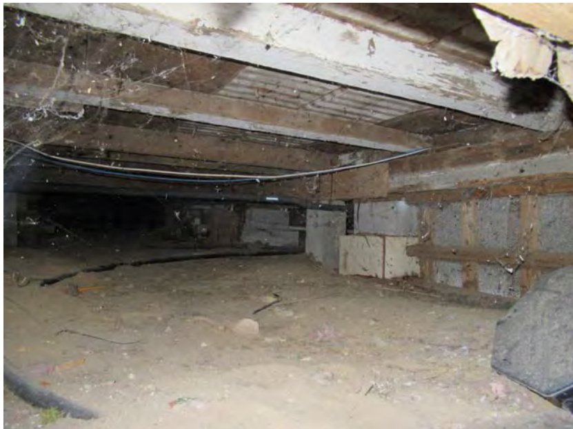
27. Crawl space, view southwest
