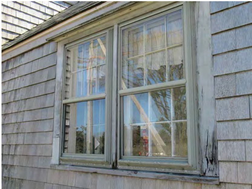
3. Main House, ell, north elevation, typical six-over-six wood windows
