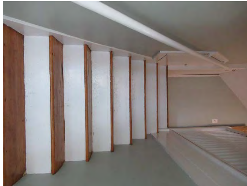
50. First floor, main stair, view north
