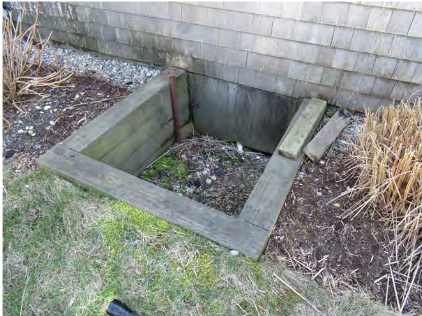
23. West elevation of first ell, crawlspace access, view southeast
