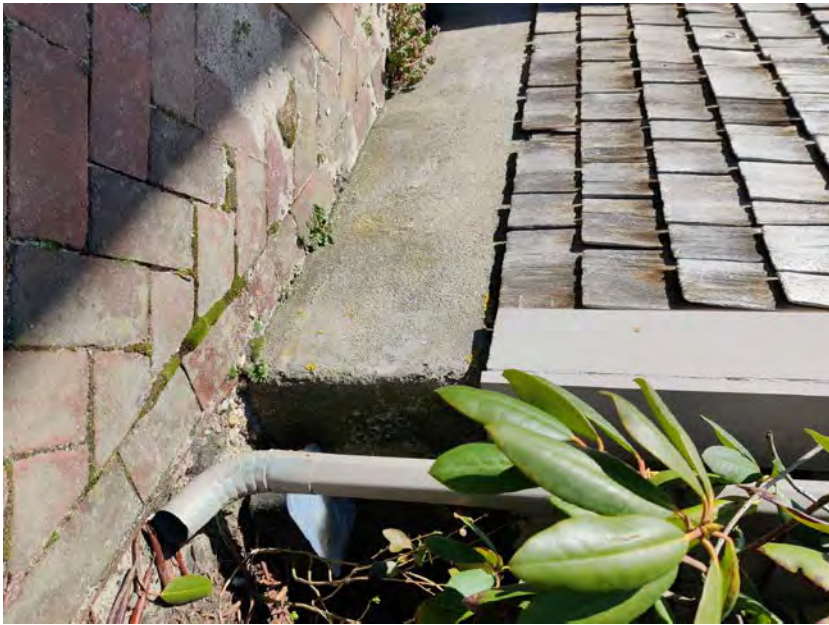
9. South elevation, foundation detail, view northwest
