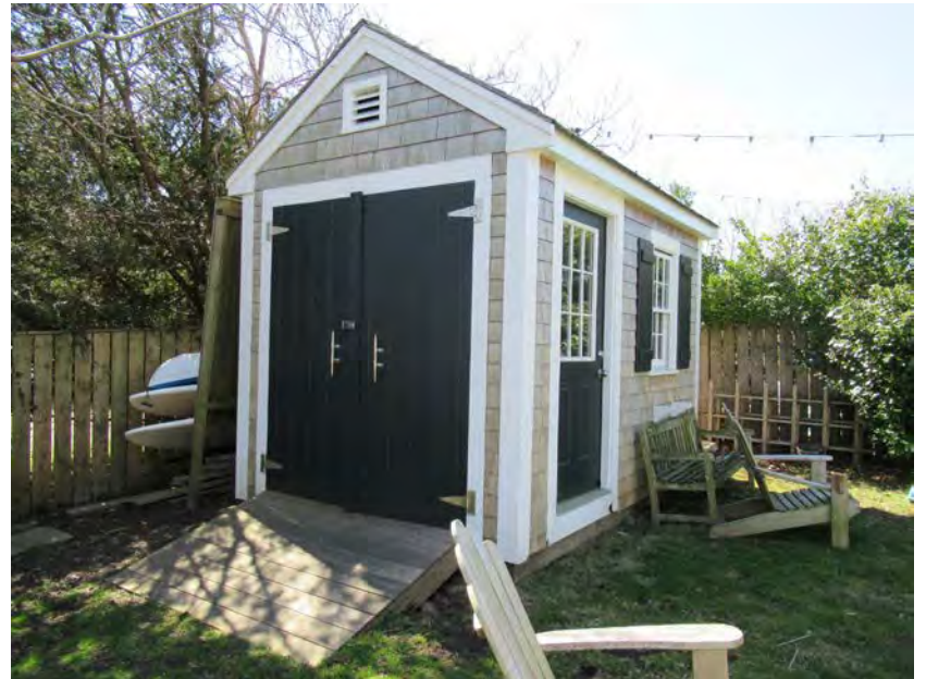
16. Shed, view southeast
