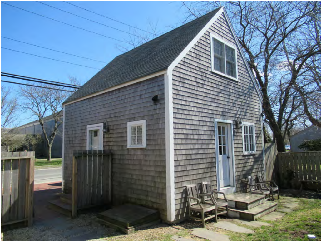
8. 5 Surfside Road, Cottage, view southeast
