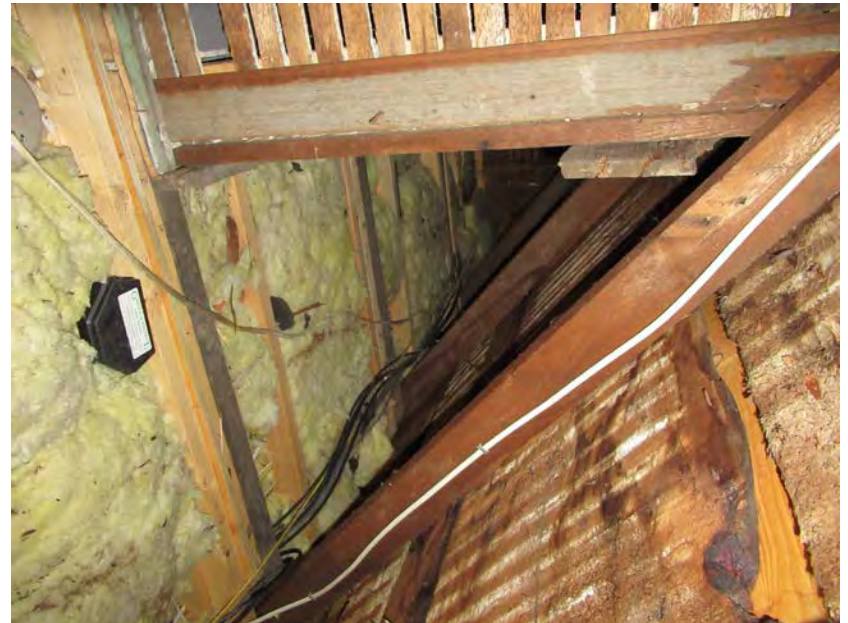
68. Second floor, utility room, view southeast
