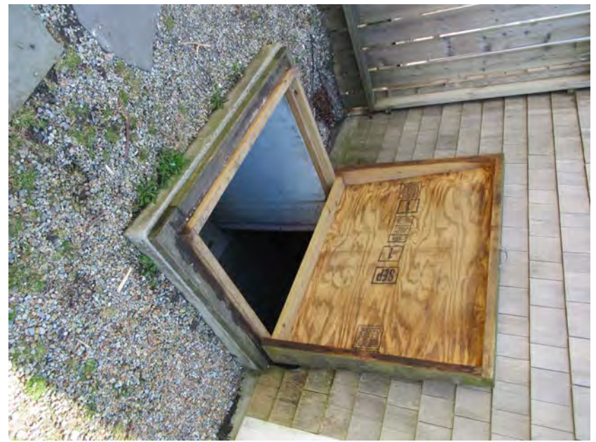
6. Cottage, north elevation, crawlspace access detail, view southeast
