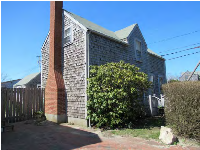
4. South elevation (left) and east elevation (right), view northwest
