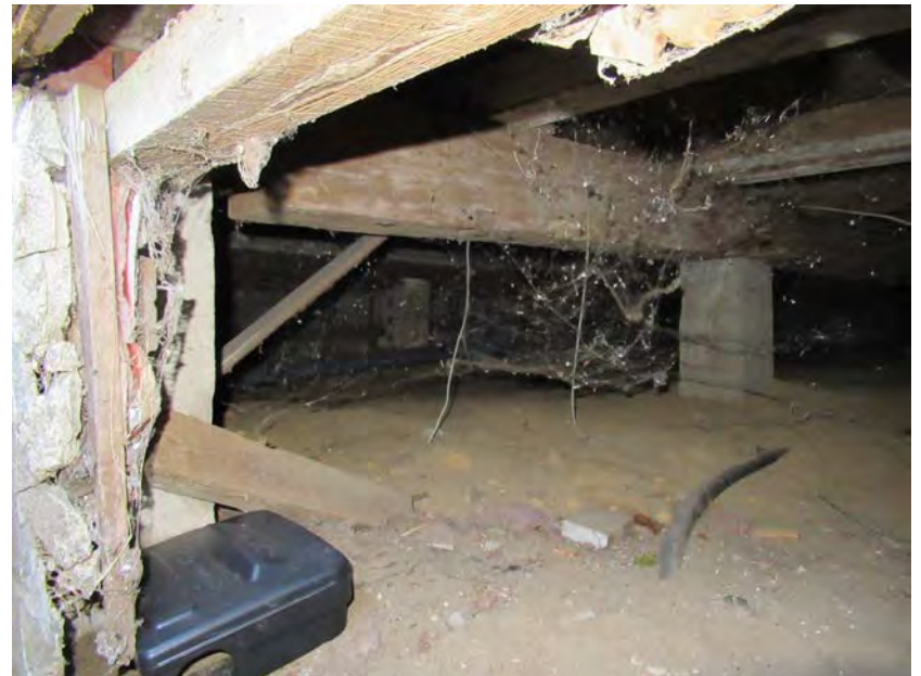
28. Crawl space, view southeast
