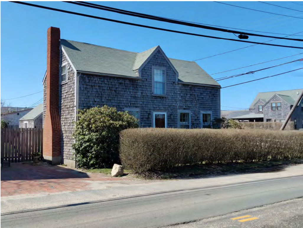
1. 5 Surfside Road, Main House, view northwest
