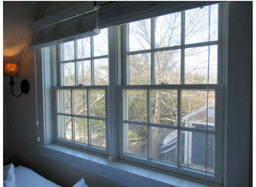
8. Cottage, second floor, typical six-over-six wood windows
