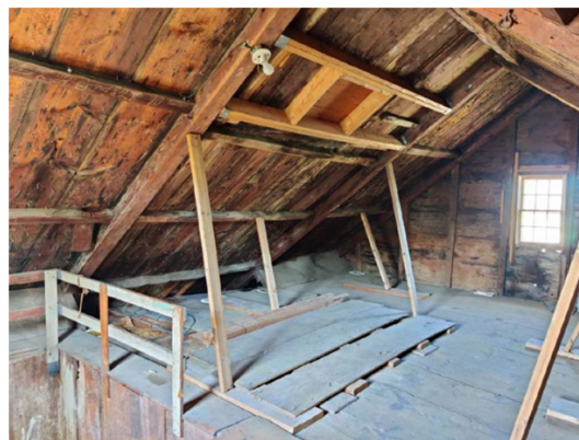
23. Attic, view northeast
