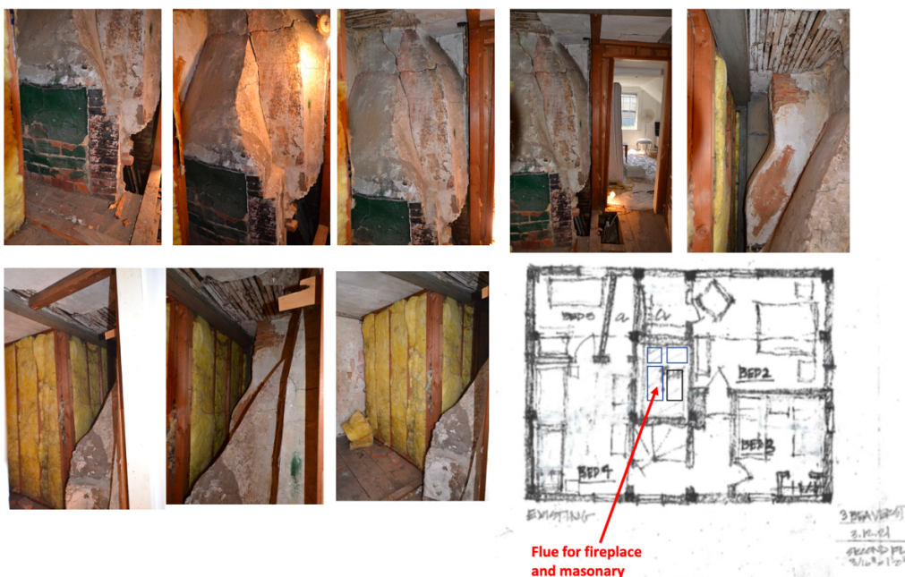
Chimney stack at second floor, documented in 2021 (under previous owner)
