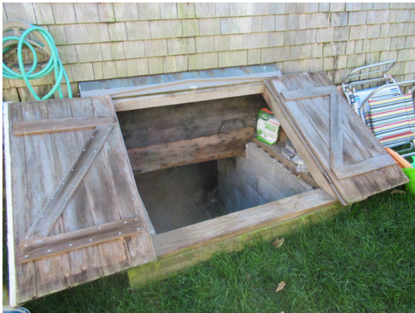
17. North elevation, basement bulkhead, view southwest
