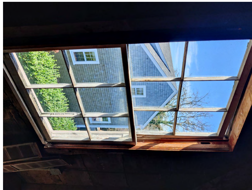
76. Attic, window detail, view northwest
