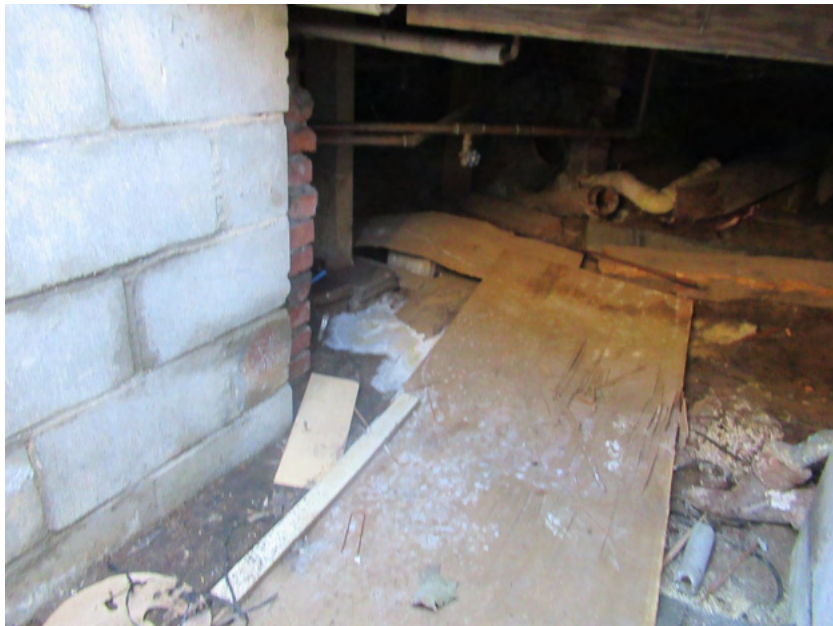
23. Crawl space, view southeast
