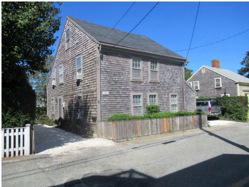
1. West elevation (left) and south elevation (right), view northeast
