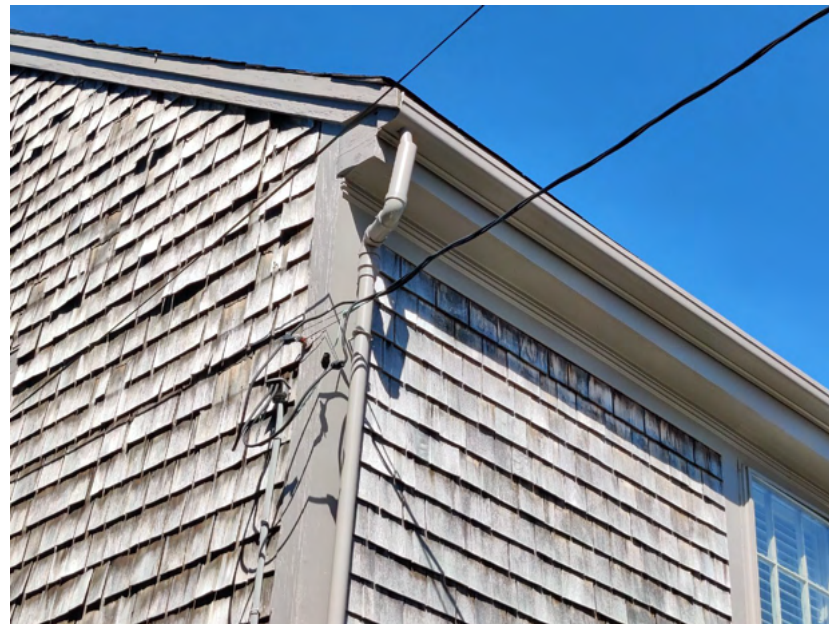
6. South elevation, cornice detail, view northeast
