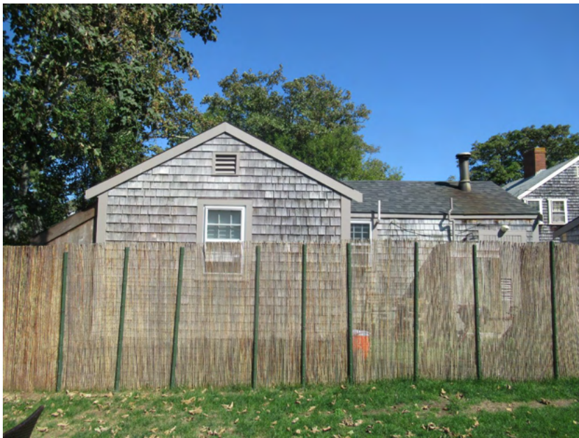
5. Cottage, west elevation (1975 addition at left), view east
