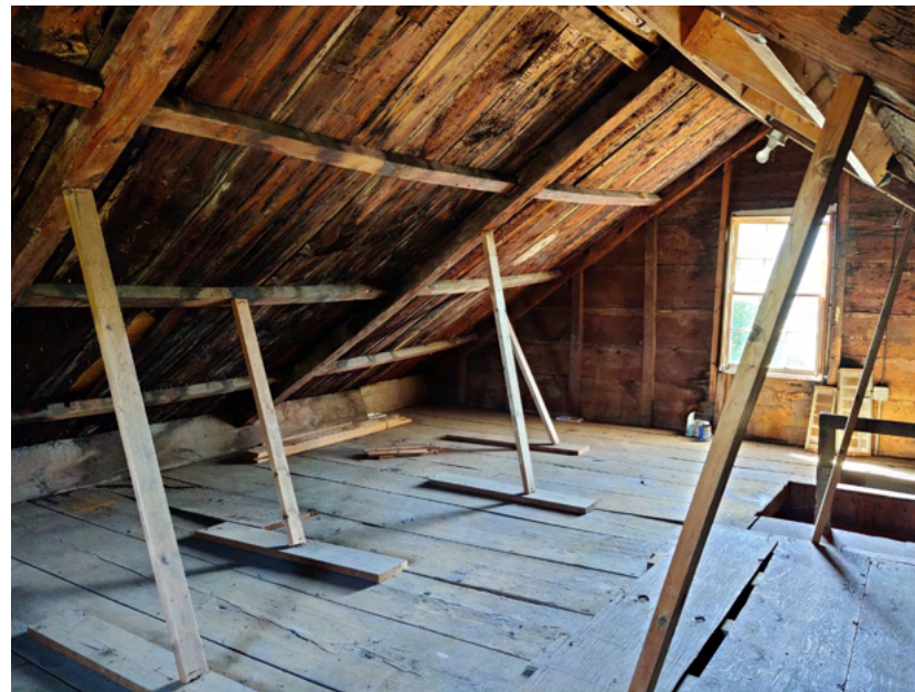
78. Attic, view southwest
