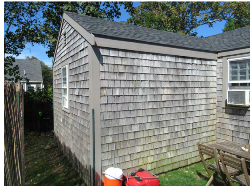
10. Cottage, 1975 addition, west elevation (left) and south elevation (right), view northeast
