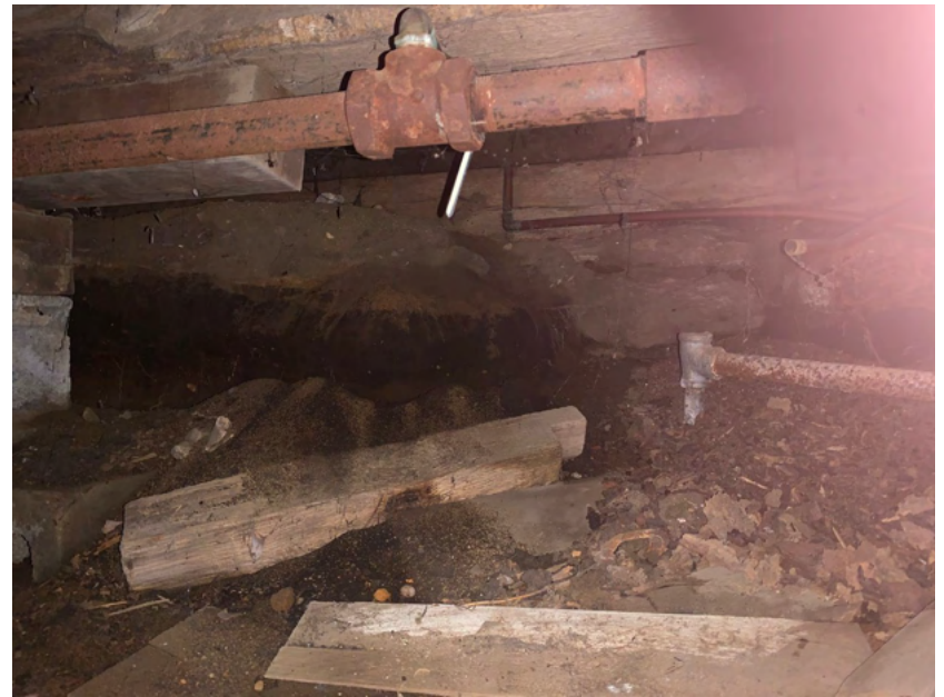
26. Crawl space, view east
