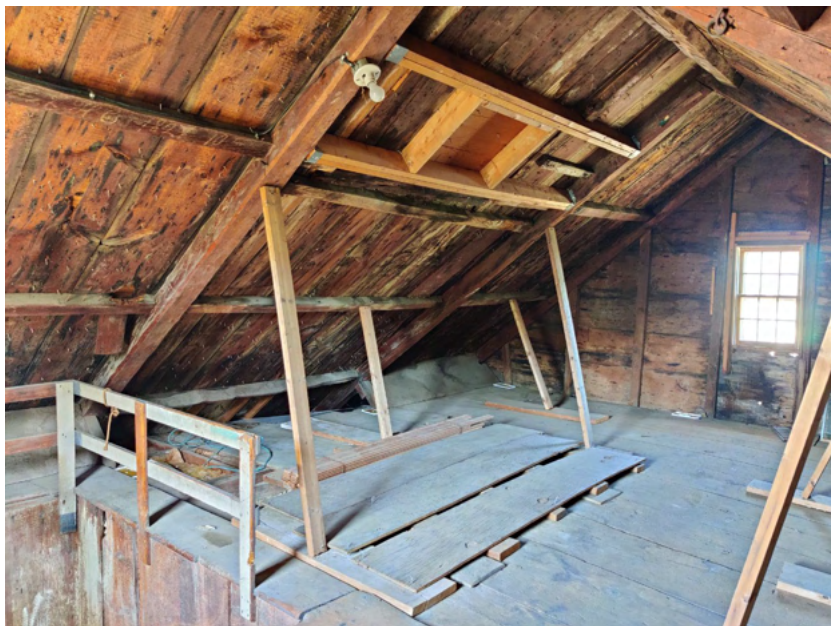
75. Attic, view northeast
