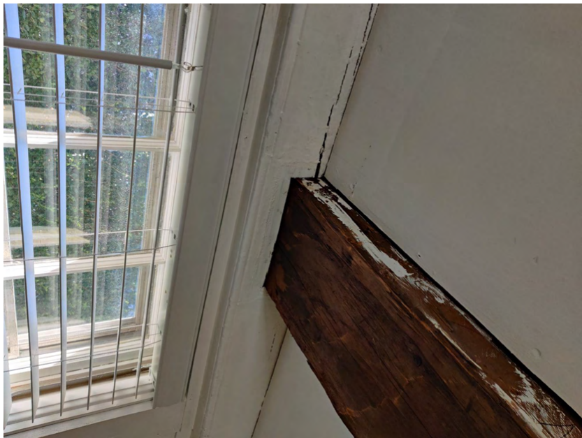
30. First floor, living room, beam detail, view west
