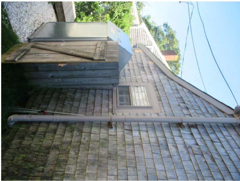
18. North elevation, east addition, view southeast
