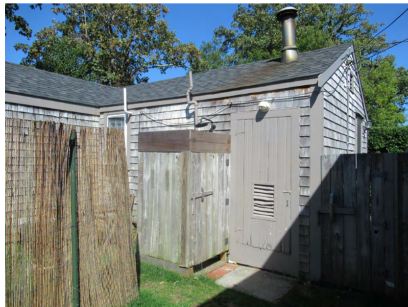
4. Cottage, west elevation (left) and south elevation (right), view northeast
