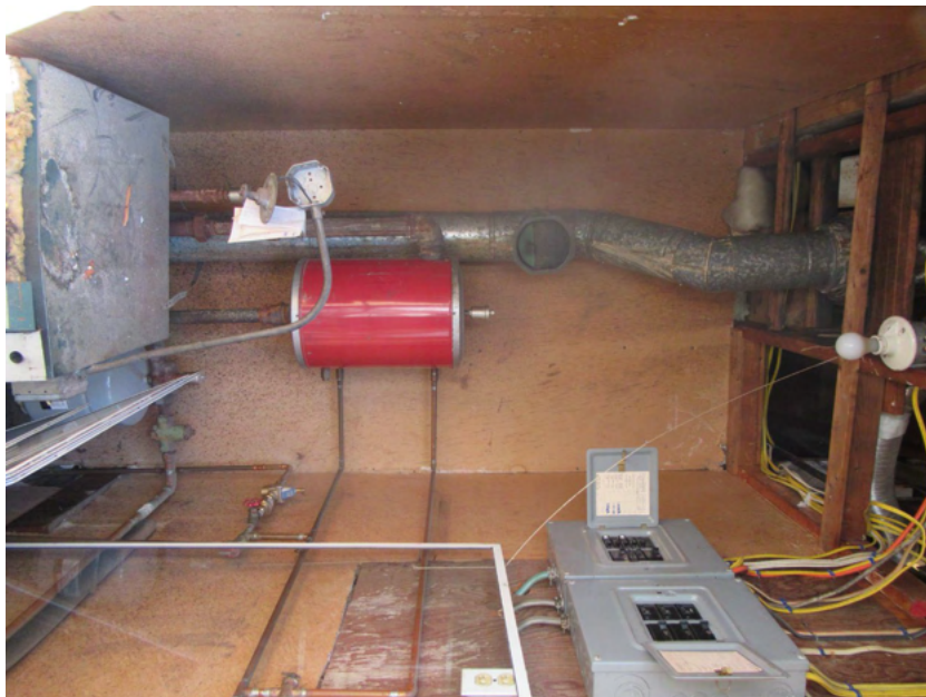
27. Utility room, view east
