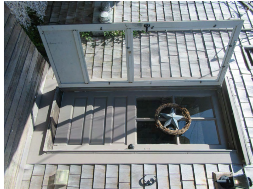
2. Cottage, south elevation, main entrance, view northwest
