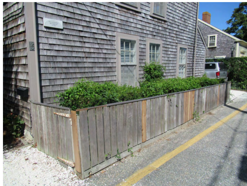
4. South elevation, front yard detail, view northeast
