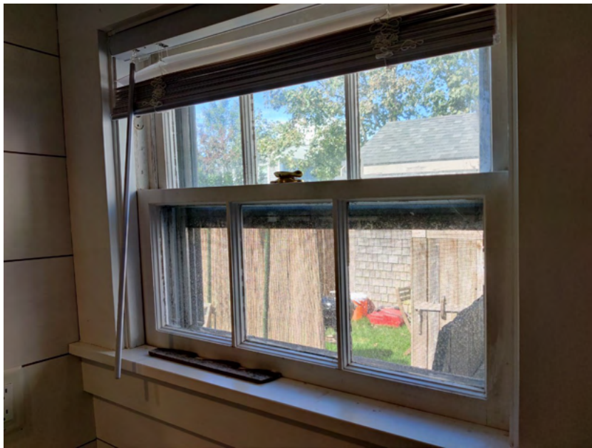
49. First floor, bathroom, window detail, view northwest
