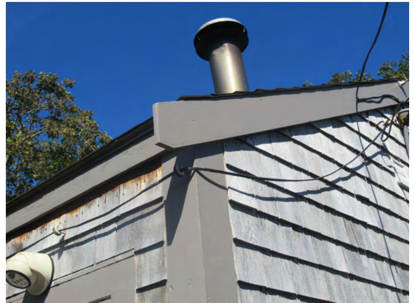
8. Cottage, rake trim detail, view northeast
