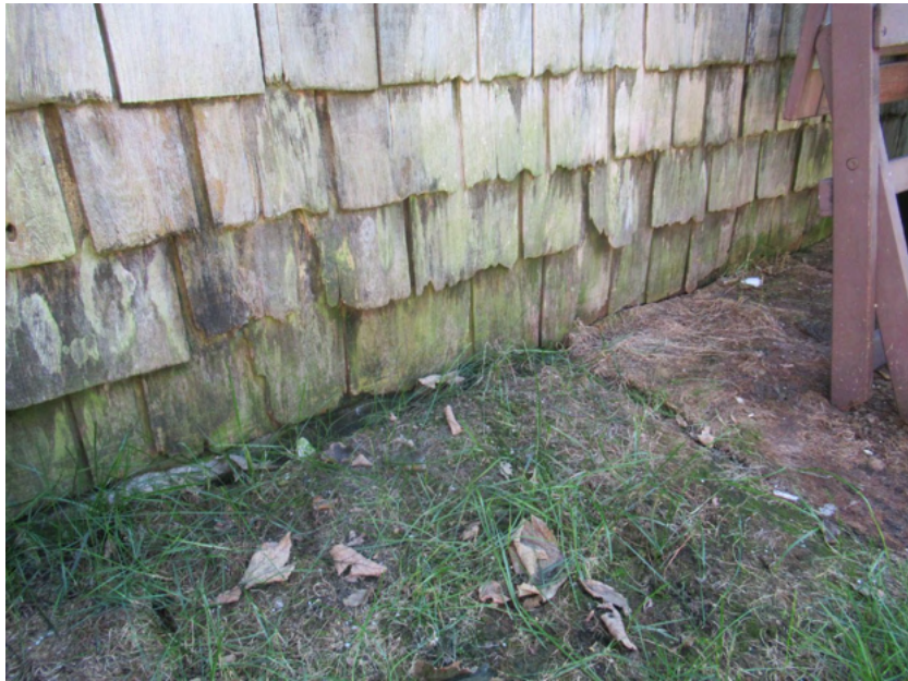
15. North elevation, shingle detail (typical conditions), view southwest
