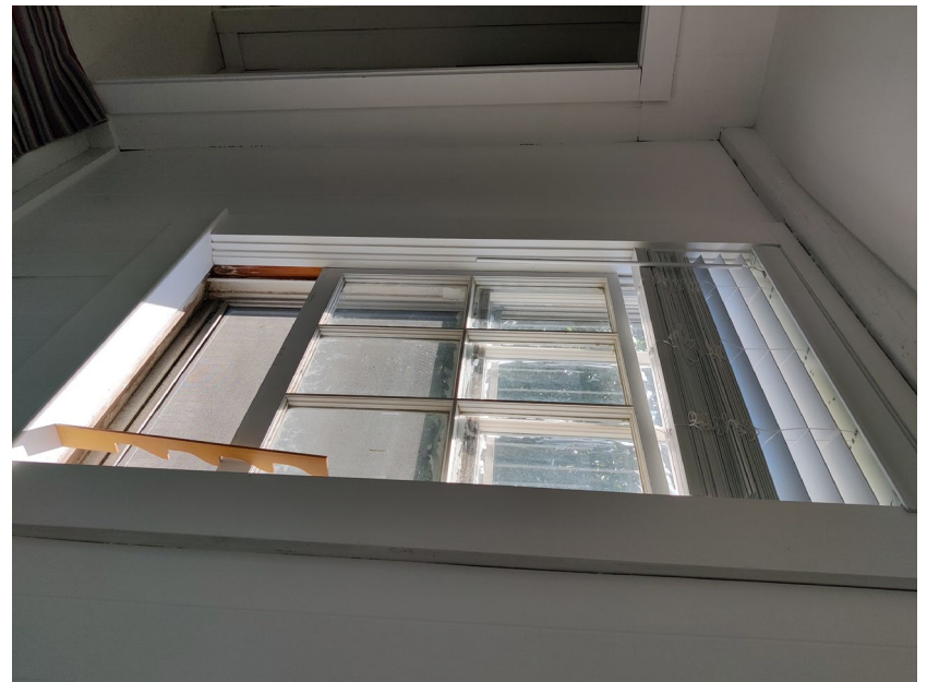
56. Second floor, stair hall window, view southwest
