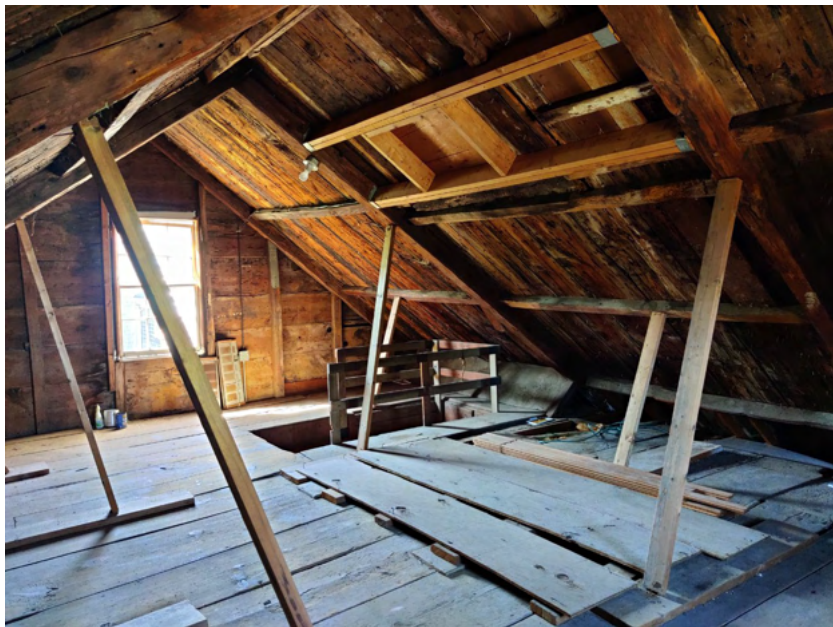
77. Attic, view northwest
