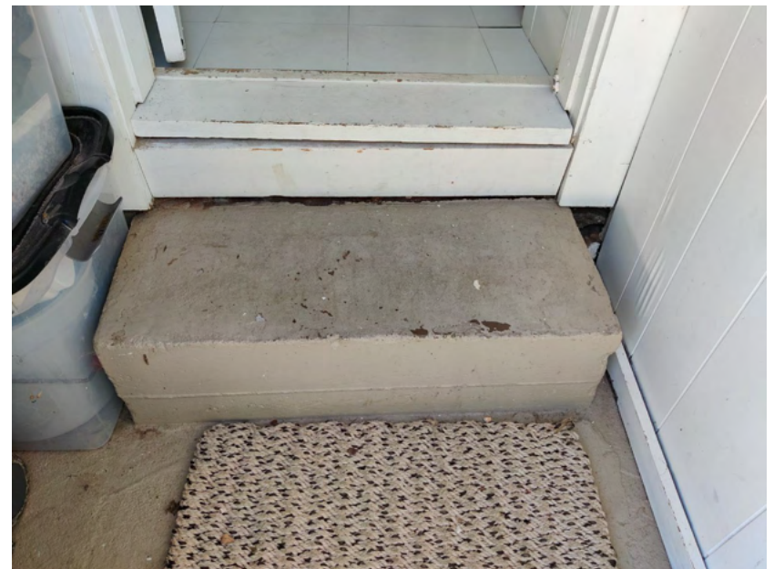
52. First floor, east entry vestibule, view west
