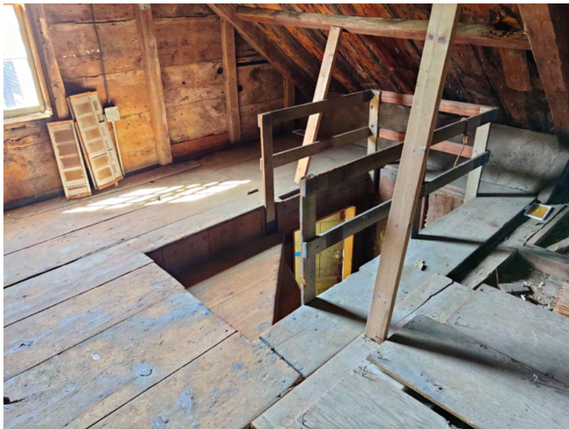
73. Attic stair, view northwest
