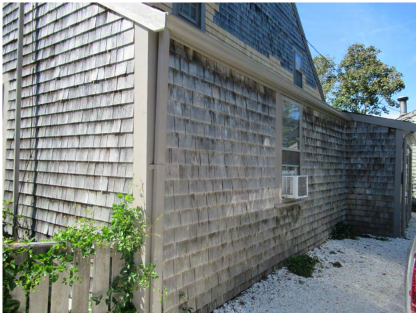
21. East elevation, south addition, view northwest
