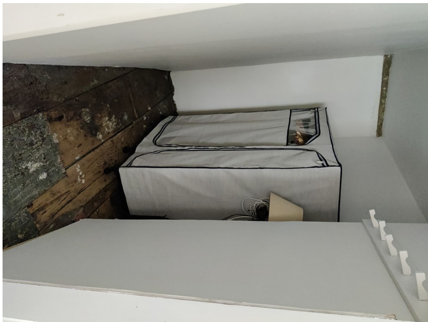
71. Second floor, closet, view east
