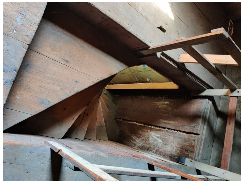
72. Attic stair, view north
