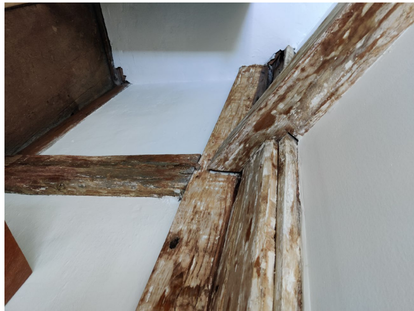
70. Second floor, northeast room, framing detail, view northwest
