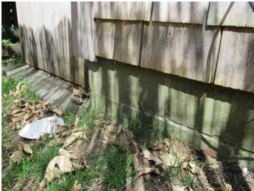
13. Cottage, foundation detail, view northeast
