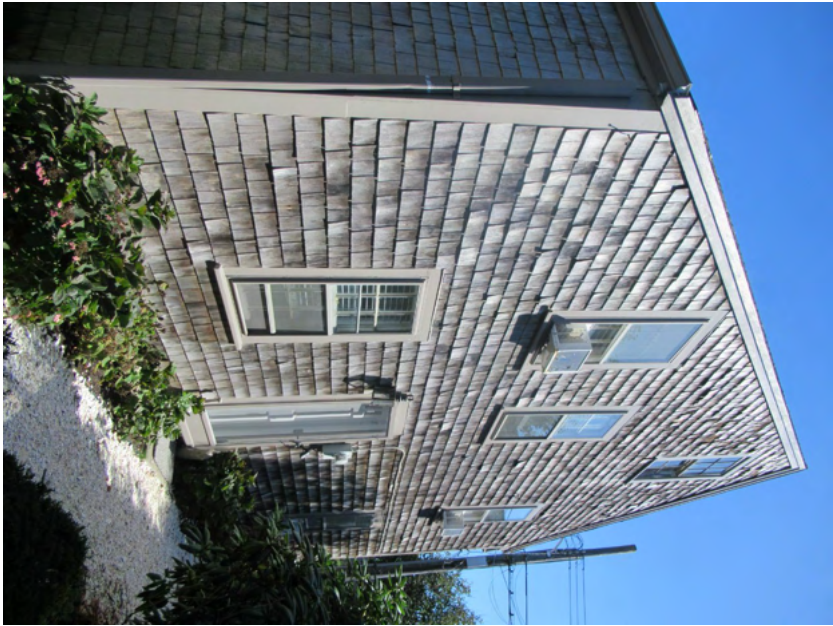
12. West elevation, view southeast
