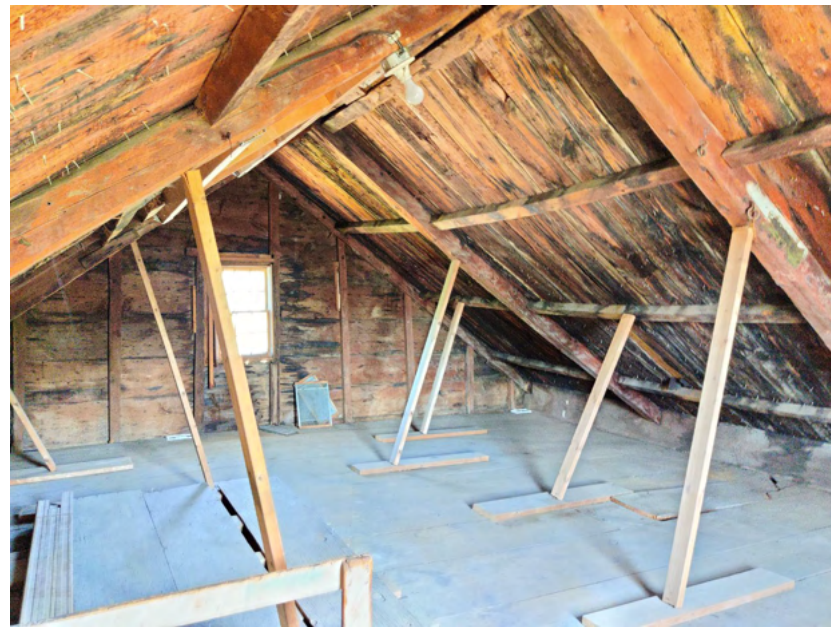
74. Attic, view southeast
