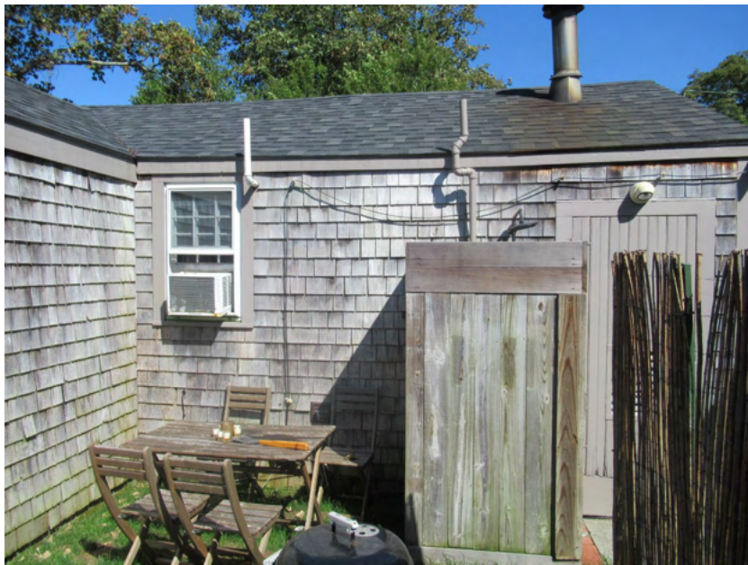
9. Cottage, west elevation, view east
