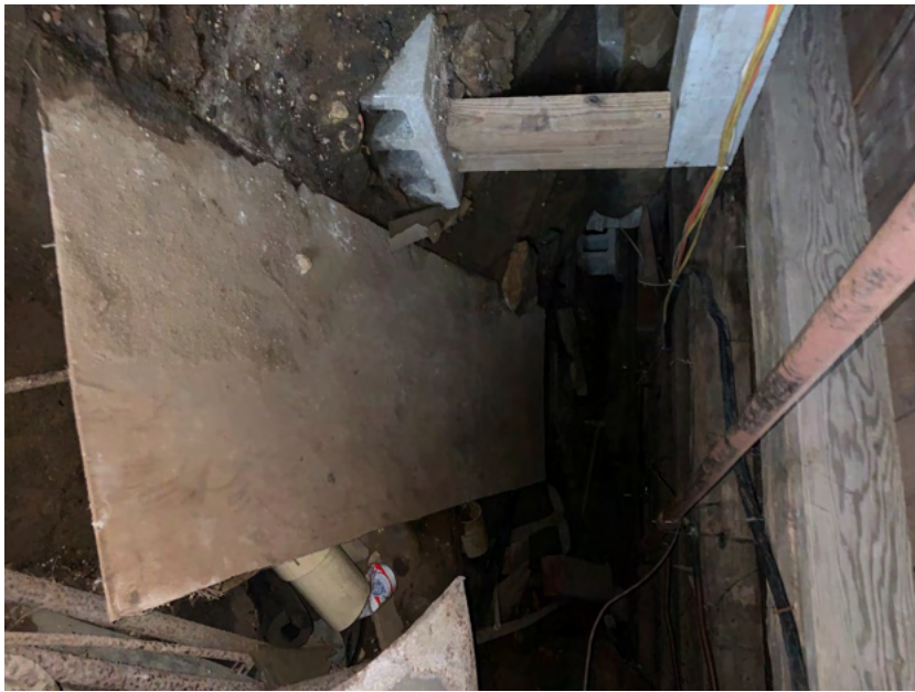
25. Crawl space, view west
