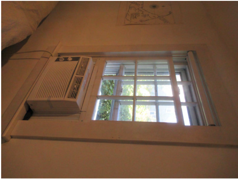
33. North bedroom, window detail, view northwest
