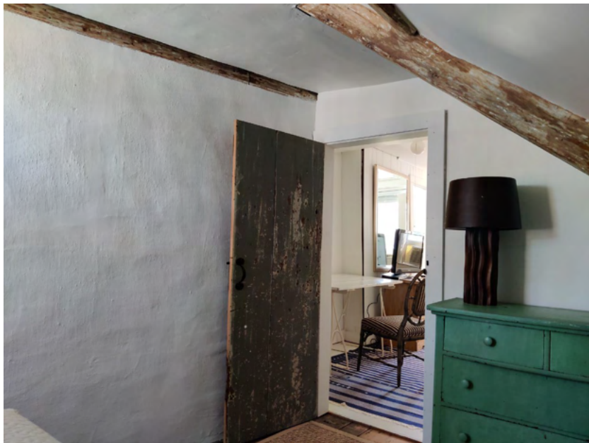
69. Second floor, northeast room, view southwest
