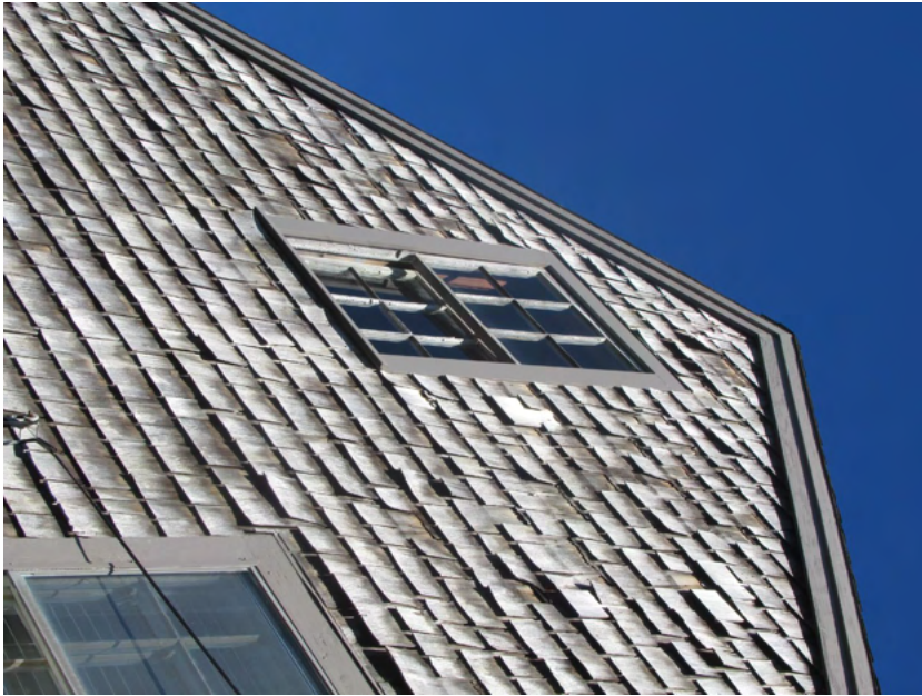
11. West elevation, attic level window, view northeast
