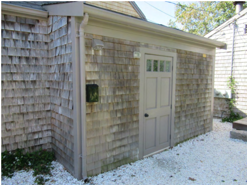
20. East elevation, north addition, view northwest
