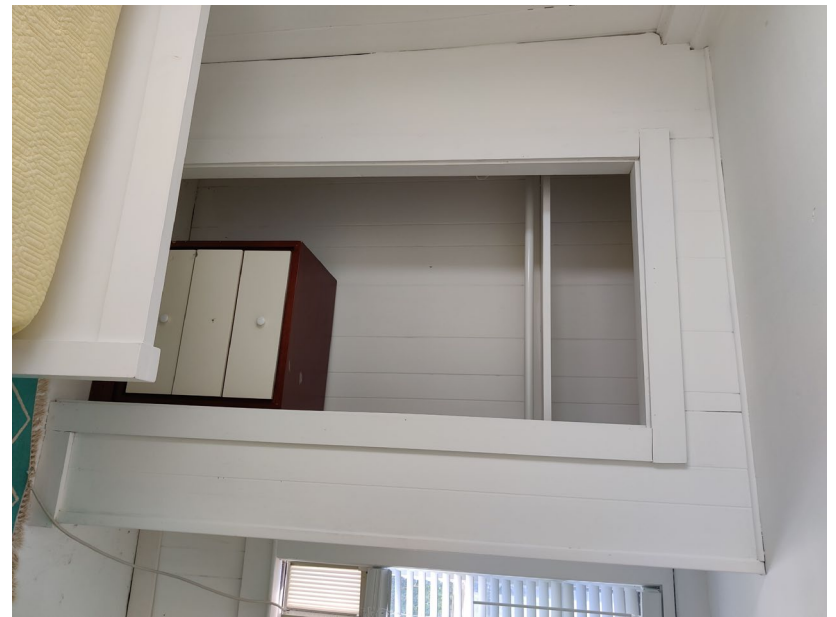
62. Second floor, southwest bedroom, non-historic closet, view southwest
