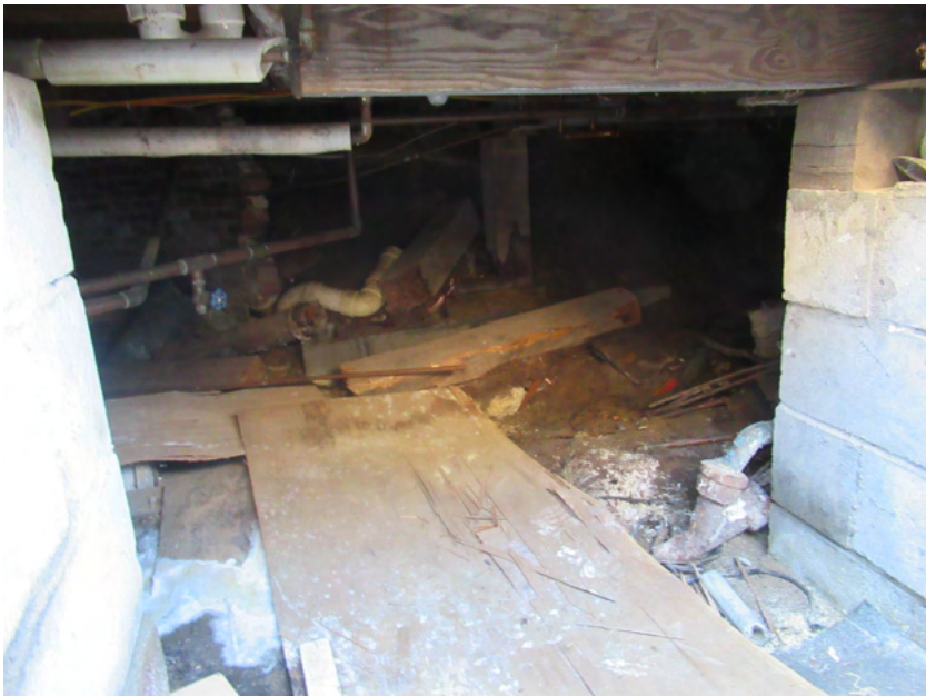
24. Crawl space, view southwest
