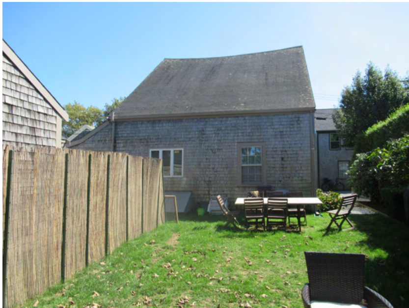
13. North elevation, view south
