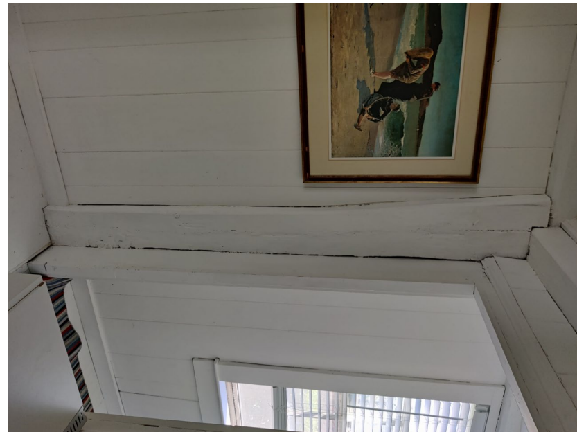
58. Second floor, hall, view northwest
