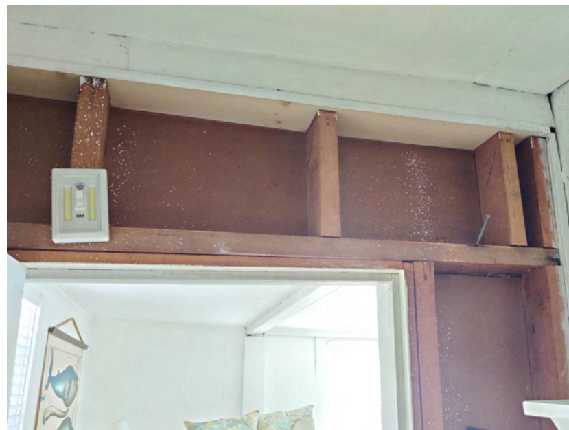
40. First floor, bedroom closet framing detail (modern construction), view south
