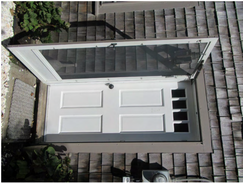
10. West elevation, main entrance, view northeast
