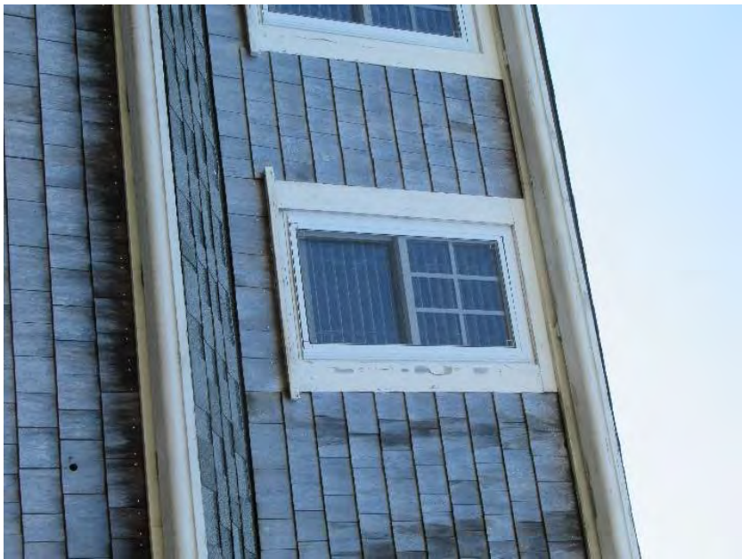
5. North elevation dormer window detail, view southeast
