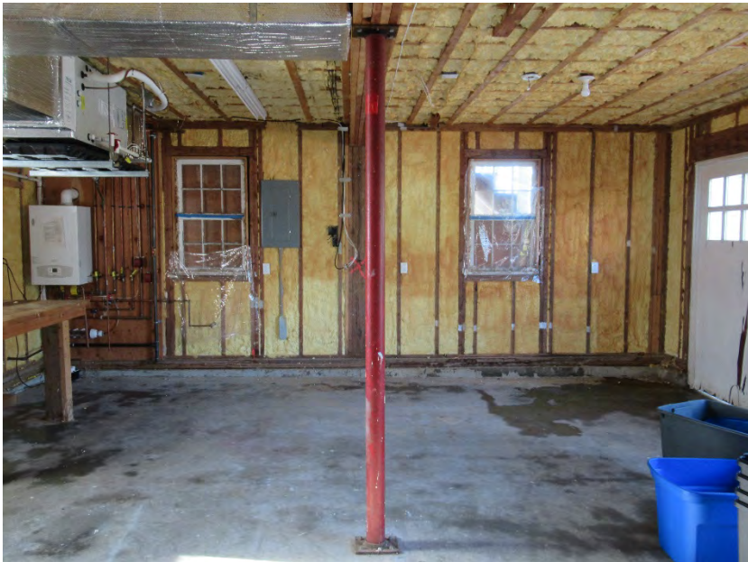
15. First floor, view west
