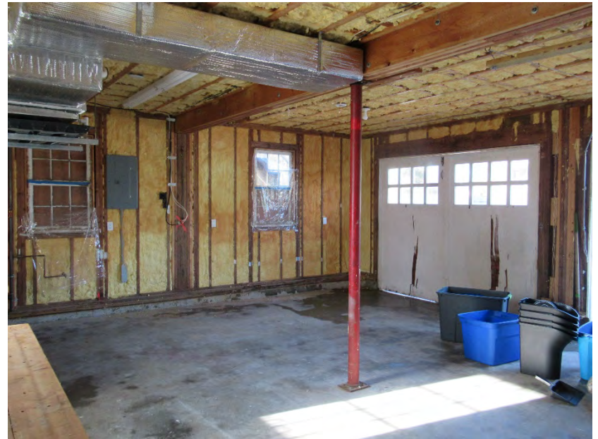
16. First floor, view northwest
