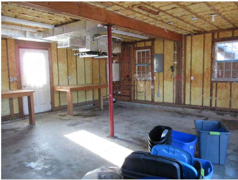
13. First floor, view southwest
