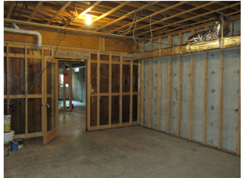
36. Basement, room under north addition, view southwest
