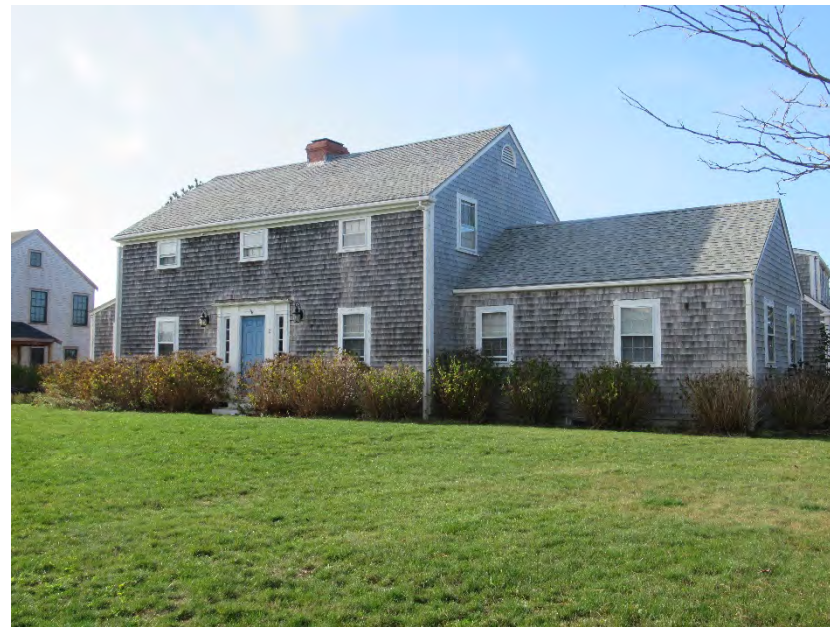
2. East elevation (left) and north elevation (right), view southwest
