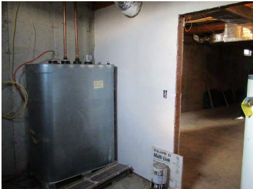
31. Basement, utility room, view northwest
