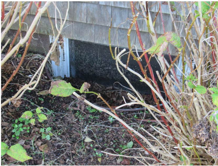
5. East elevation, typical existing window well, view southwest
