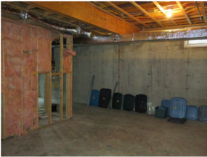
33. Basement, north room, view southwest
