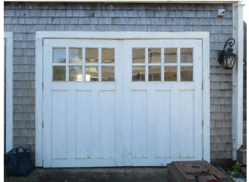
4. North elevation, garage door detail, view south
