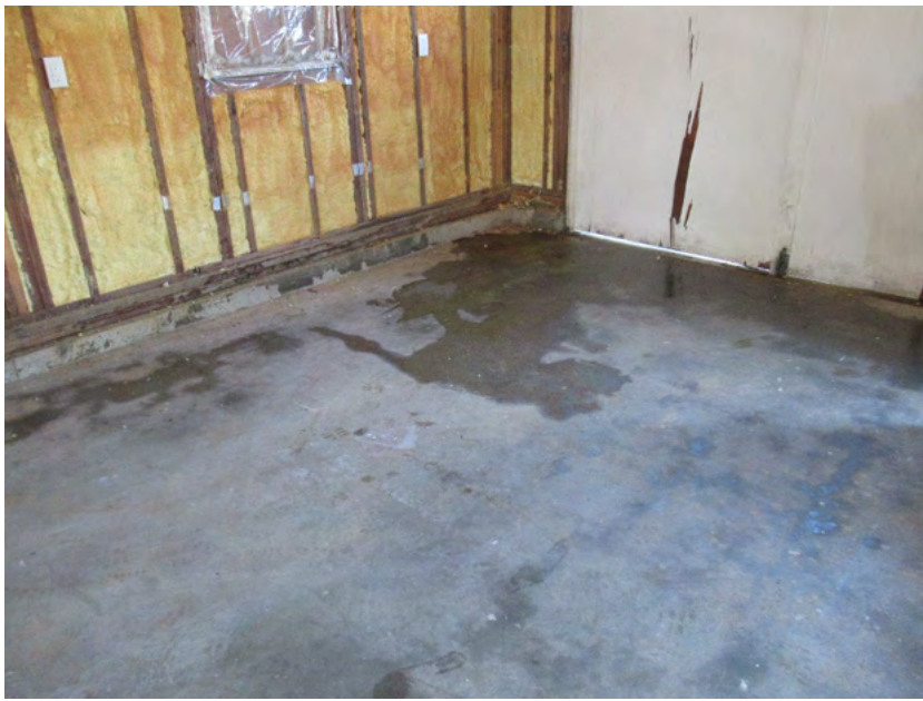
21. First floor, concrete flooring detail, view northwest
