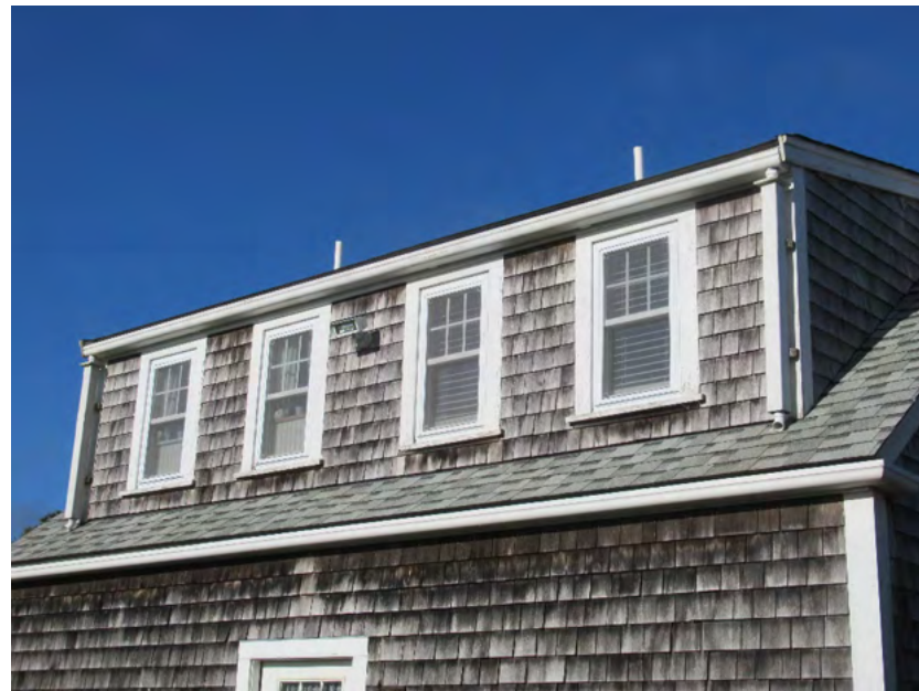
10. South elevation dormer detail, view northwest
