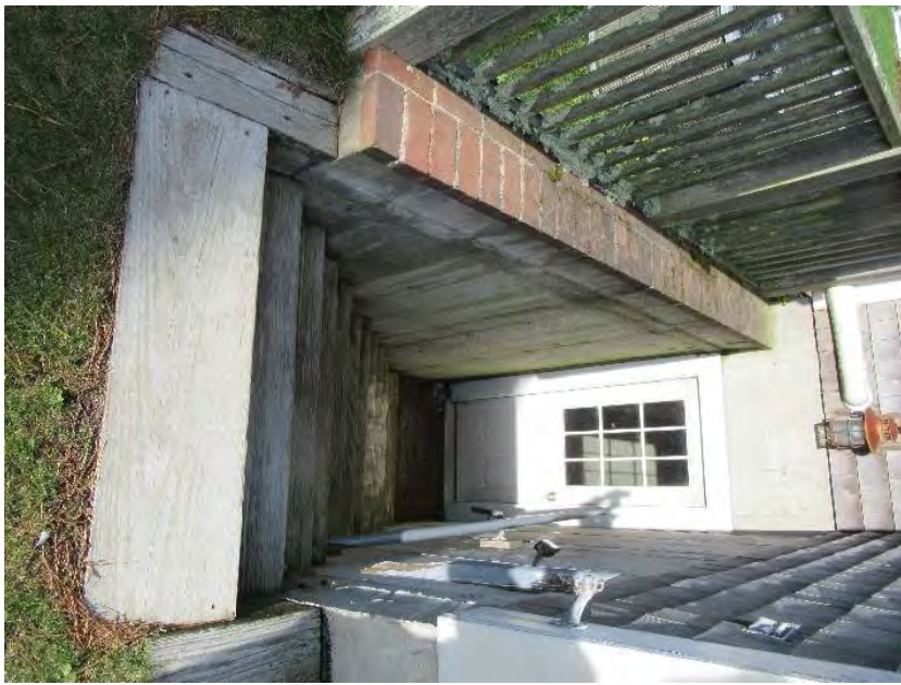
21. South elevation, basement entrance, view north
