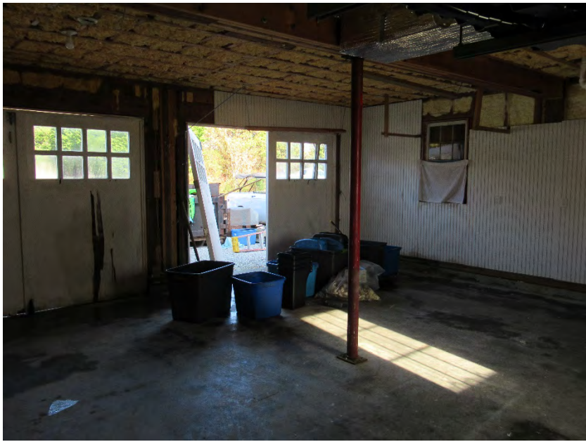
18. First floor, view northeast
