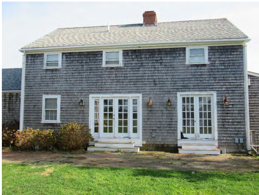
17. West elevation, main block, view east
