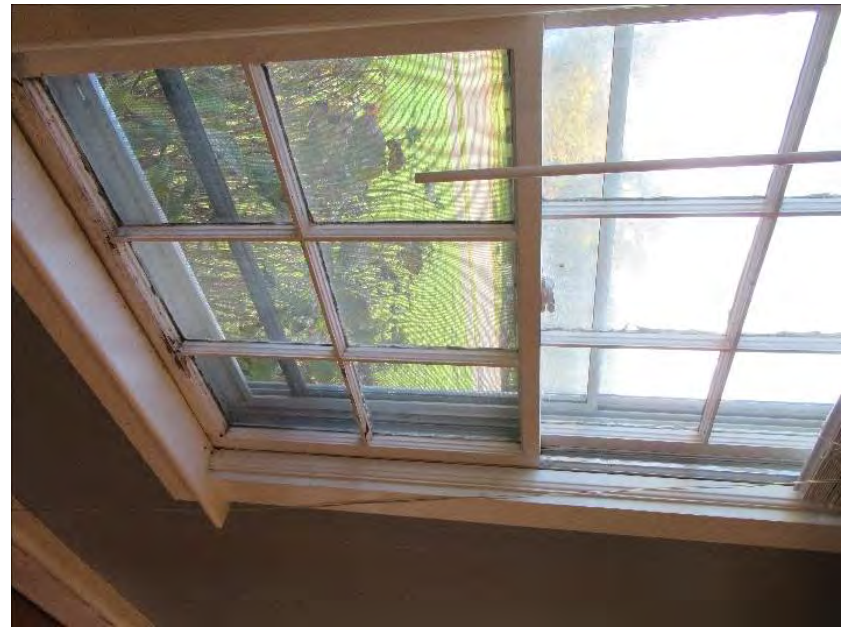
50. First floor, window detail, typical conditions, view southeast
