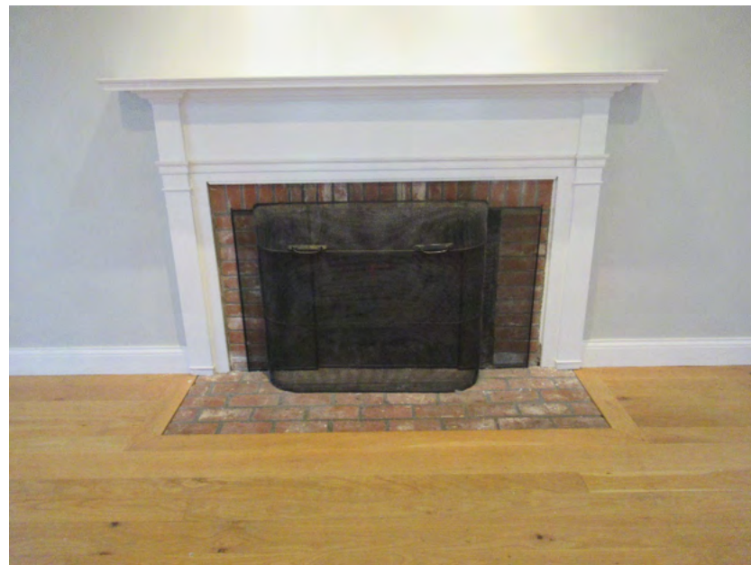
40. First floor, living room, fireplace detail, view north
