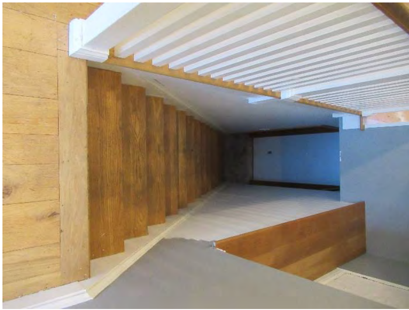
45. First floor, stair to basement, view east
