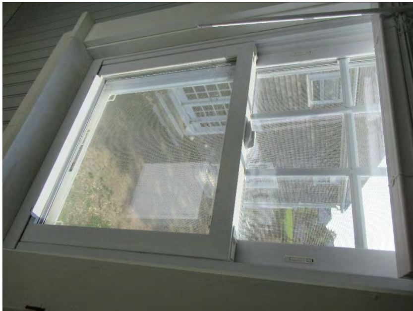
29. Second floor, bathroom, typical modern vinyl replacement window
