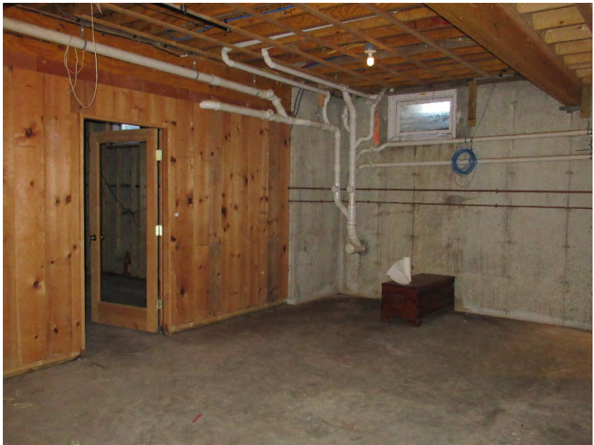
32. Basement, north room, view northeast
