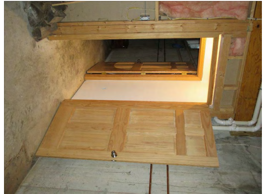
24. Basement, entrance to south room, view northeast
