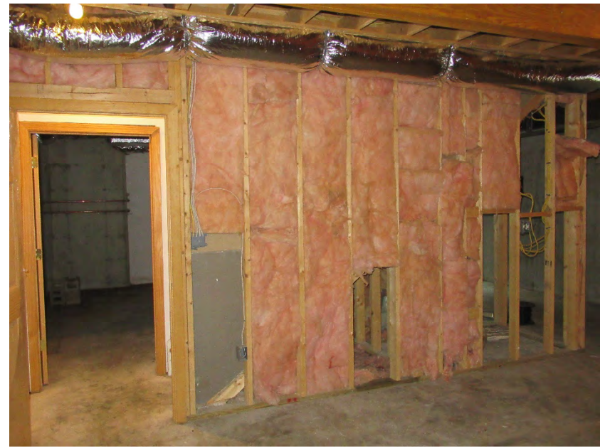
34. Basement, north room, view south
