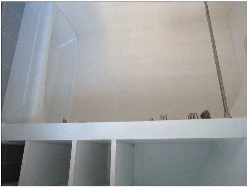
69. Second floor, west bathroom, view southeast
