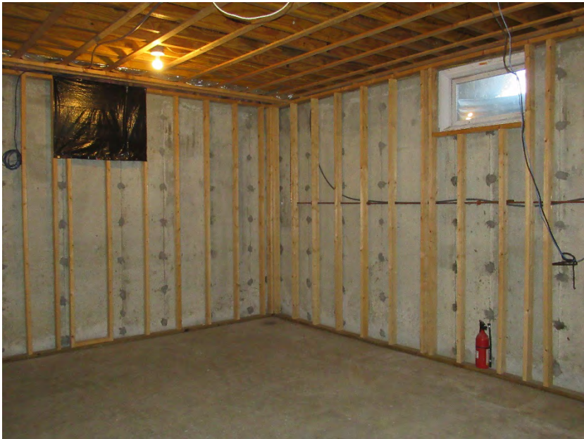
35. Basement, room under north addition, view northeast
