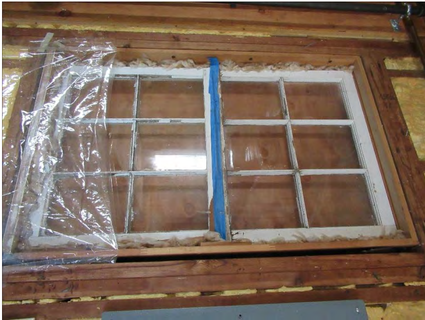
19. First floor, typical window, view southwest
