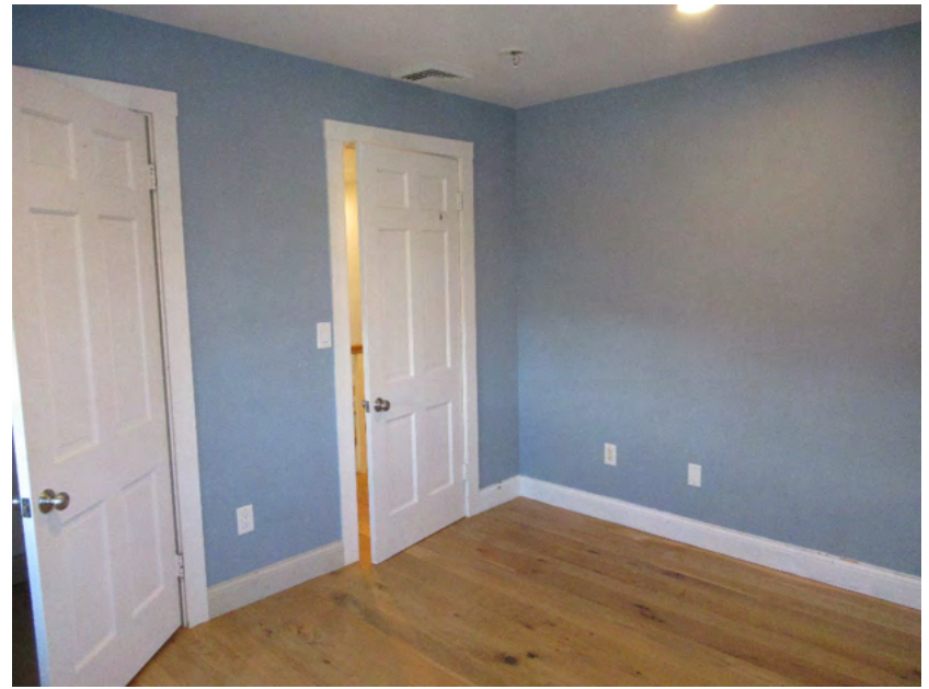
62. Second floor, northeast bedroom, view southwest
