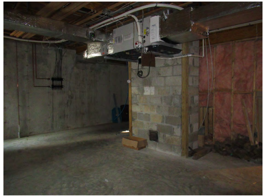
26. Basement, south room, view northwest
