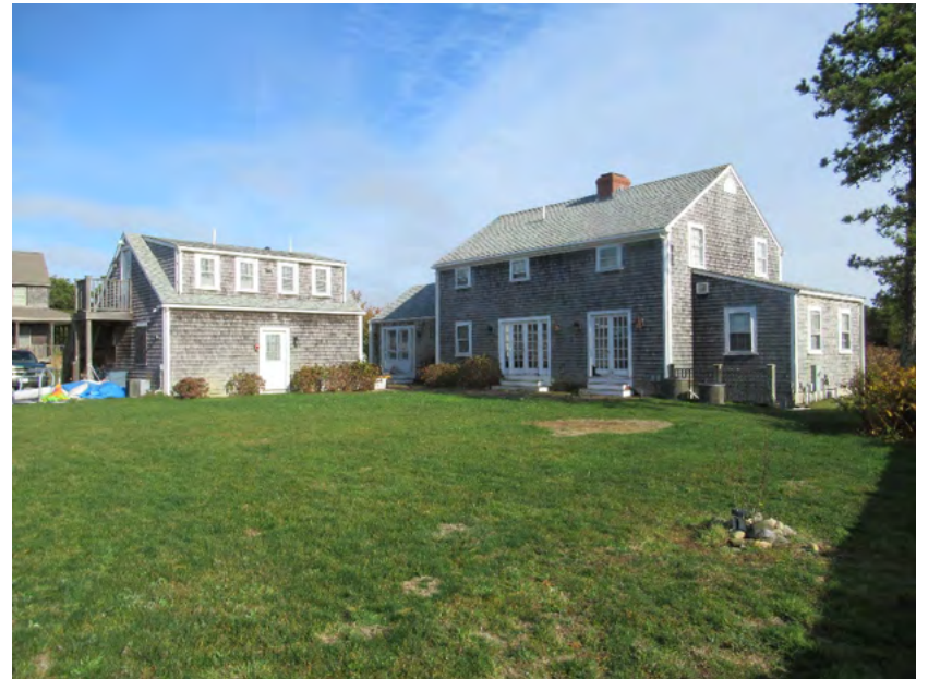
16. Garage (left) and main house (right), view northeast
