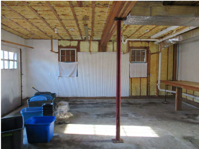
20. First floor, view east
