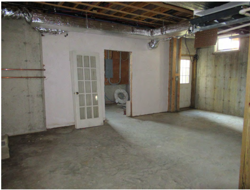
25. Basement, south room, view southwest
