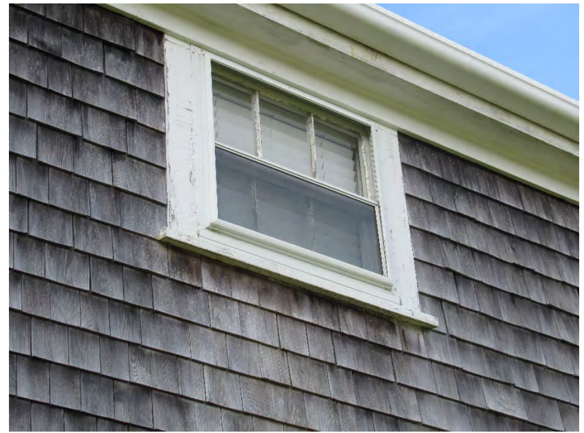
6. East elevation, typical upper floor window, view northwest
