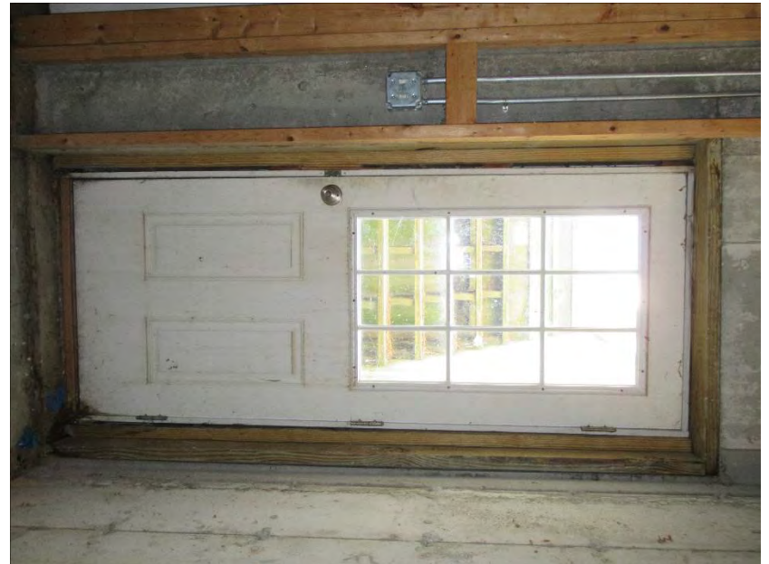
28. Basement, exterior door, view south
