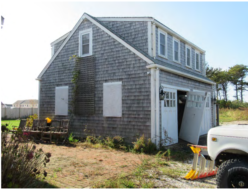
1. East elevation (left) and north elevation (right), view southwest
