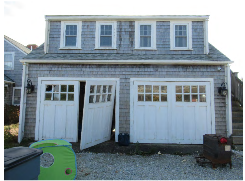
2. North elevation, view south
