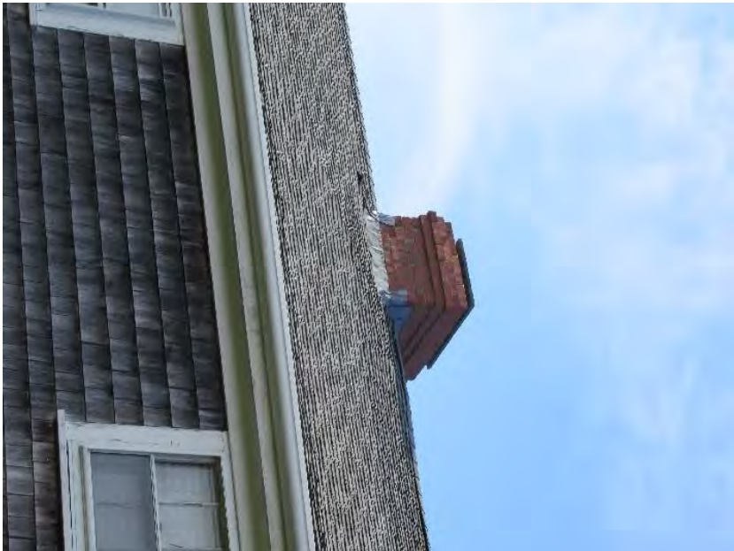
7. Chimney at main block, view southwest
