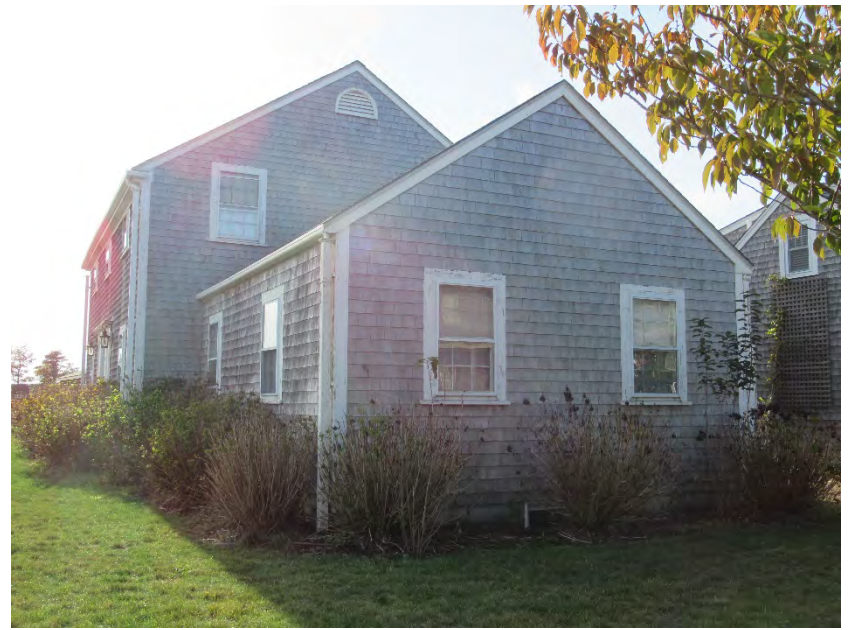
10. North elevation, view south
