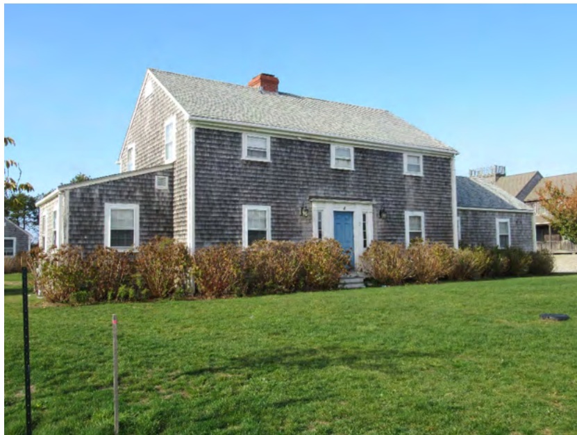
1. South elevation (left) and east elevation (right), view northwest
