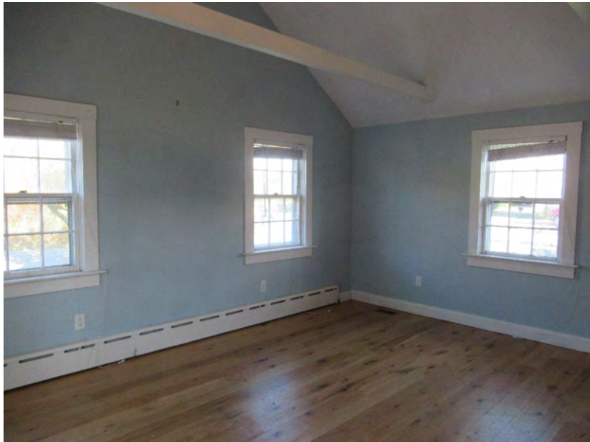
55. First floor, north addition, view northeast
