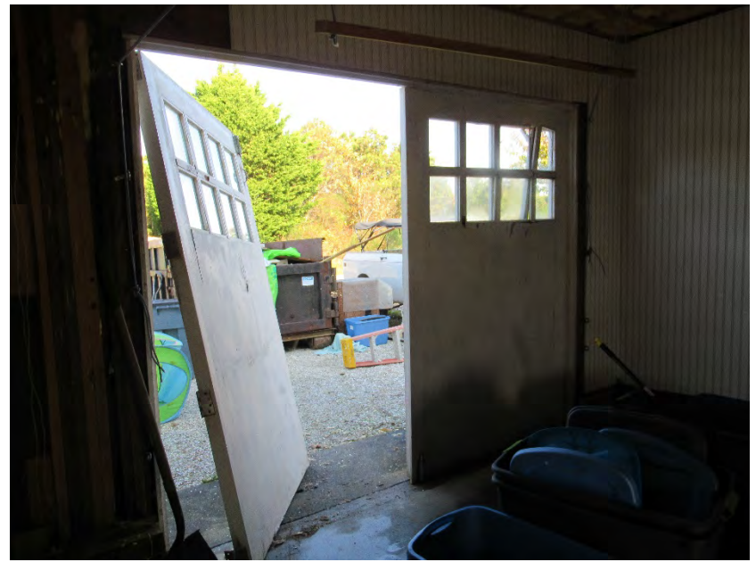
14. First floor, garage door detail, view northeast
