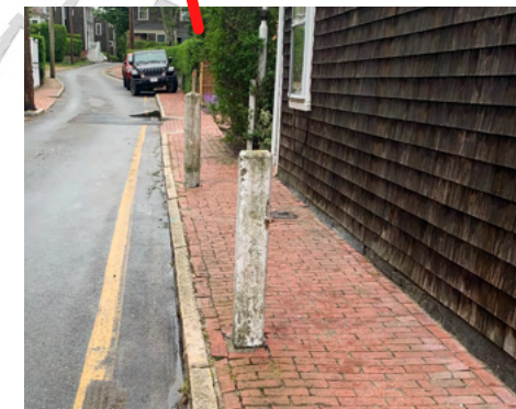
Concrete bollards to remain
