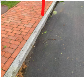
Example of New Sidewalk
