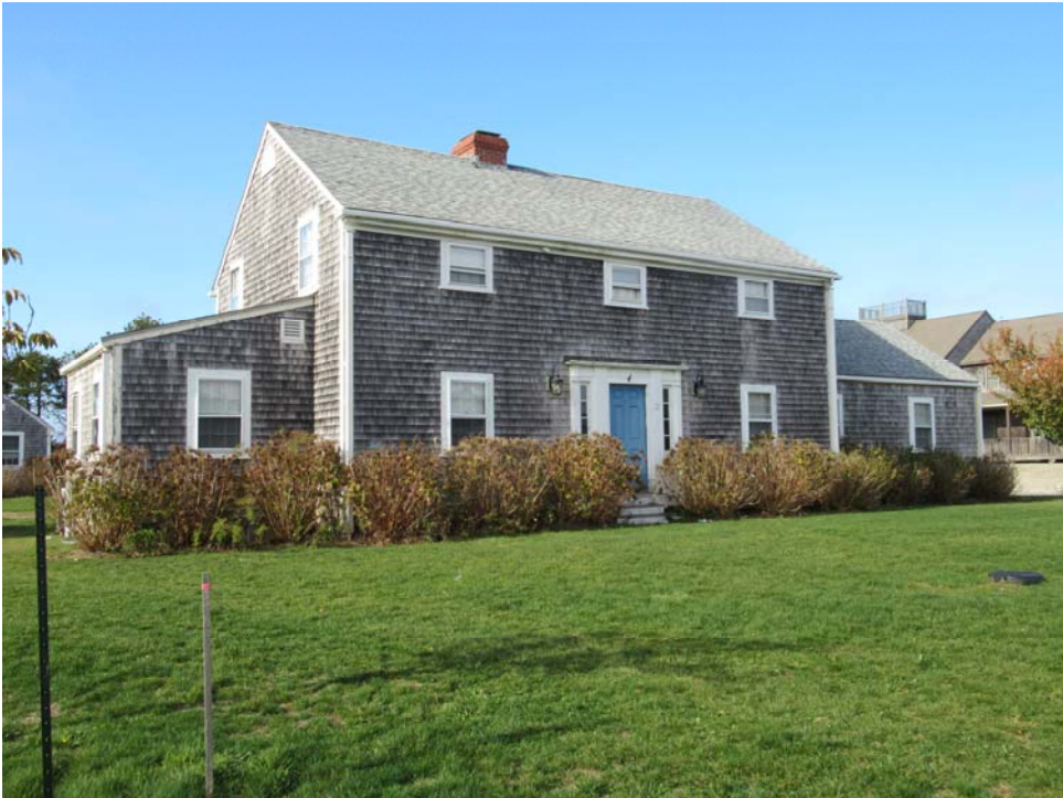
1. 2 Mayflower Circle, main house, view northwest
