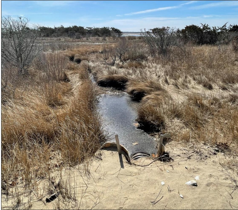
Figure 45. Existing corrugated plastic pipe under road.
