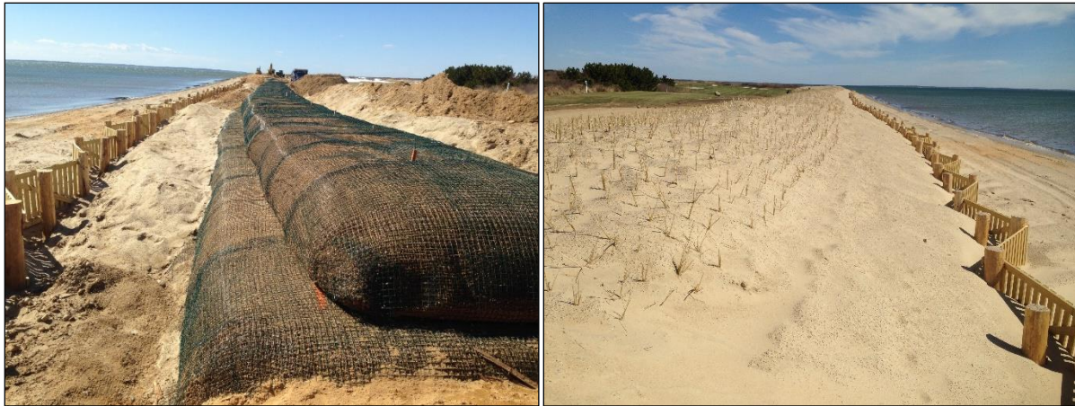
Figure 82. Example of a coir project on Cape Cod, located in NHESP habitat.
