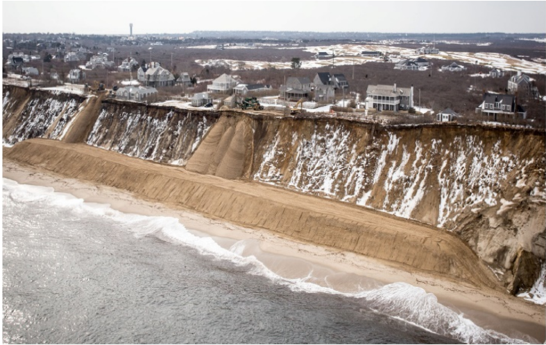
Source: Baxter Road and Sconset Bluff Stabilization Project, Nantucket, MA, EEA No. 15240 Available HERE
