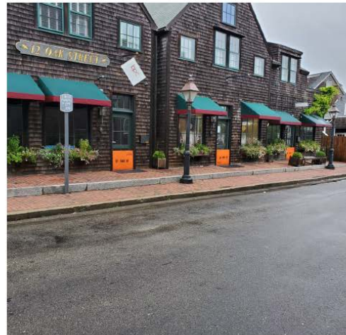
Deployable Flood Barriers on Oak Street (Image: Vincent Murphy)
